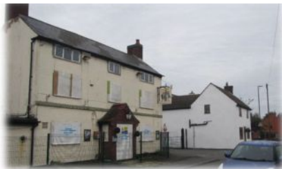
Front elevation of the Oddfellows Arms taken from Main Street
