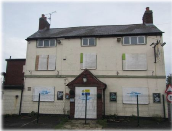
Front elevation of the Oddfellows Arms taken from Main Street
