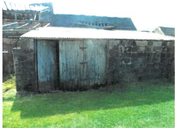
Photo 2: Second cinder structure adjoined to barn along northern elevation.
