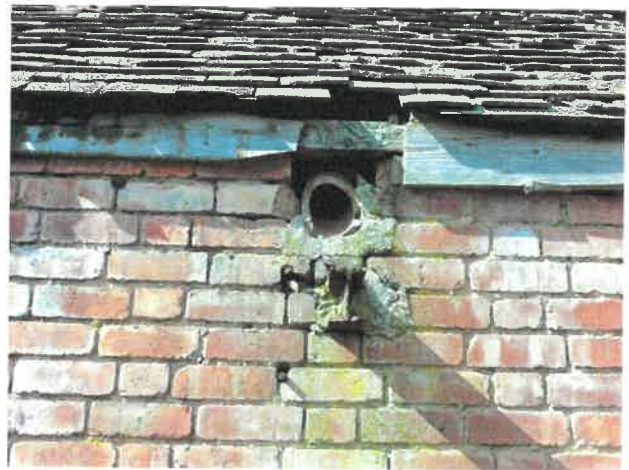
Photo 6: Ventilation pipes in walls of stable 1 from eastern elevation.
