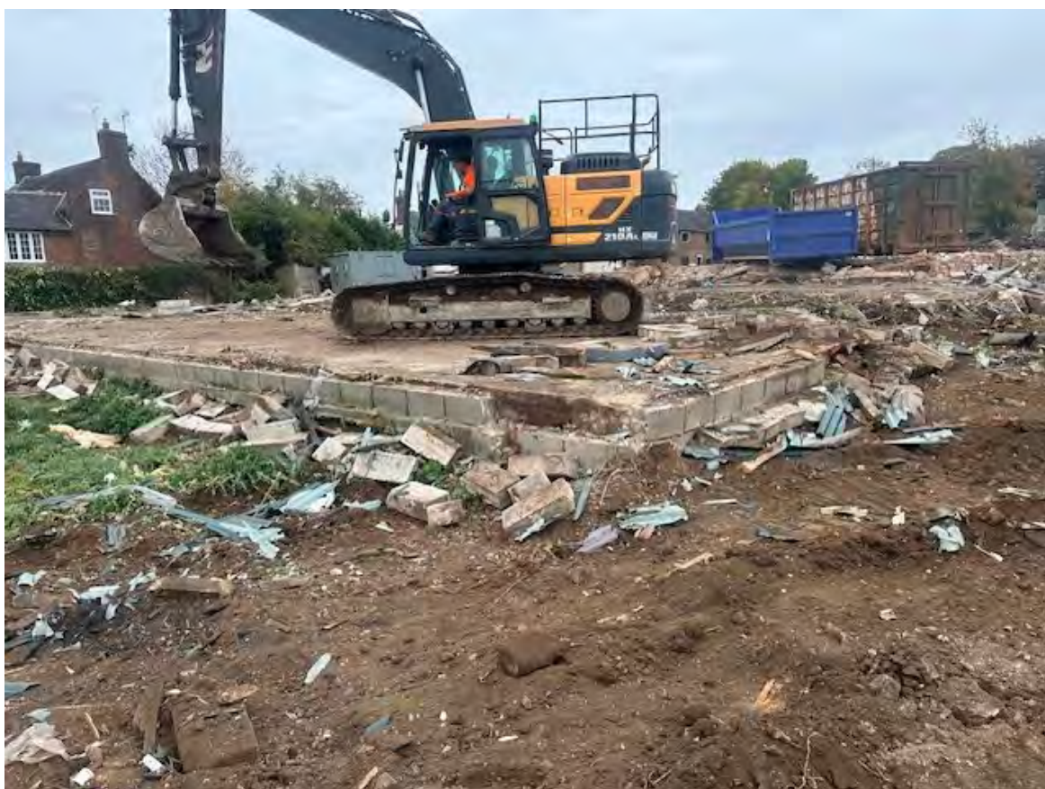
Plate 2: Example of raised concrete raft
