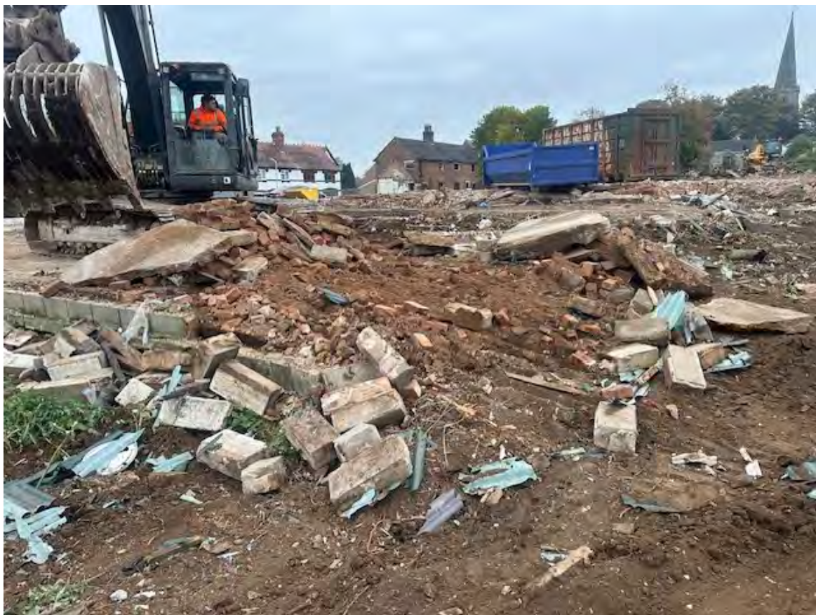
Plate 3: Rubble exposed below raft
