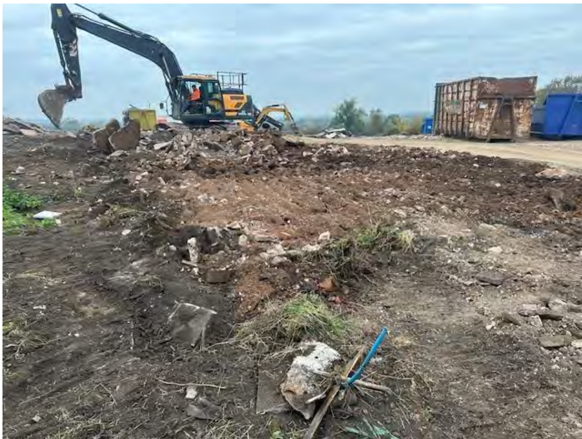
Plate 4: Extent of demolition work
