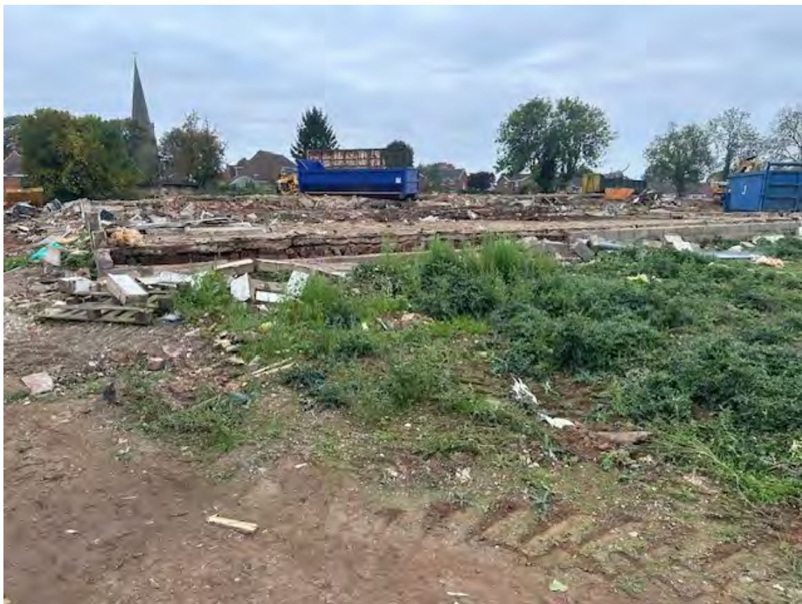
Plate 1: Looking south across site
