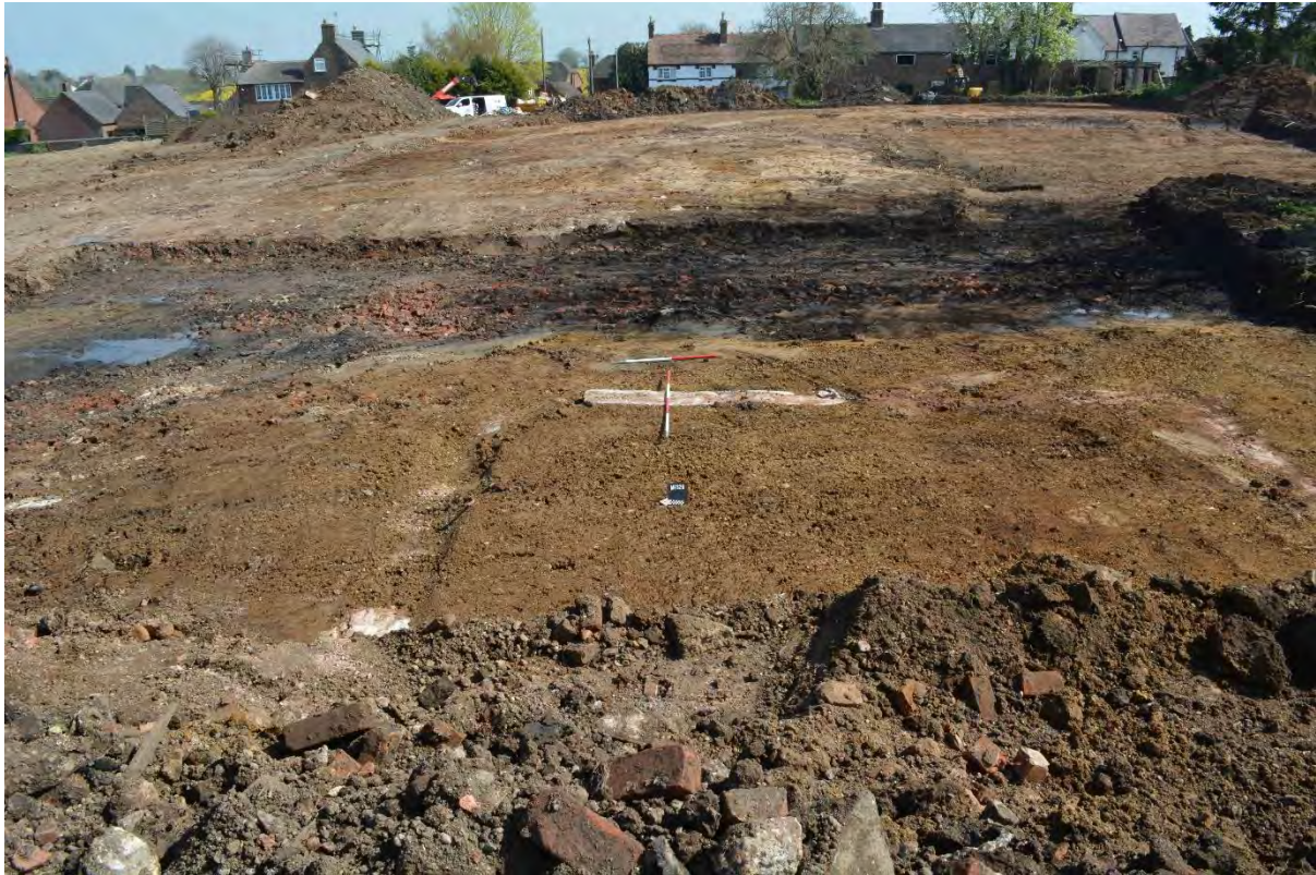
Plate 5: view across stripped area looking east
