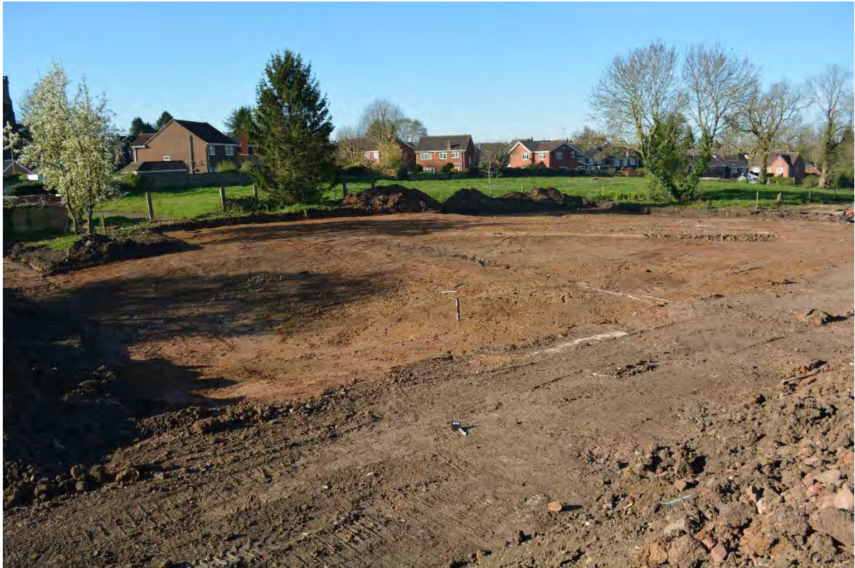
Plate 1: View across stripped area looking south-south-west
