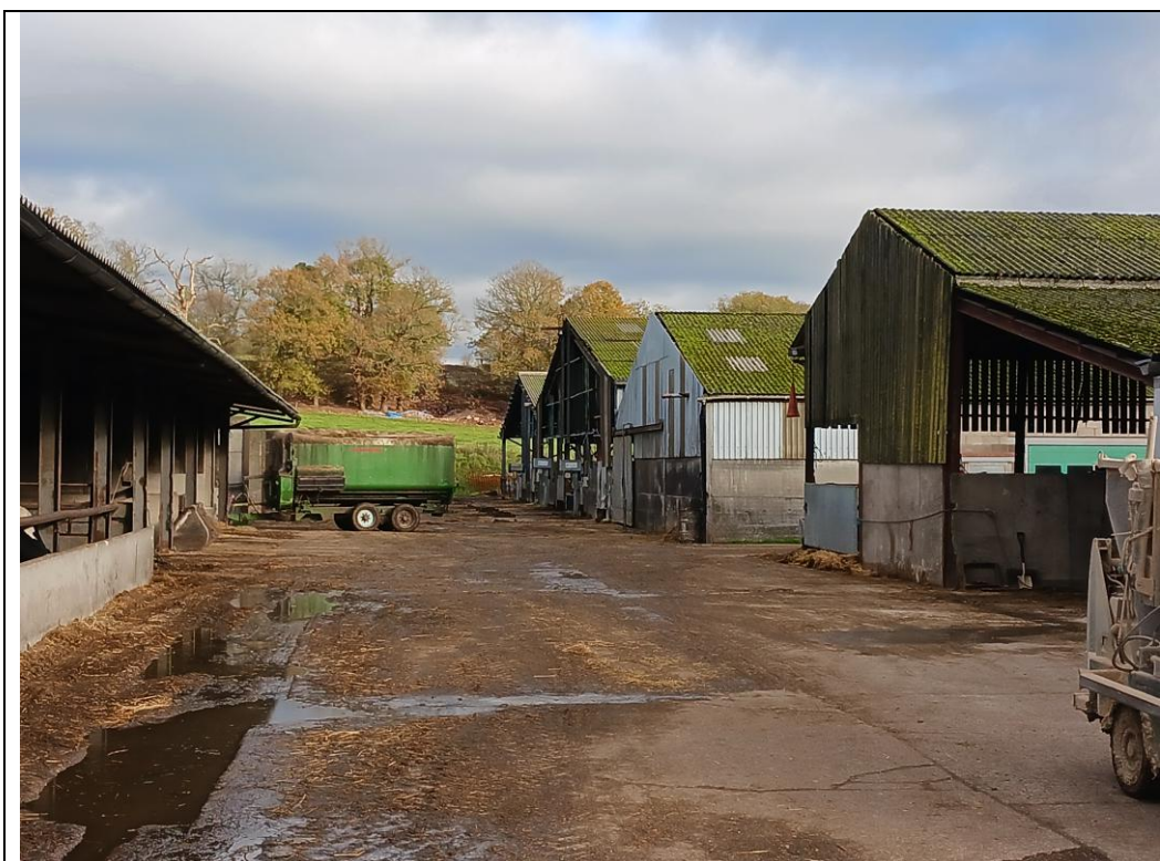
Plate 5: The adjacent farm building of Groby Park Farm which comprise modern steel framed buildings set in a concrete yard.
