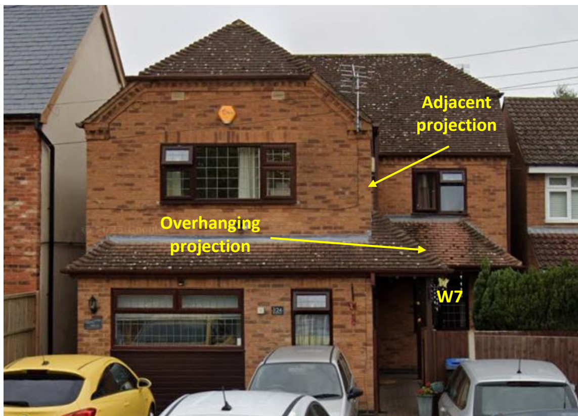
Figure 6: Two Hoots front elevation, annotated with the location of window ref. W7 and highlighting inherent design constraints concerned
