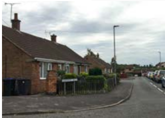
Existing dwellings on Station Road
