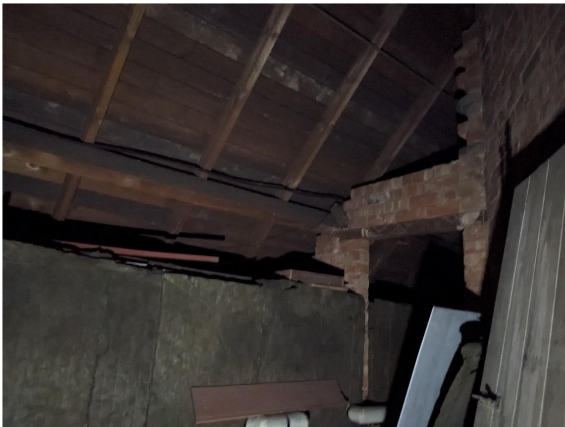
Plate 16 – Internal loft space, southern aspect of the main section.
