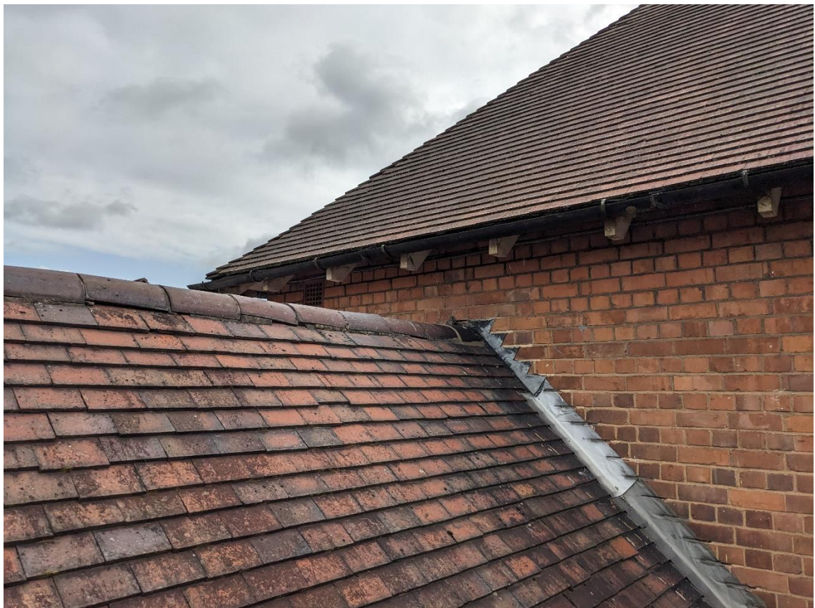
Plate 8 – Close up of eaves and ridge tiles.
