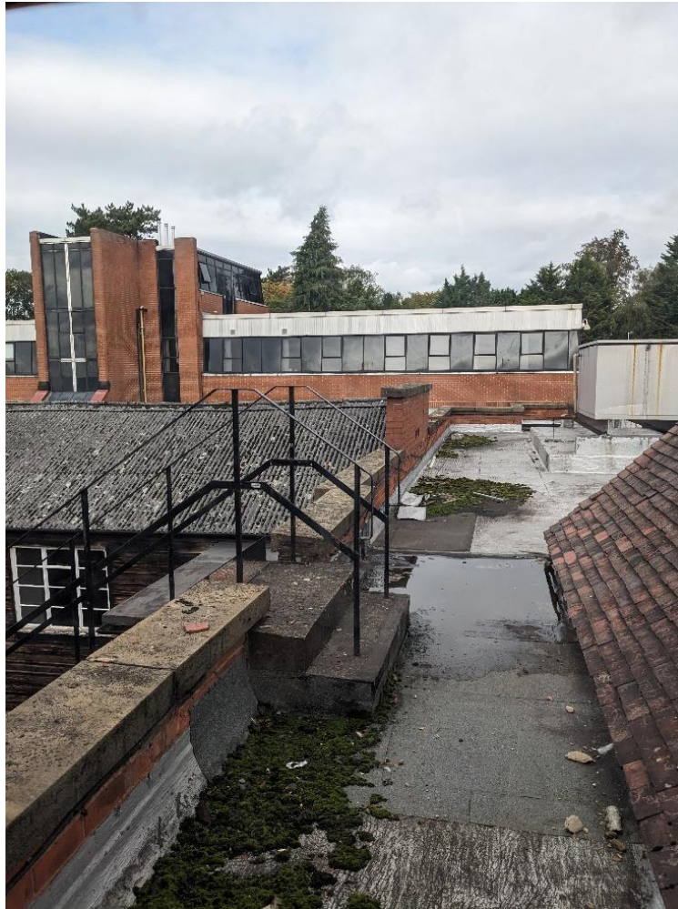
Plate 7 – Rooftop of main building.
