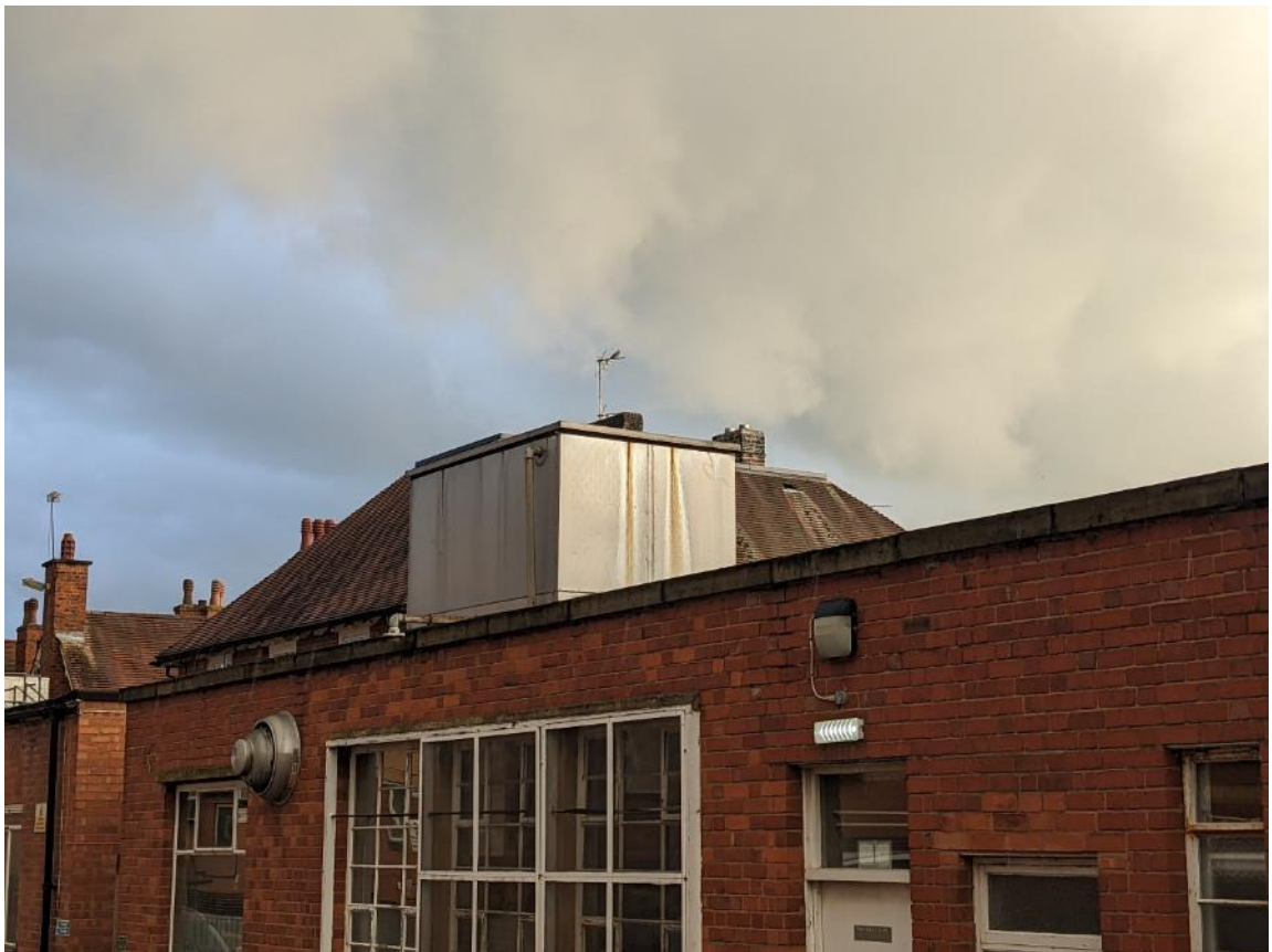
Plate 4 – eastern aspect roof.
