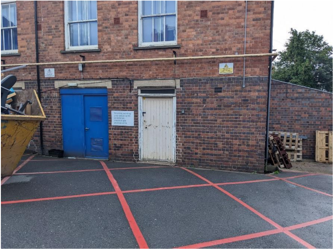
Plate 1 – General view of the northern aspect.
