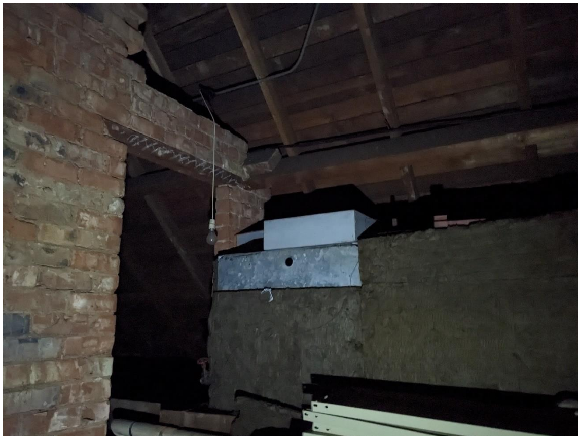
Plate 17 – Eastern aspect of the main internal loft space.
