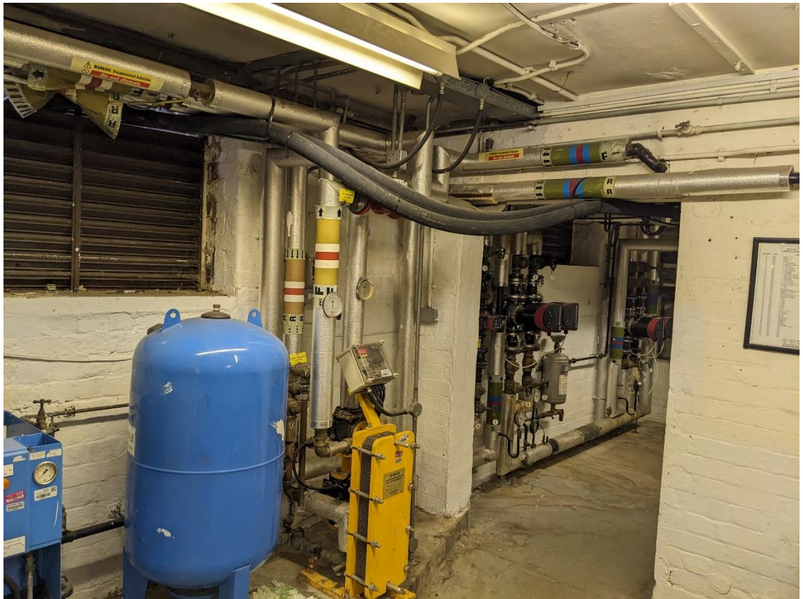
Plate 11 – Internals of basement areas.
