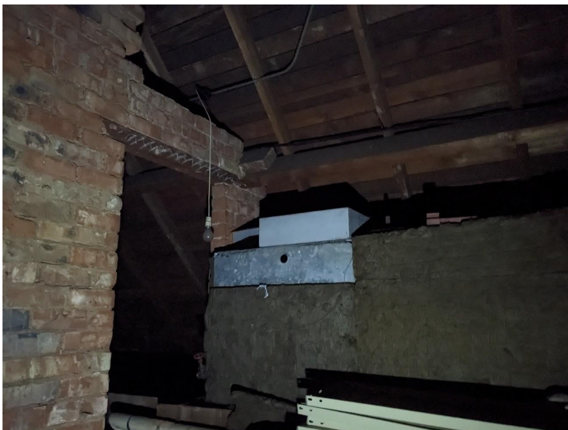
Plate 18 – Ceiling of the main internal loft space.
