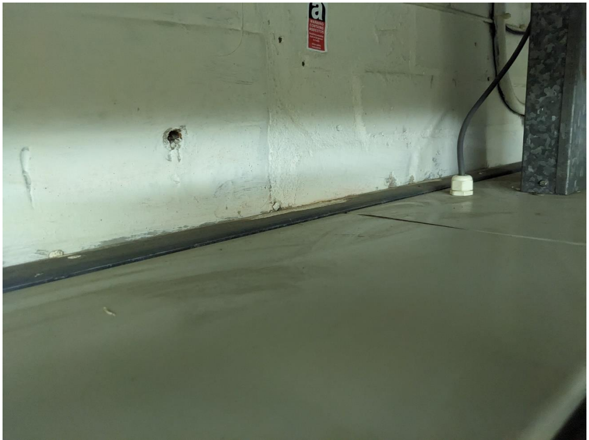
Plate 12 – Example of cabinet tops in basement area with no guano present.
