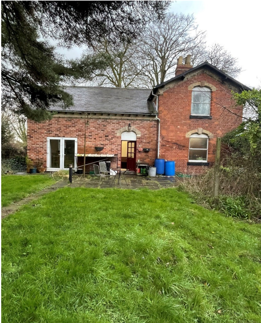
EXISTING REAR ELEVATION OF THE PROPERTY
