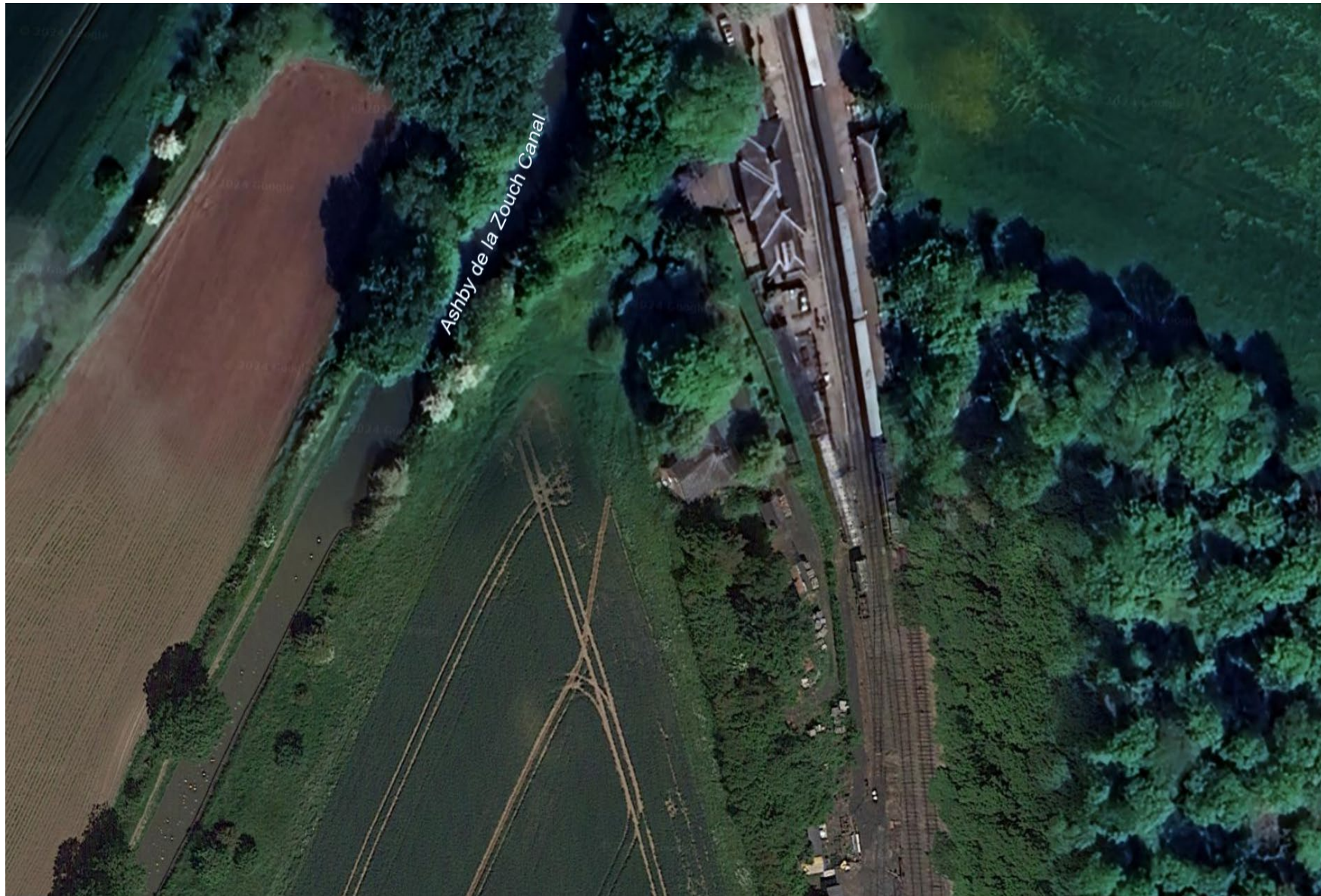
PHOTOGRAPH OVERVIEW OF STATION HOUSE AND THE ADJACENT STATION
