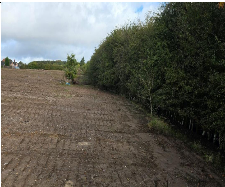
Plate 3: Image showing the site clearance and retained line of trees.
