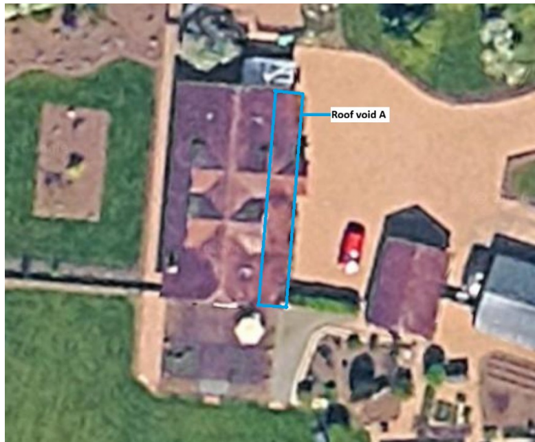
Figure 4: Roof void A within building B1.
