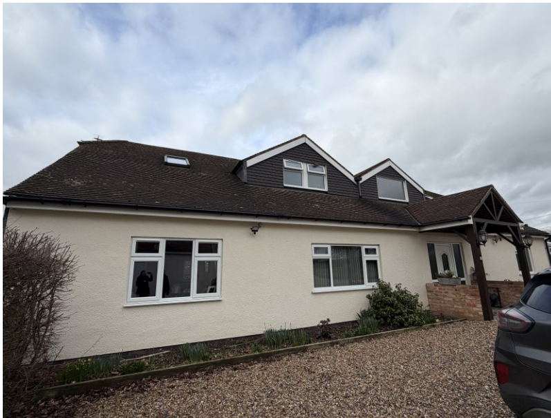
Figure 3: The existing residential building that will be extended and modernised within the proposed development.
