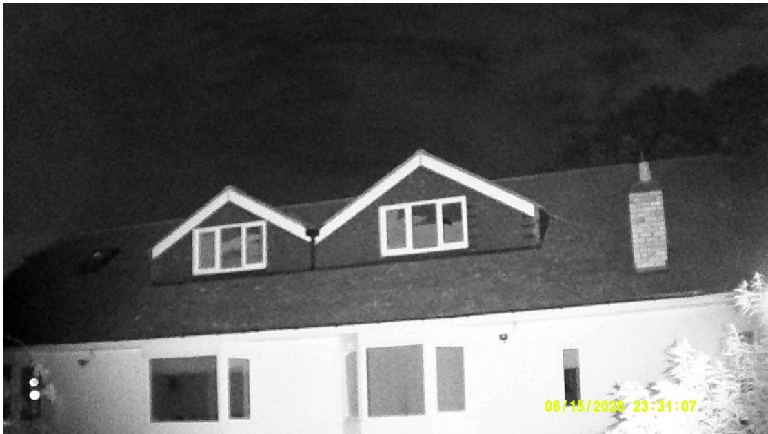
Figure 8 Western Elevation of B1 15 June 2026
