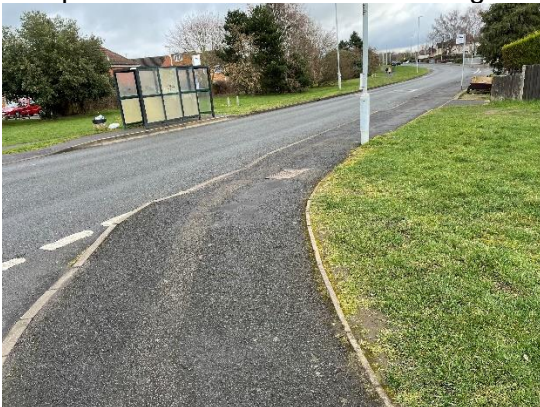
The photo above shows the existing dropped kerb and the existing lamp post.
