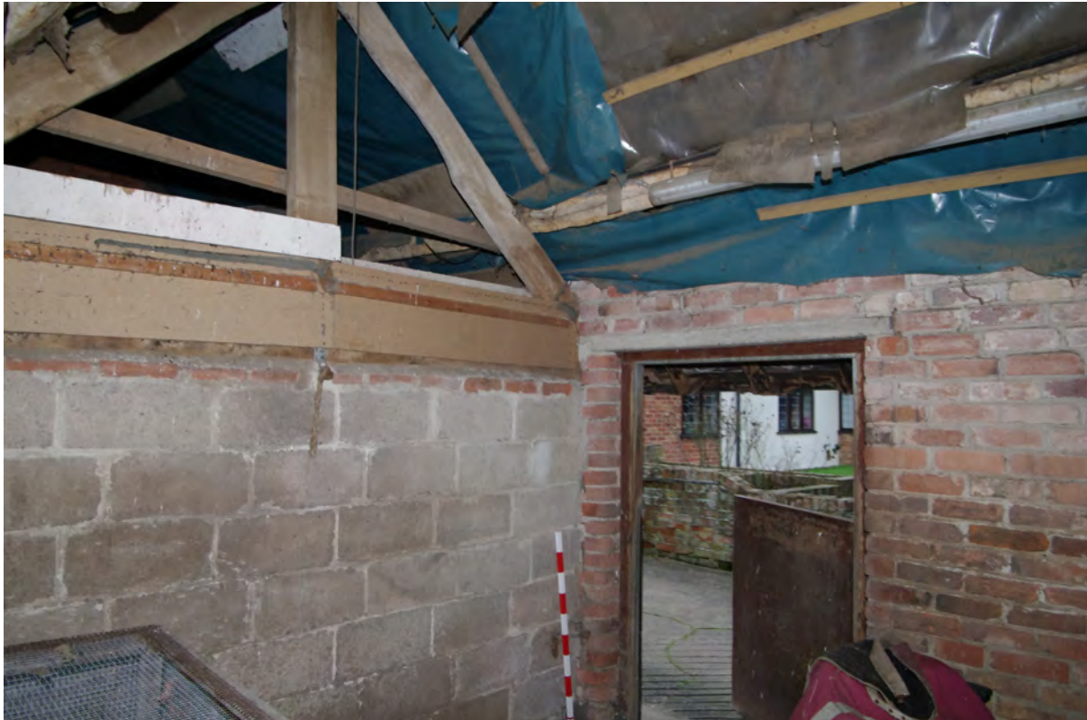
Figure 49: North-eastern stable, dividing wall and roof structure Looking east. 1m scale
