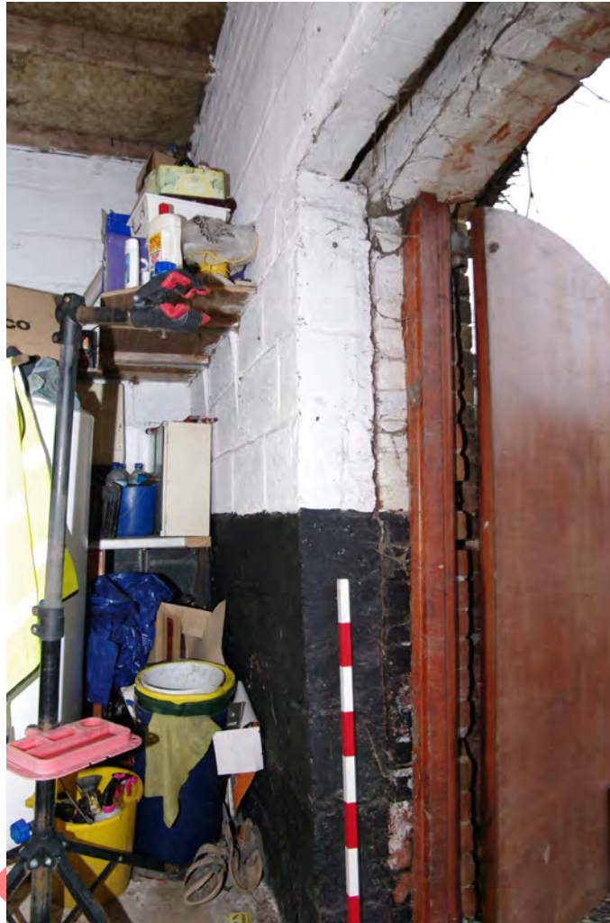
Figure 37: Threshing barn ground floor east end room
