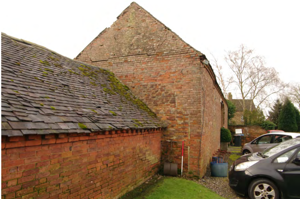
Figure 31: Threshing barn. North-east facing elevation
