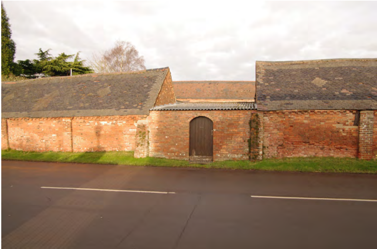
Figure 17: Area of roof to be raised between the barns on Main Street Looking north-west
