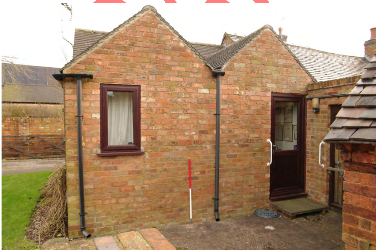
Figure 53: South-west facing elevation of the office annex Looking north-east. 1m scale
