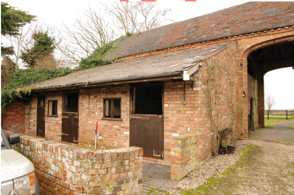
Figure 38: Stable built against the south-east facing elevation of the threshing barn Looking north-west. 1m scale
