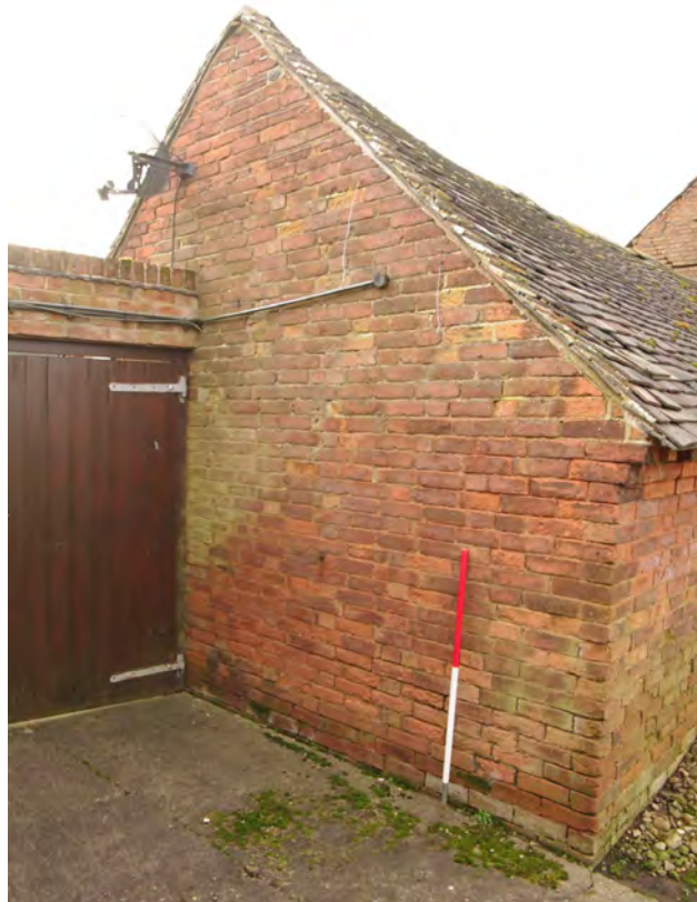
Figure 47: North-eastern stable, north-east facing gable end Looking south-west. 1m scale. The wall and gateway on the left joins the front of the office extension
