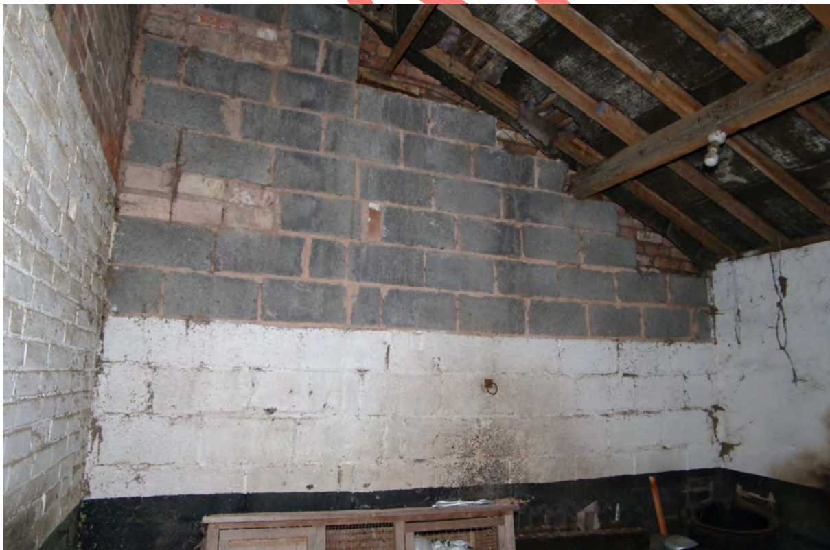
Figure 44: South-western stable, reinforced eastern end wall Looking north-east at the inserted skin of modern blockwork
