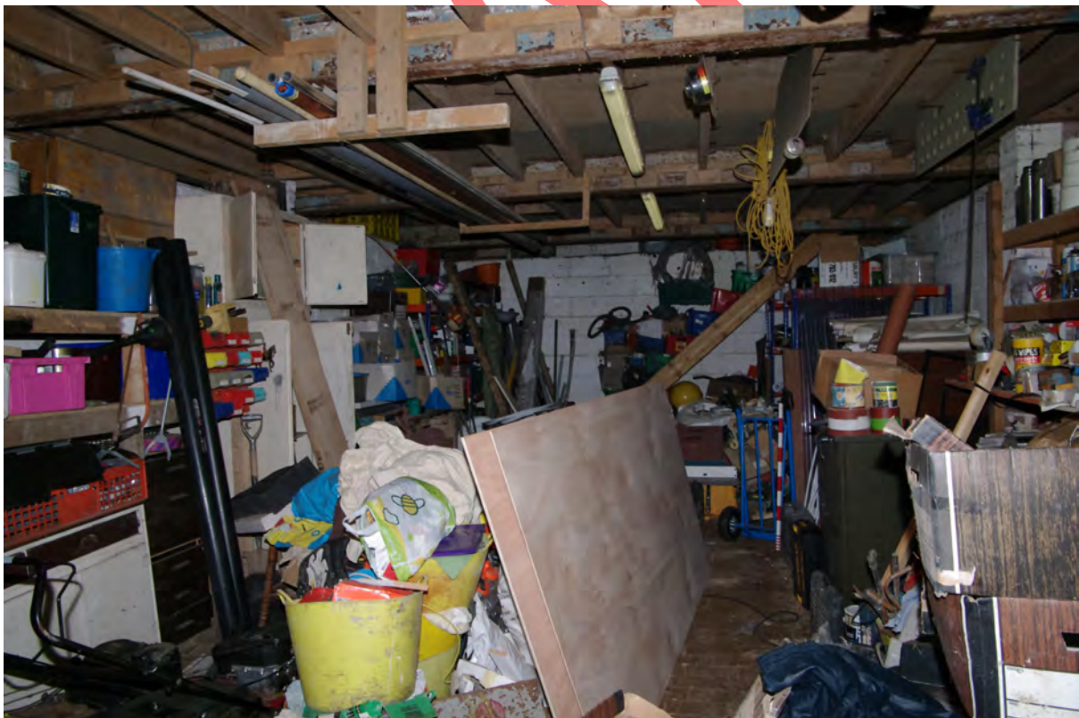
Figure 34: Threshing barn ground floor Looking south-west in the western room. Note the breeze block-lined wall at the end and sides of the room and the modern RSJ girders forming the ceiling
