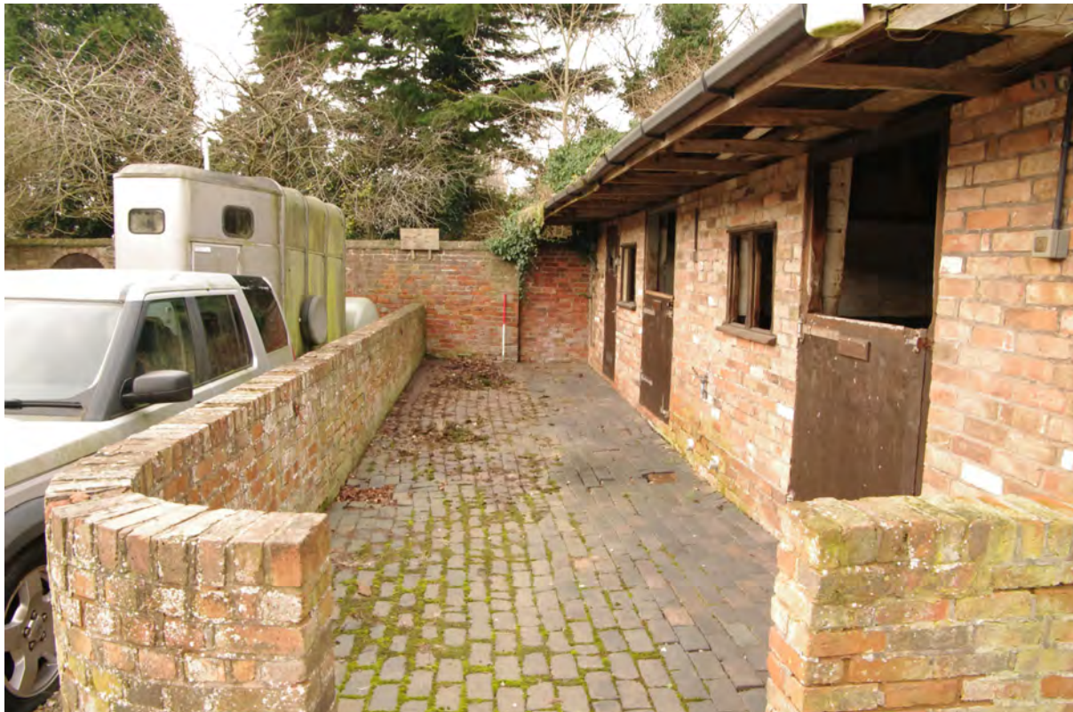
Figure 39: Yard in front of the south-western stable building Looking south-west. 1m scale
