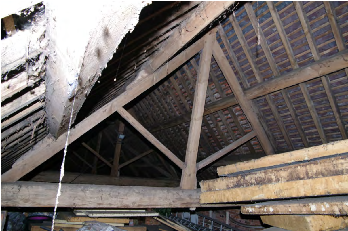
Figure 35: Threshing barn roof structure Looking north-east. Taken from stairs at the western end of the building
