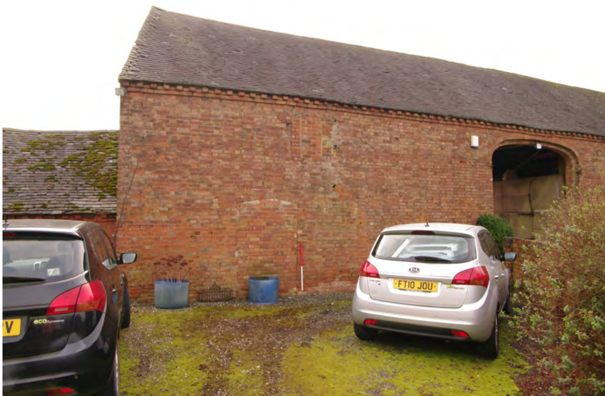
Figure 26: Threshing barn. Eastern end of the north-west facing elevation Note the blocked doorway to the left of the 1m scale. Another first floor window above the scale has been blocked
