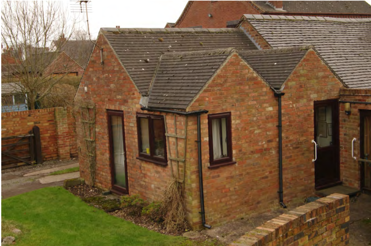
Figure 50: The office annex Looking south-east
