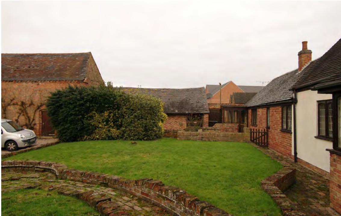
Figure 23: View of the yard looking NNE
