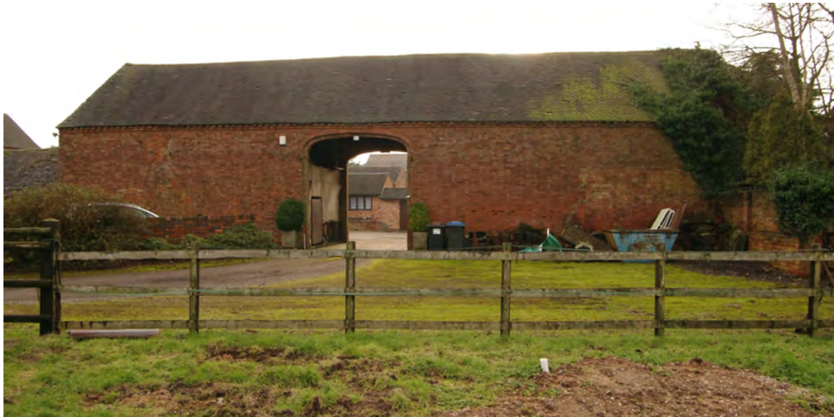
Figure 25: North-west facing elevation of the threshing barn Looking southeast
