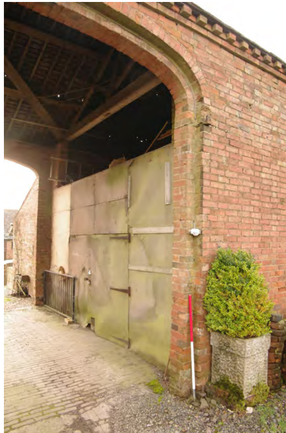
Figure 29: Threshing barn. North-west facing elevation doorway detail Note the door pintles. 1m scale
