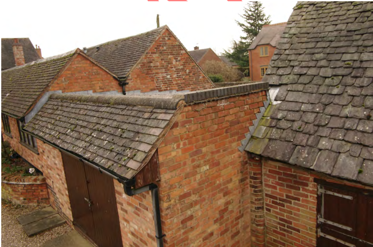
Figure 24: Flat-roofed section on the southern range
