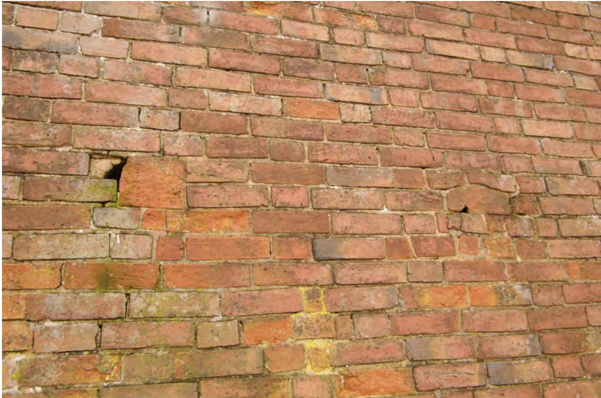
Figure 27: Threshing barn vents. Eastern end of the north-west facing elevation Note the two blocked vents which are located below the blocked window shown in Figure 26
