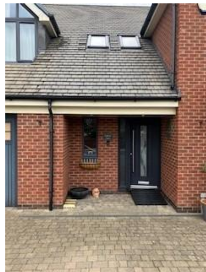
Figure 15: Front access to be altered.
