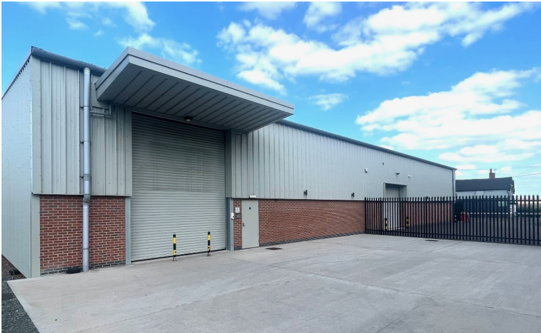
Figure 2: The existing building at The Redgate Depot
