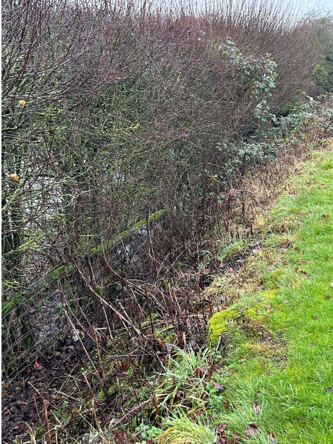
Photo 4 – existing outfall to ditch
