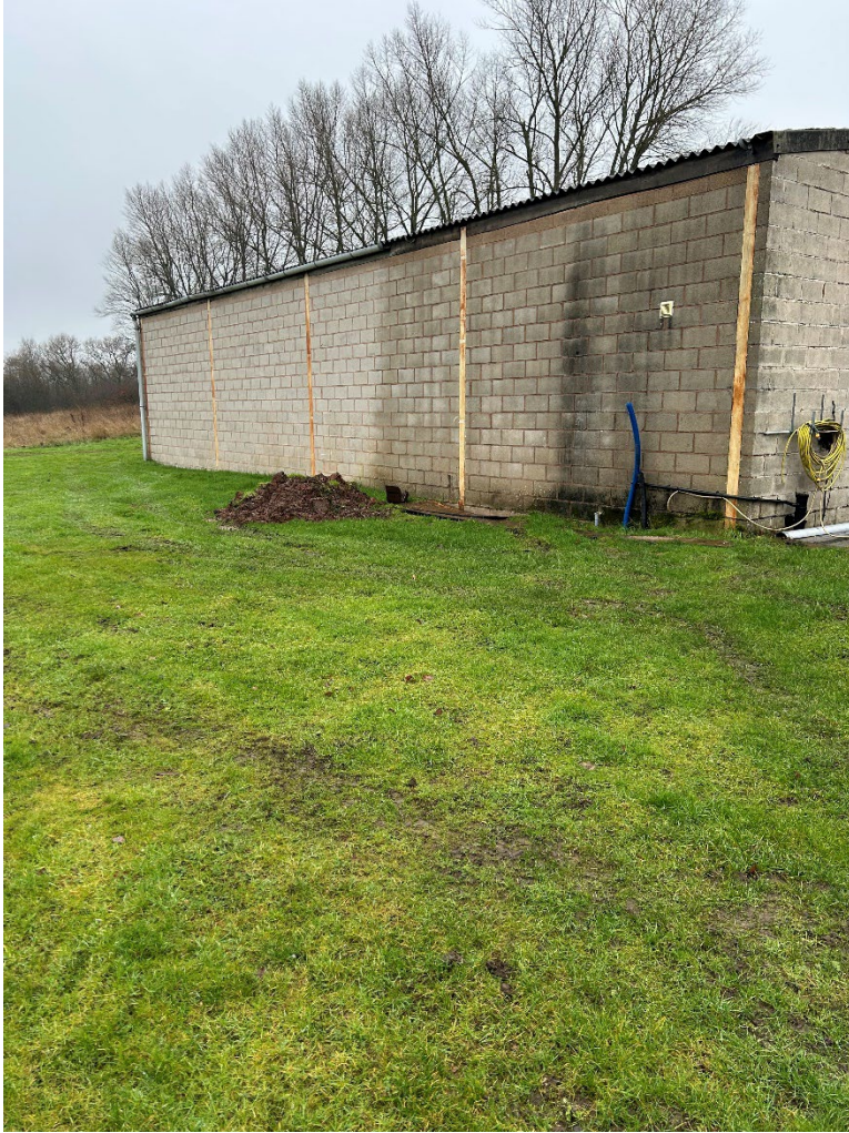
Photo 3 – existing agricultural building, showing existing rwp.
