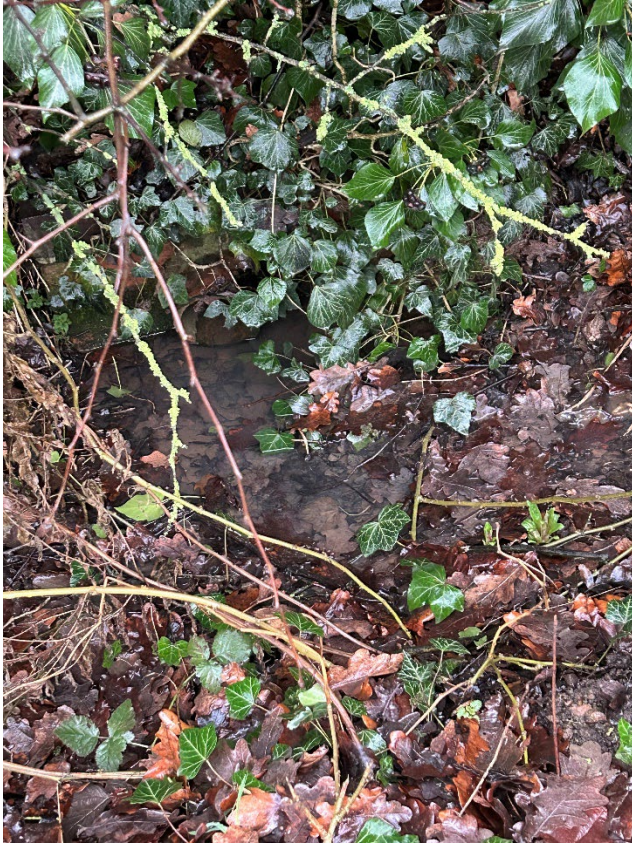
Photo 5 – another existing outfall to ditch
