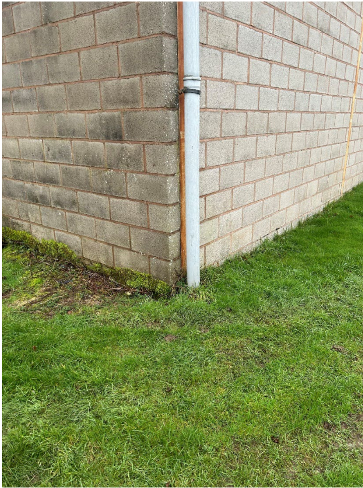
Photo 1 – existing rainwater pipes from existing agricultural building
