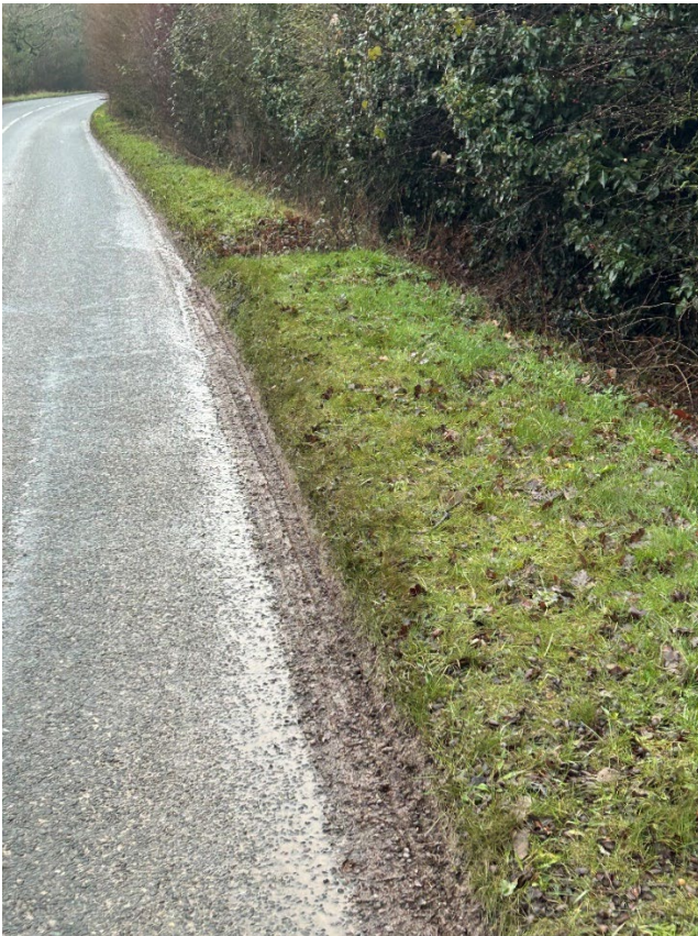
Photo 6 – existing ditch that existing agricultural building discharges into along Heath Road.
