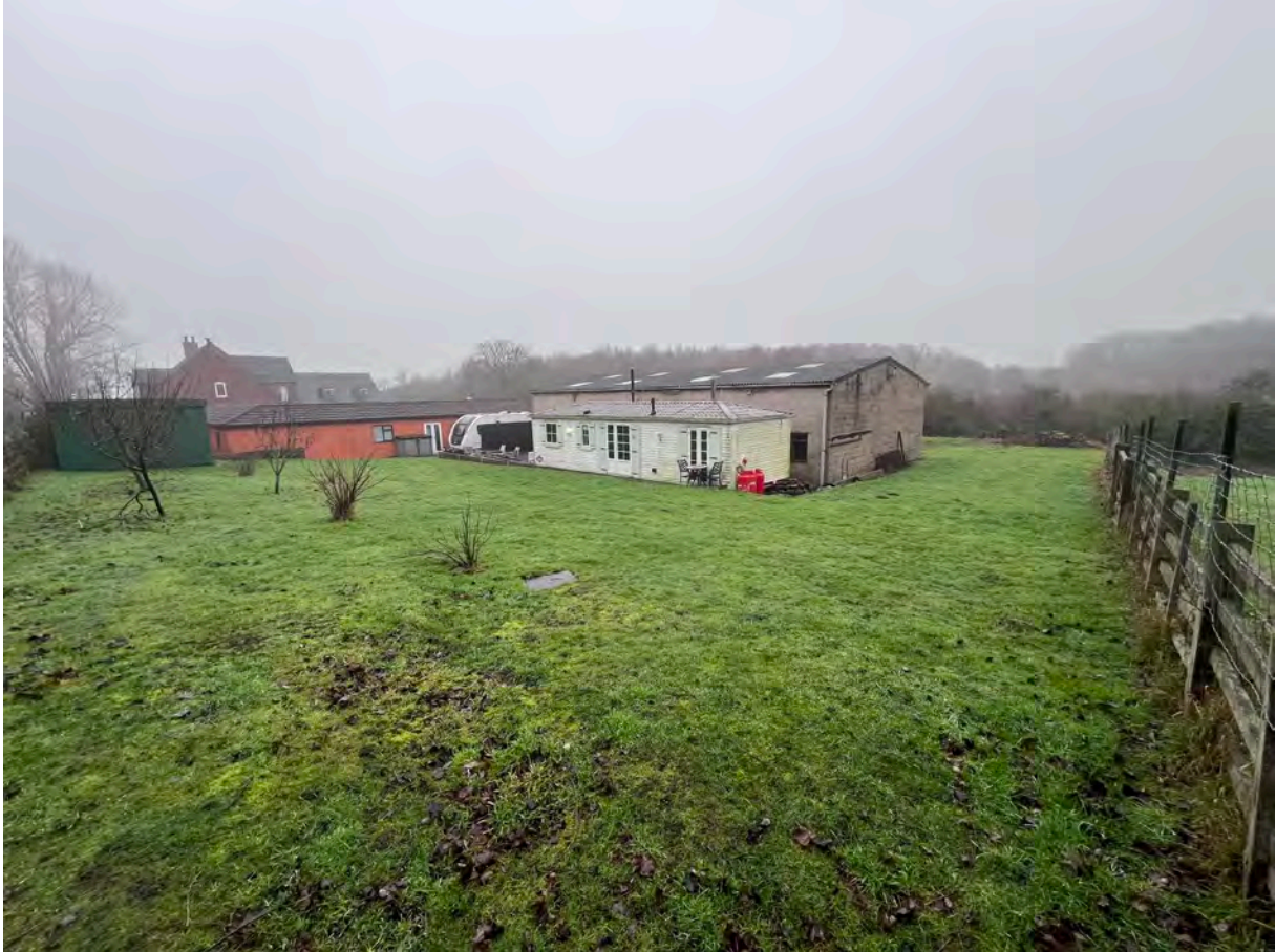
Photograph 6 – View across site from the north east
