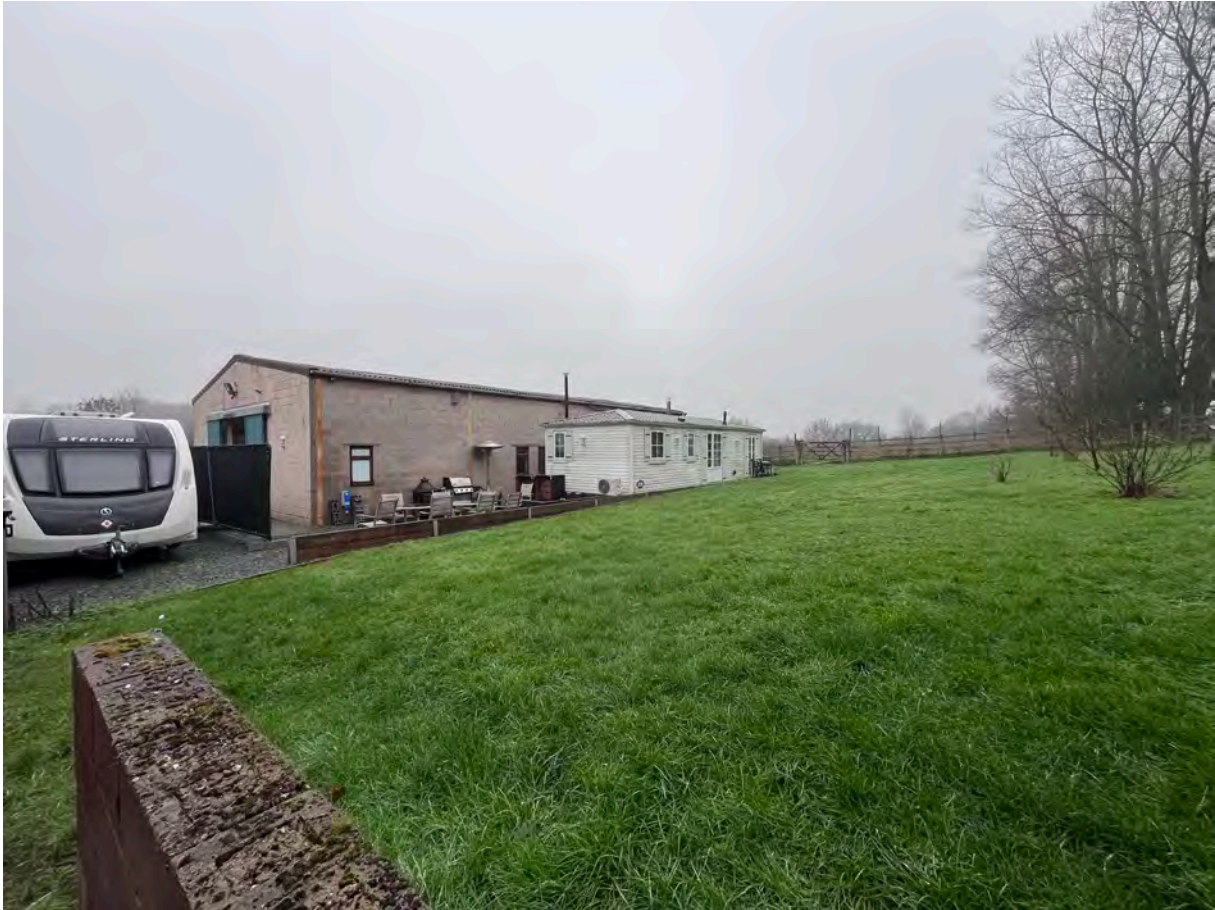
Photograph 5 – View across site from the south east
