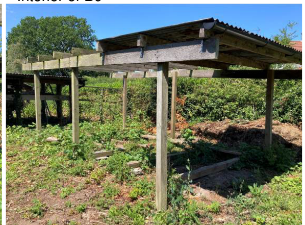
Open storage structure B11
