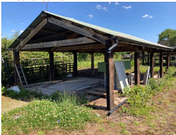
Covered storage area B6
