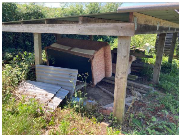
Timber frame store B2
