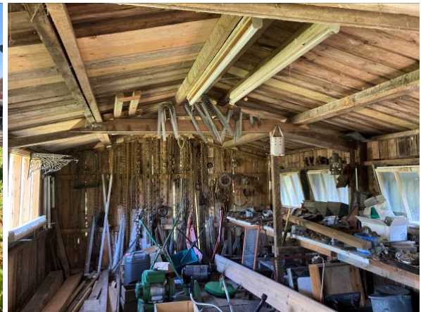
Interior of timber shed B8
