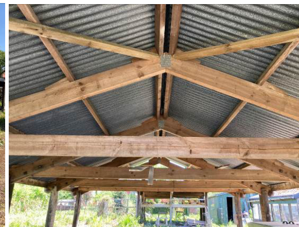
Underside of roof B6
