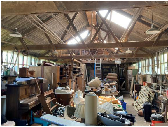
Interior of B3
