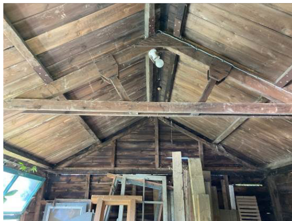
Interior of B1
