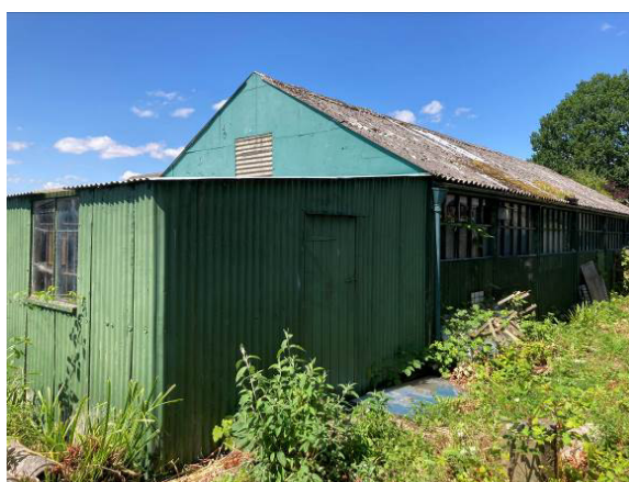
South end of workshop B3
