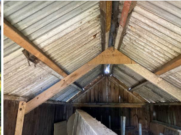
Interior roof of B4
