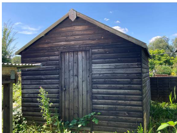
Timber shed B1
