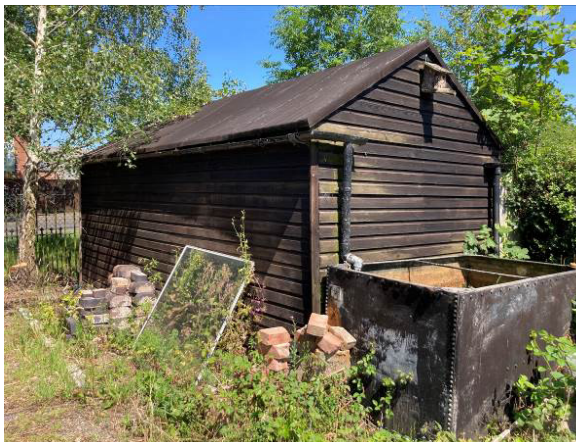
Timber shed B5
