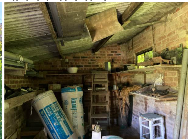
Interior of B9
