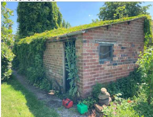
Brick outbuilding B9
