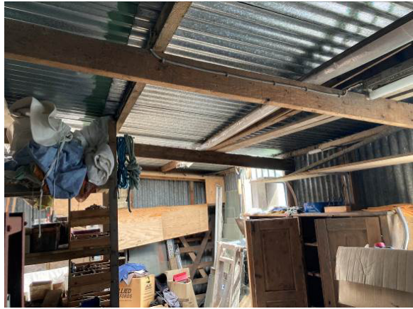
Extension roof interior of B3
