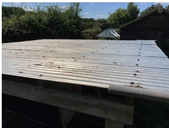
Flat roof of B2
