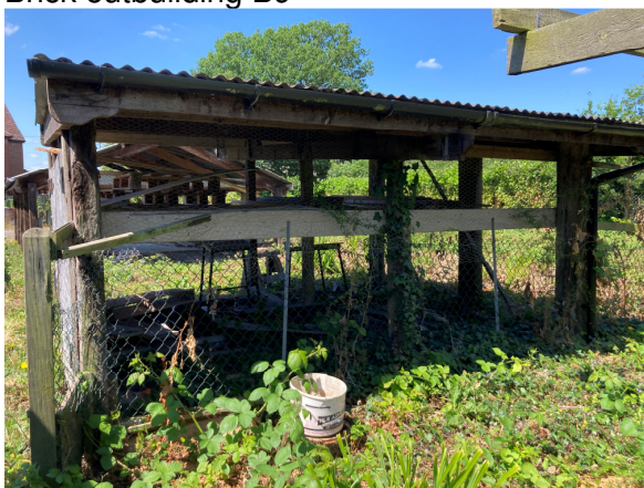
Open storage structure B10
