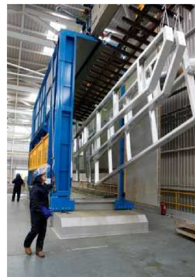
Steel elements being withdrawn from a typical hot-dip galvanizing bath
