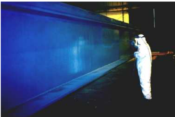
Airless spraying on steel bridge beams
