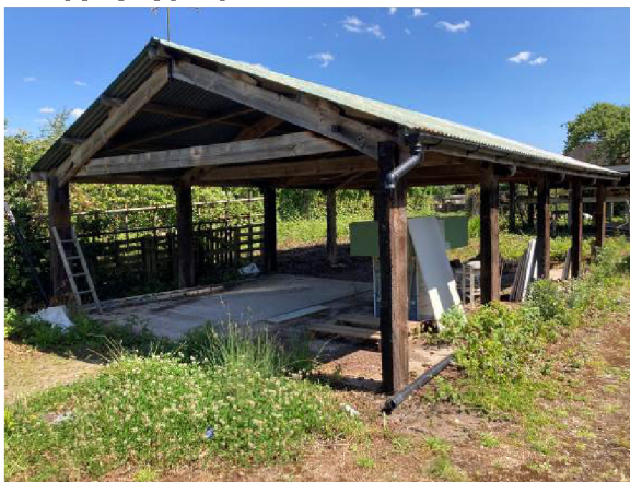
Covered storage area B6
