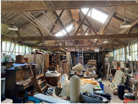
Interior of B3
