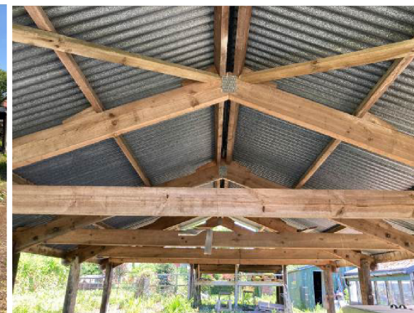
Underside of roof B6
