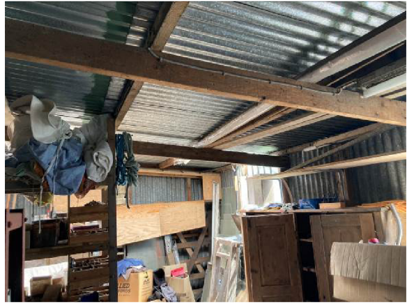
Extension roof interior of B3
