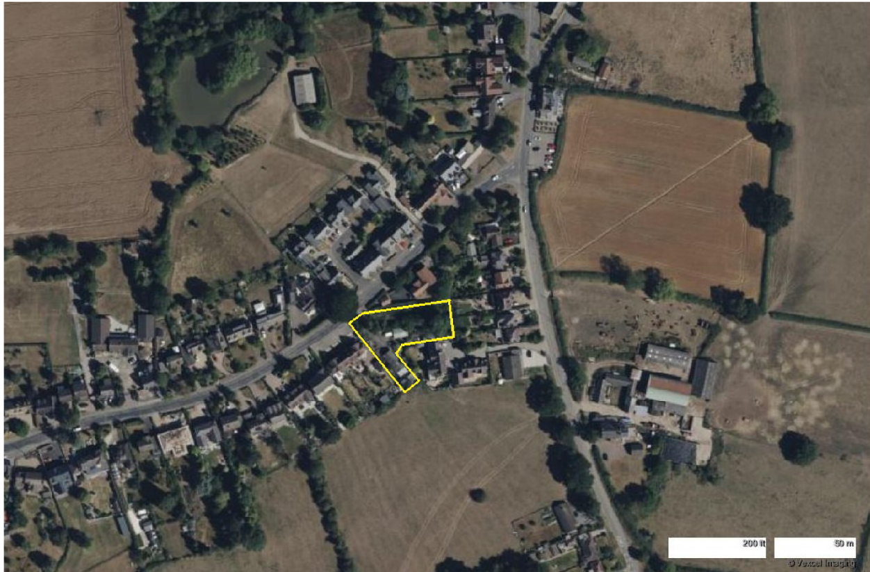
Figure 2: Site Contextual Aerial Photograph
