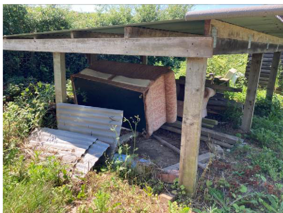
Timber frame store B2
