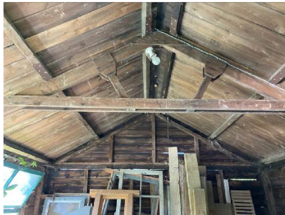
Interior of B1
