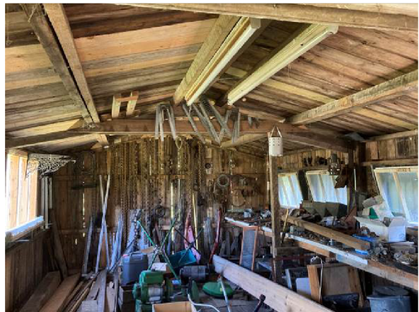
Interior of timber shed B8
