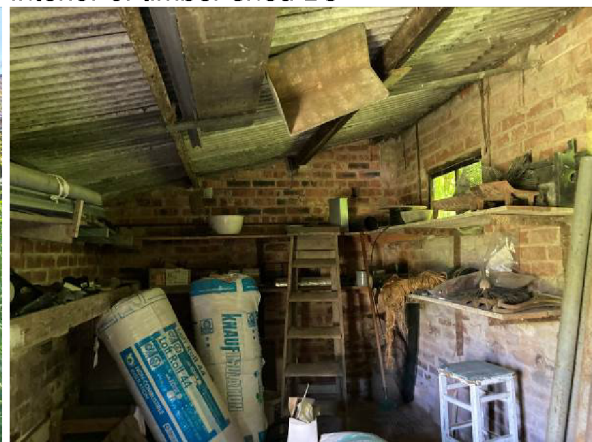
Interior of B9
