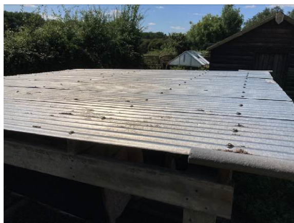
Flat roof of B2
