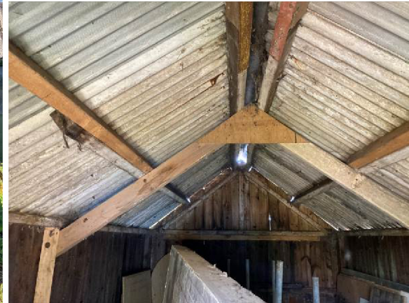
Interior roof of B4
