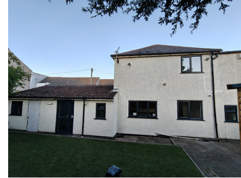
V1 B1-3 surveyor photo
