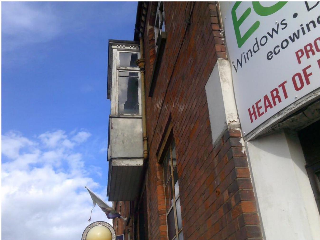
Bay window intact
