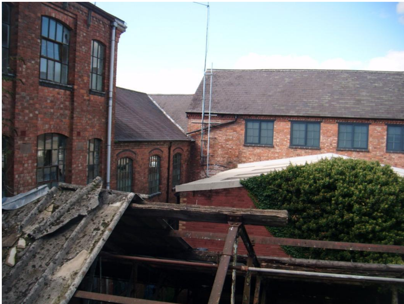
Intact roof internally to 2 storey structure
