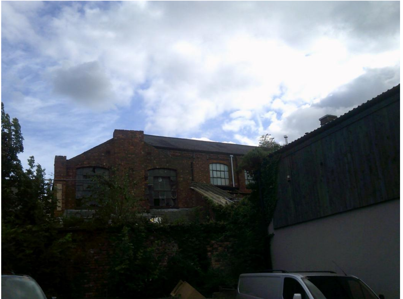
Rear view of roof B1
