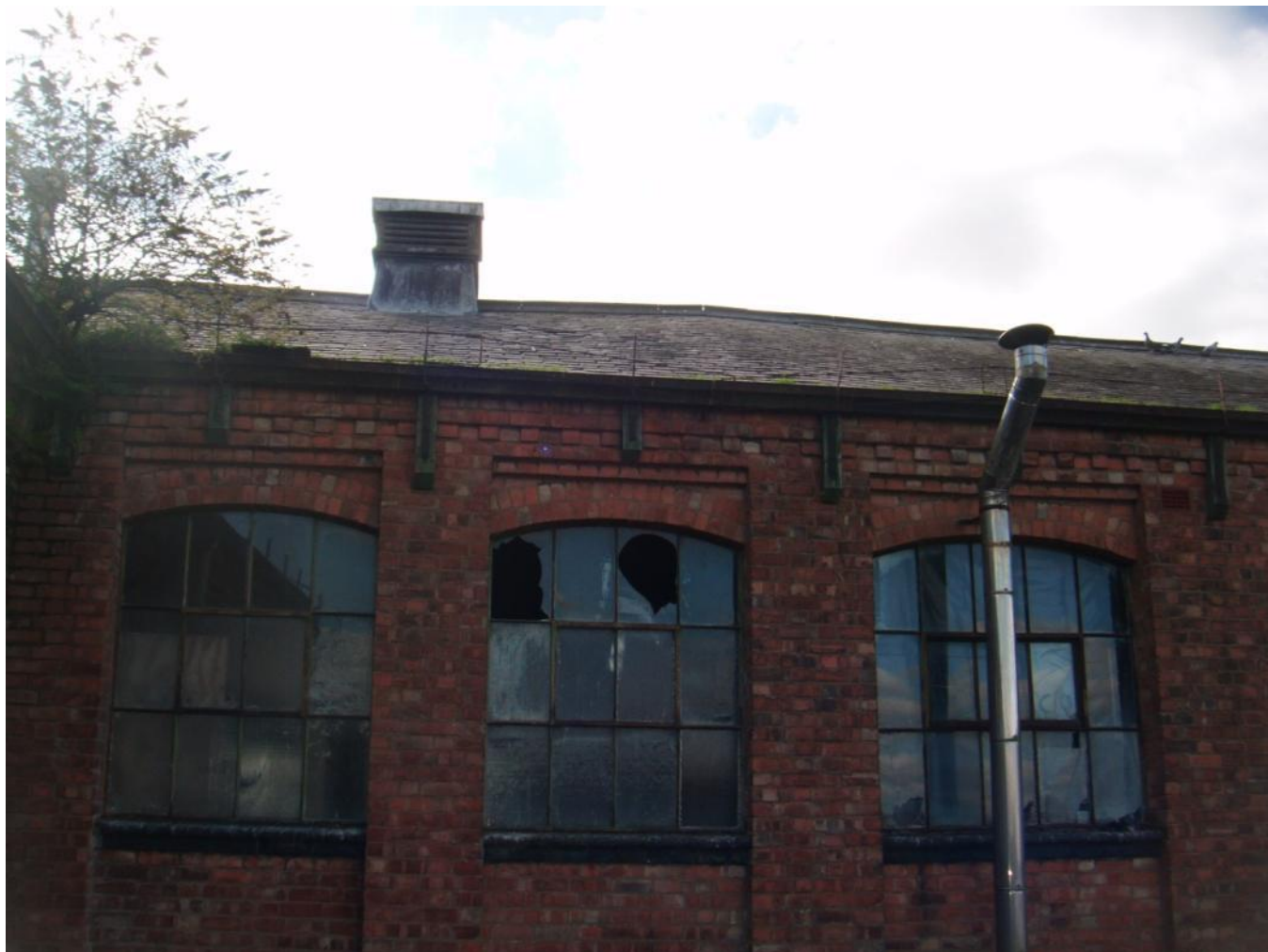
Roof intact, ventiation feature leads directly to second storey level (no void)
