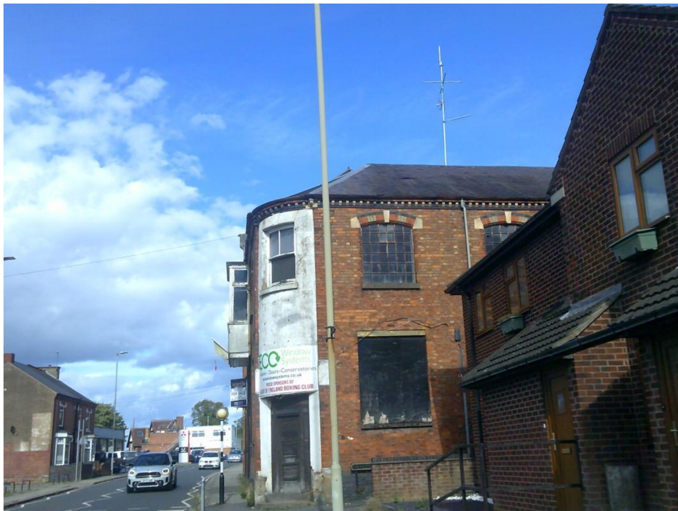
Building 2 external note 2/3 gaps in tiles on roof, flashing and brickwork intact
