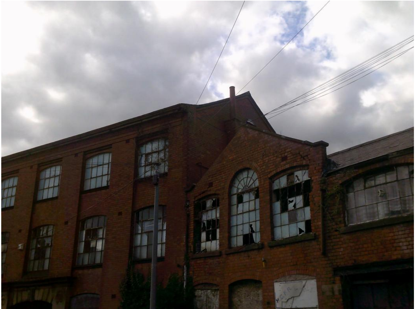
Gable end of 3 storey
