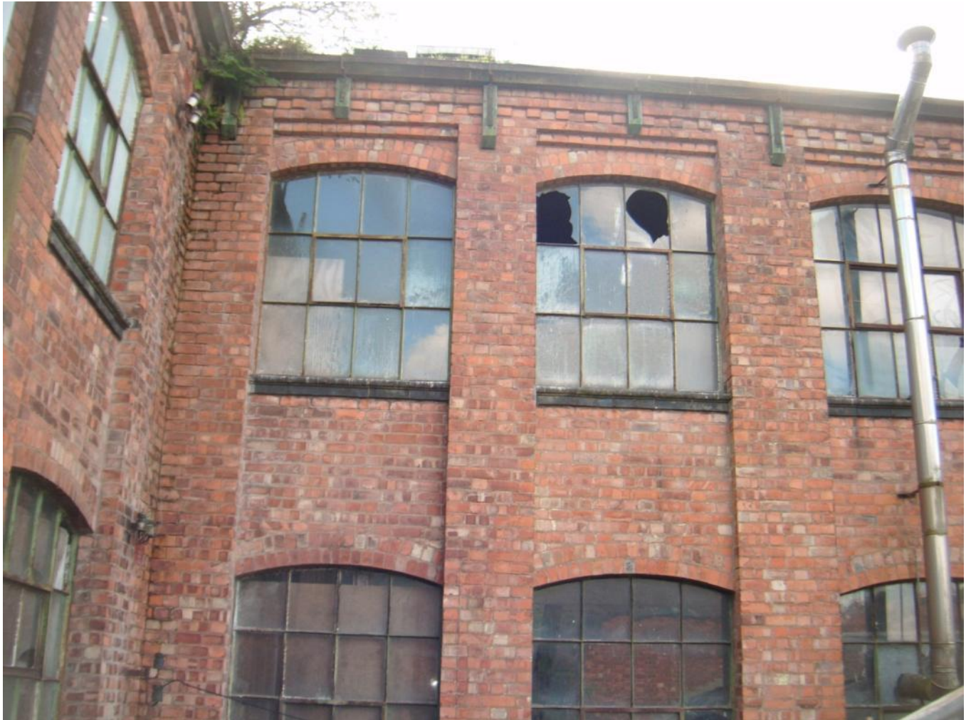
Courtyard: intact brickwork
