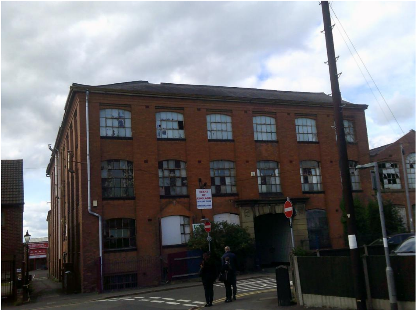
Intcat roof Druid street
