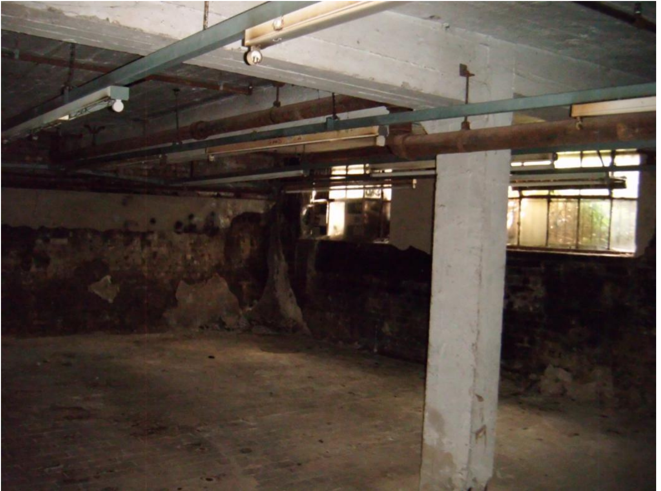
Cellar area: no bird or bat evidence
