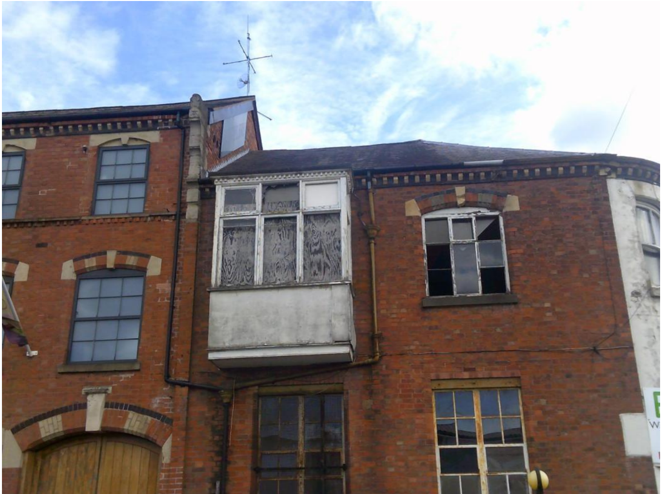
Interface of building 2 with adjoining building: intact
