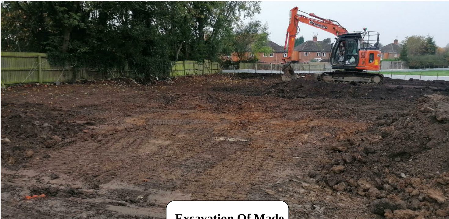
Excavation Of Made Ground and Topsoil
