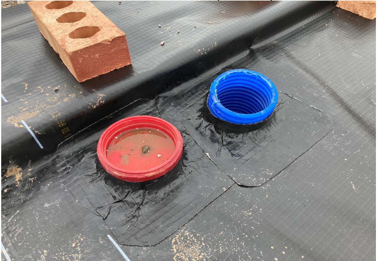
Plate 12 Plots 144 to 145 – Sealed Penetrations (31/05/2023)
