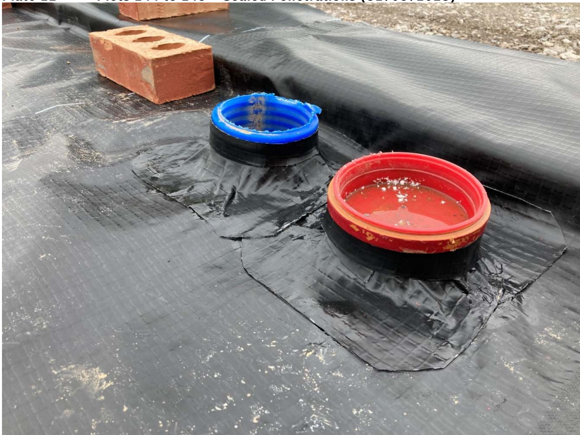
Plate 12 Plots 144 to 145 – Sealed Penetrations (31/05/2023)
