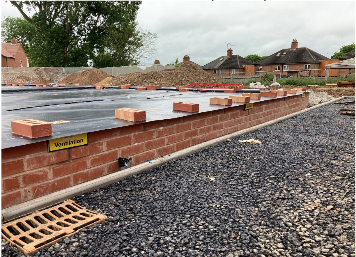
Plate 8 Plots 144 to 145 – Passive Vent Boxes (31/05/2023)
