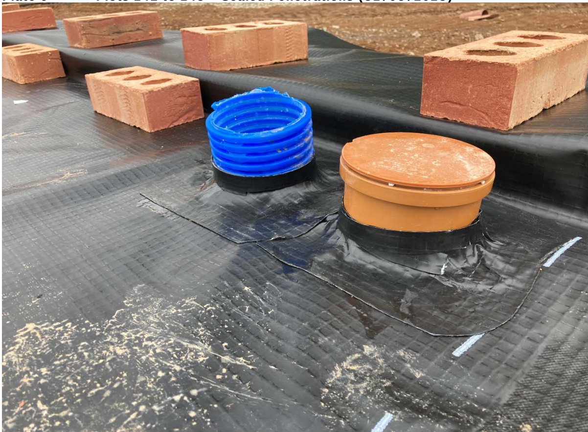
Plate 6 Plots 142 to 143 – Sealed Penetrations (31/05/2023)
