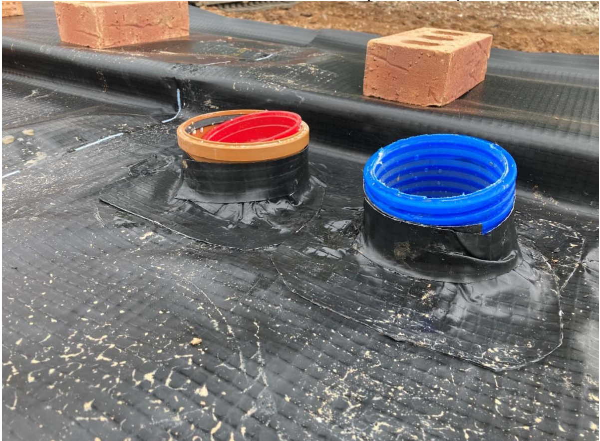
Plate 6 Plots 142 to 143 – Sealed Penetrations (31/05/2023)
