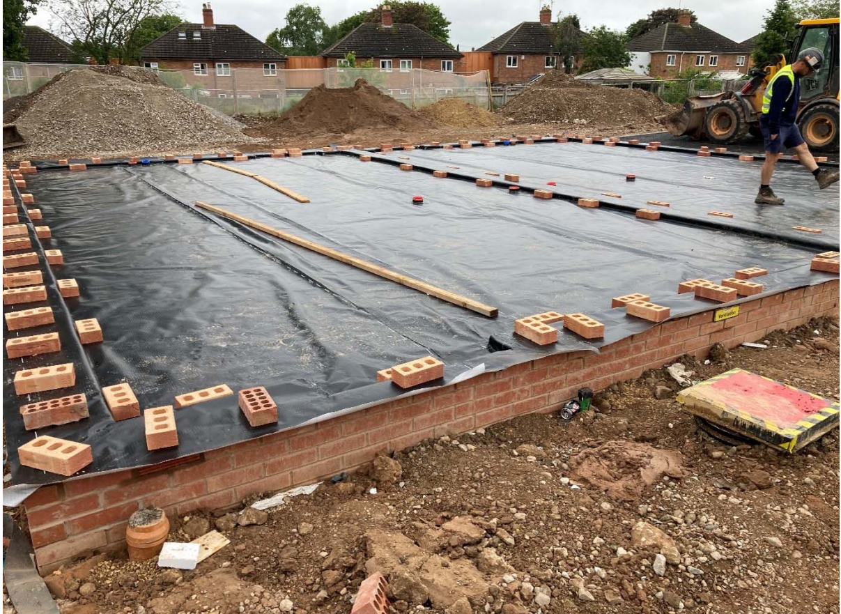
Plate 2 Plots 142 to 143 – Passive Vent Boxes (31/05/2023)
