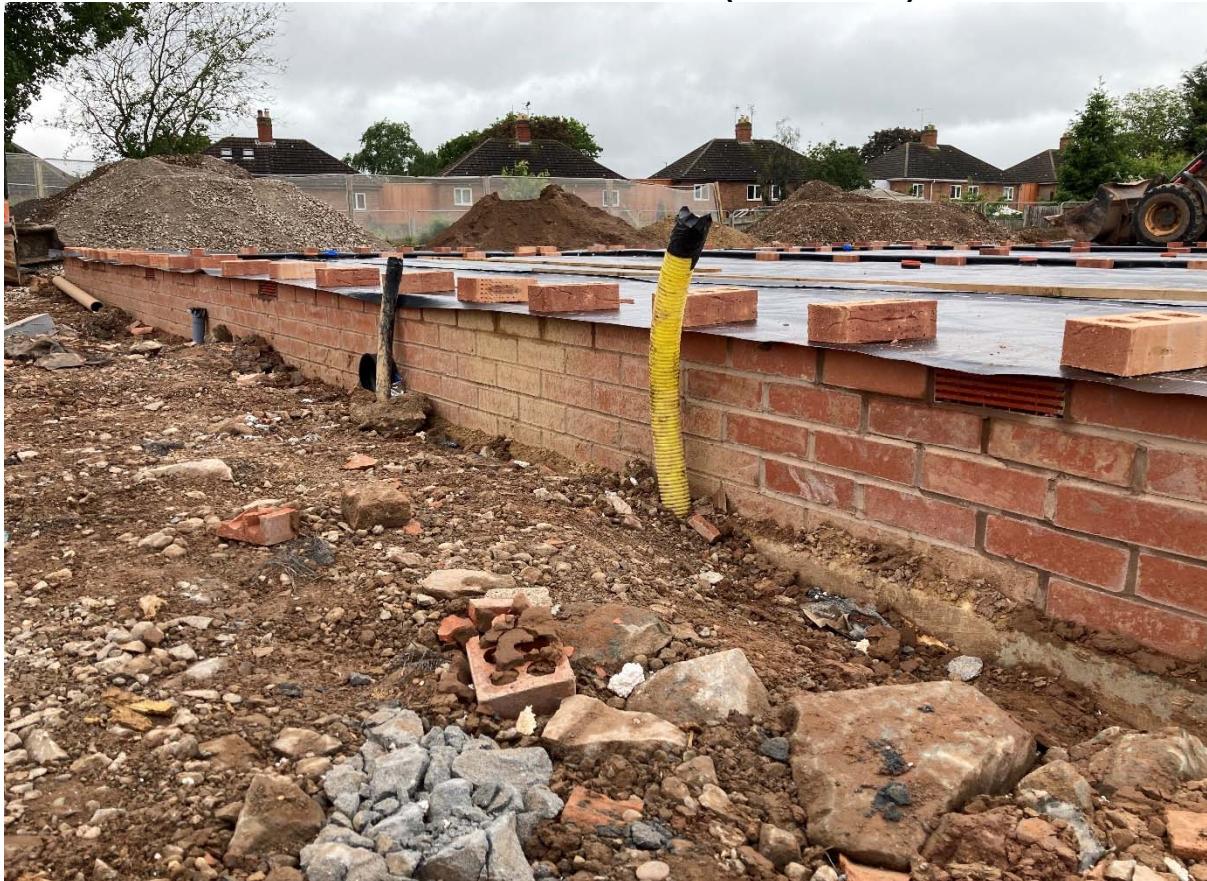
Plate 2 Plots 142 to 143 – Passive Vent Boxes (31/05/2023)
