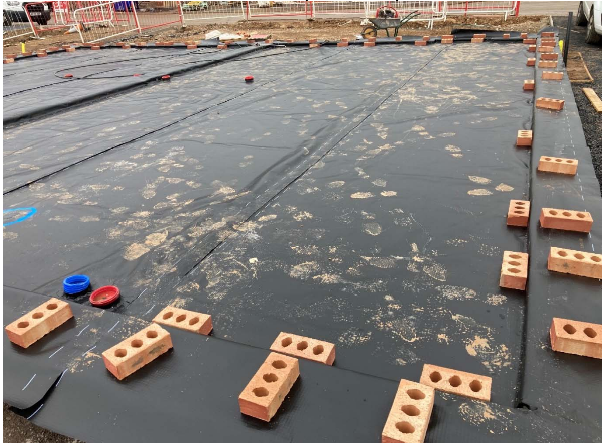
Plate 8 Plots 144 to 145 – Passive Vent Boxes (31/05/2023)
