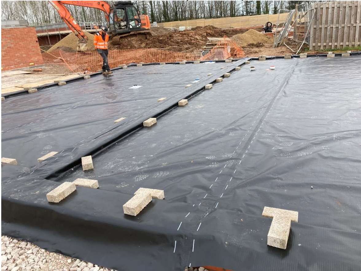
Plate 14 Plots 132 to 133 – Passive Vent Boxes (27/03/2023)
