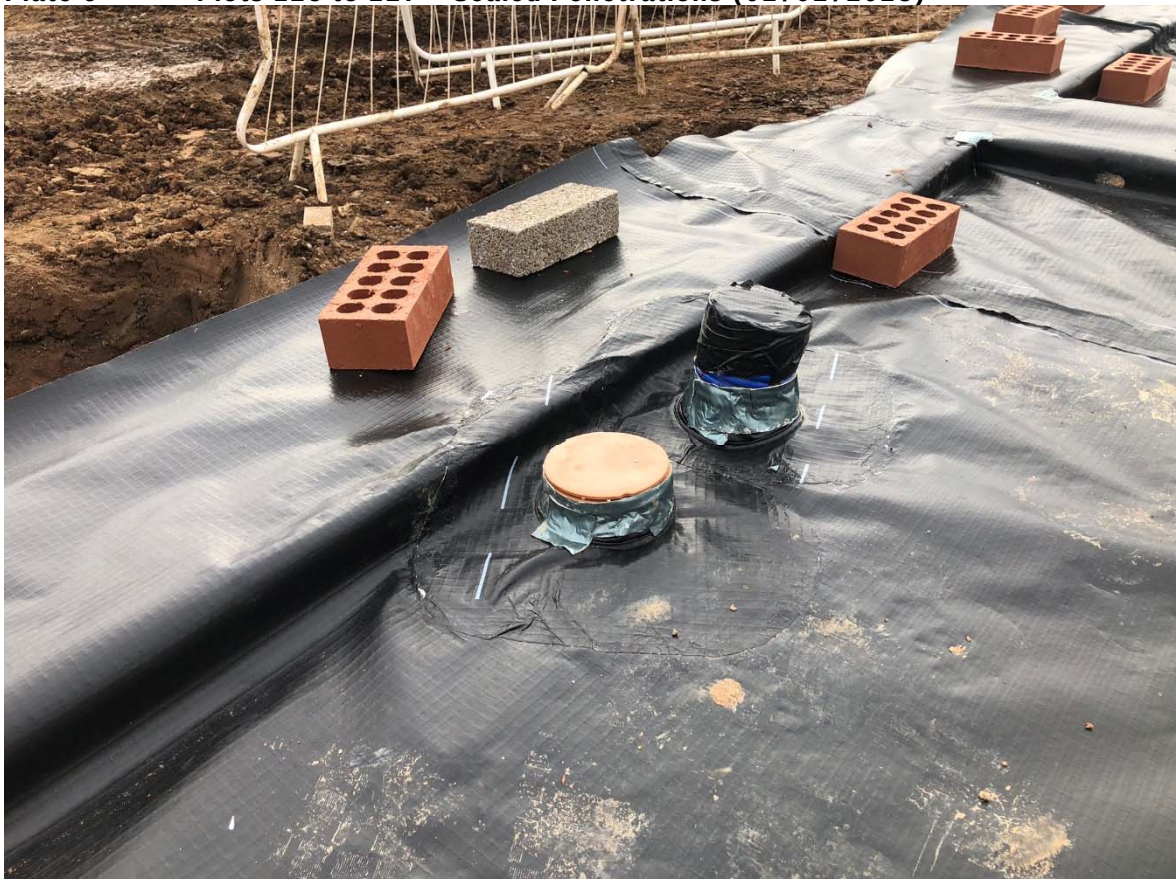
Plate 6 Plots 125 to 127 – Sealed Penetrations (02/02/2023)
