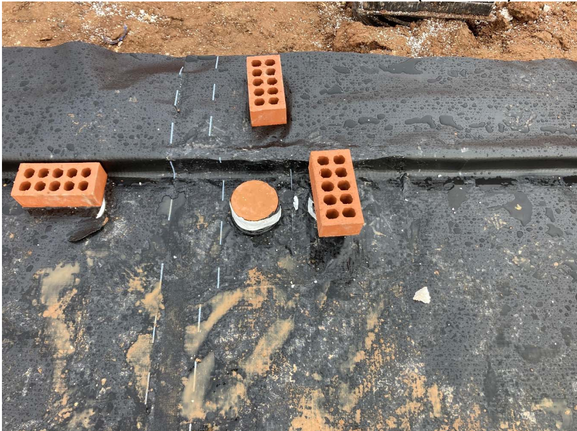
Plate 8 Plots 130 to 131 – Sealed Joint and Penetration (01/03/2023)
