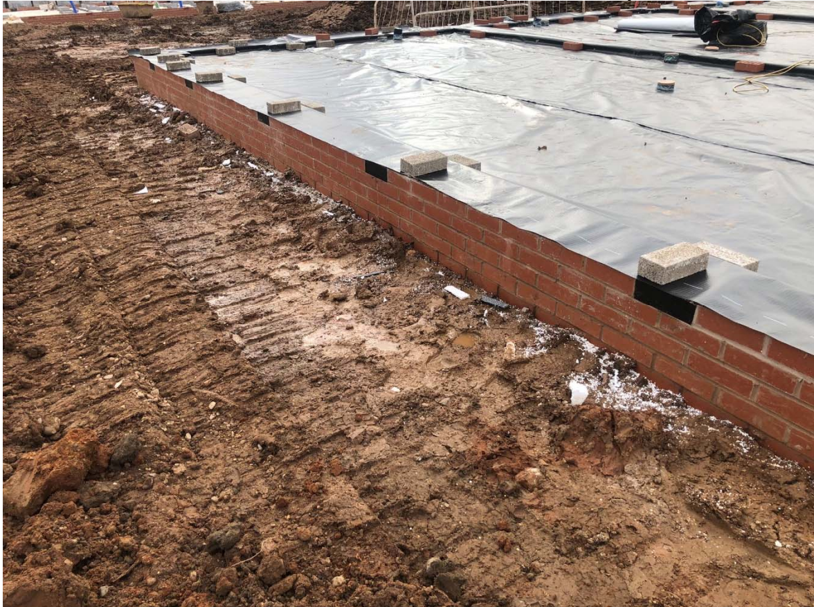
Plate 2 Plots 125 to 127 – Passive Vent Boxes (02/02/2023)
