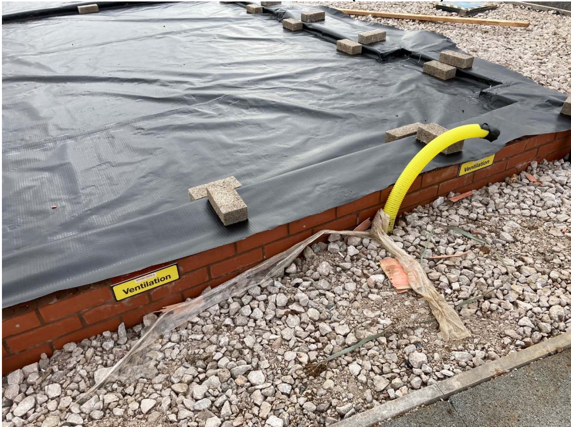
Plate 14 Plots 132 to 133 – Passive Vent Boxes (27/03/2023)
