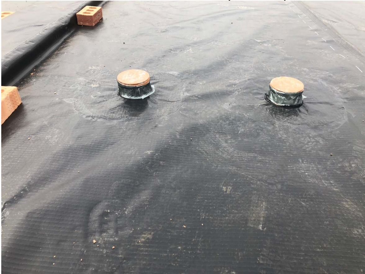
Plate 6 Plots 125 to 127 – Sealed Penetrations (02/02/2023)
