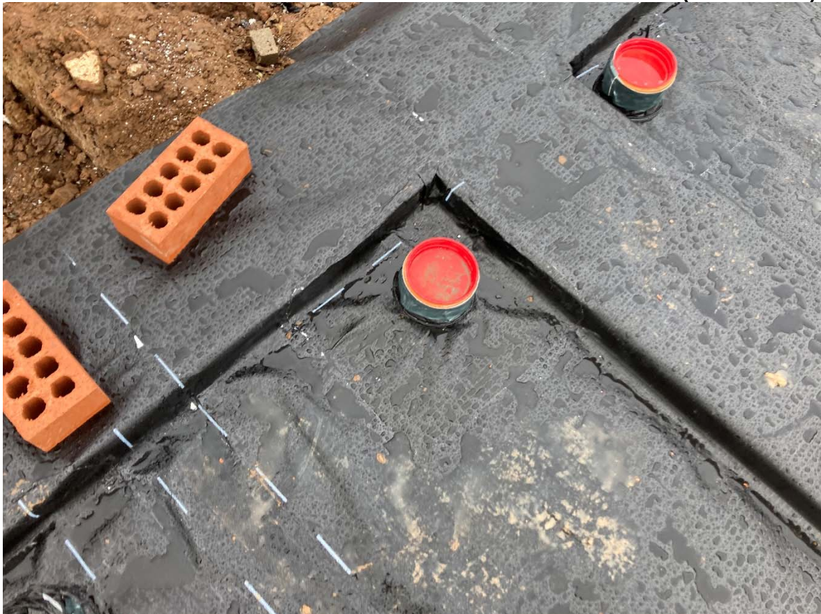
Plate 10 Plots 134 to 137 – Sealed Penetrations and Corner Detail (01/03/2023)
