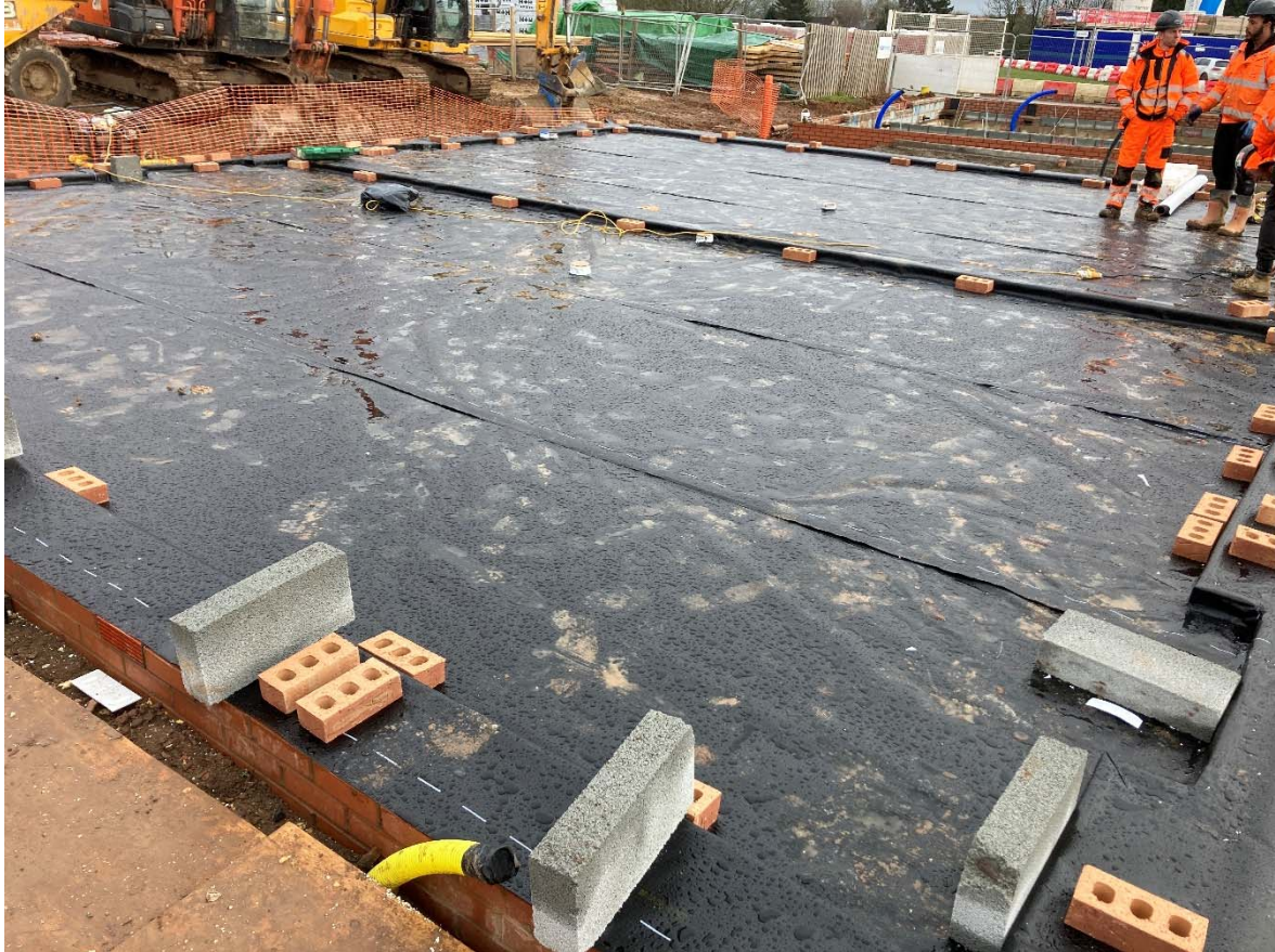
Plate 8 Plots 130 to 131 – Sealed Joint and Penetration (01/03/2023)
