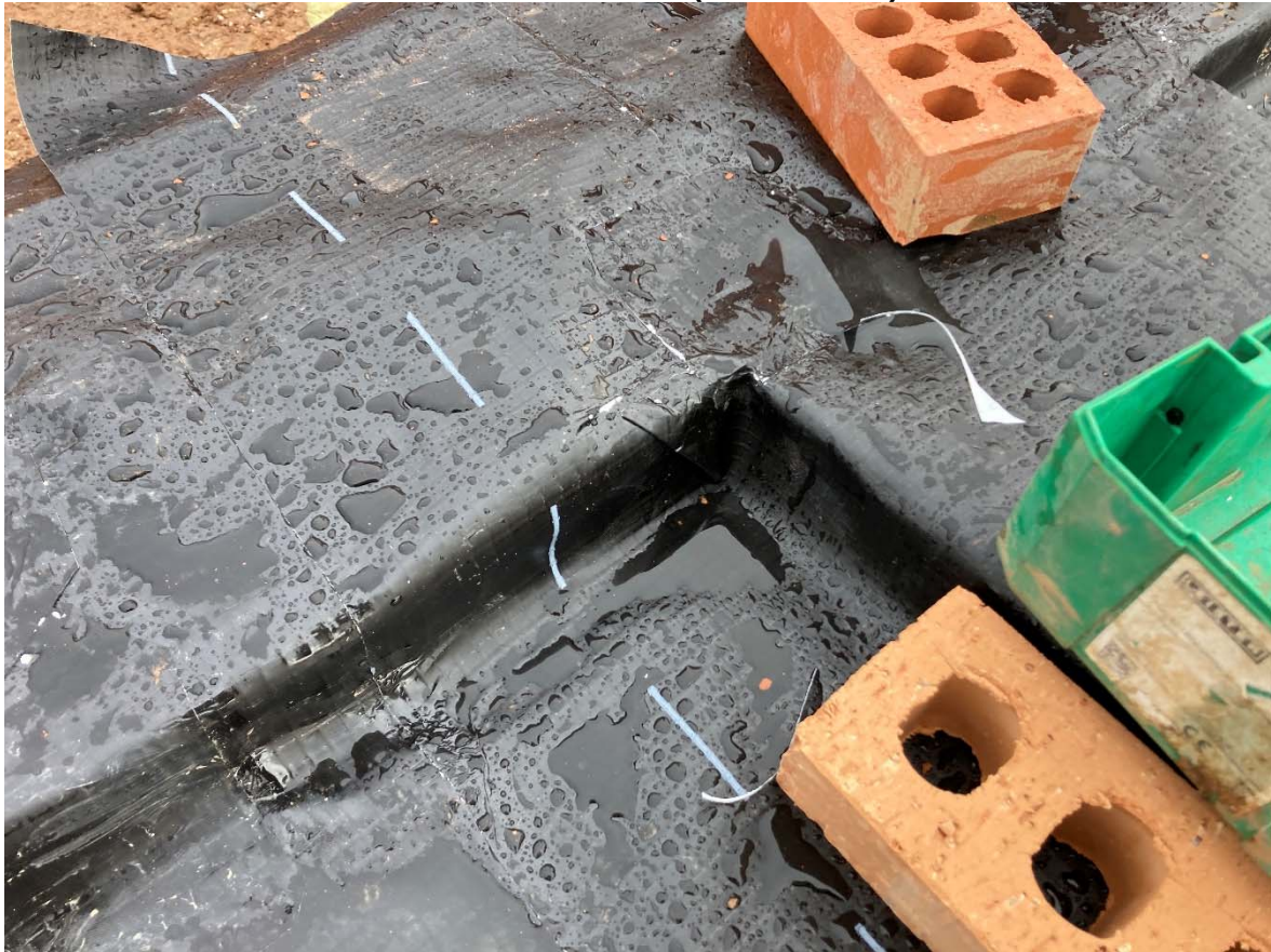
Plate 12 Plots 134 to 137 – Sealed Penetrations and Corner Detail (01/03/2023)
