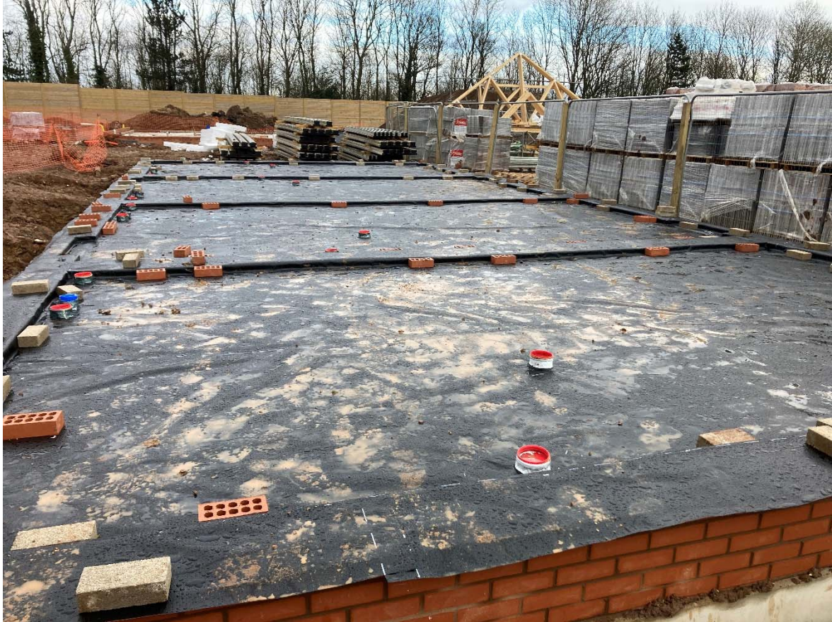
Plate 10 Plots 134 to 137 – Sealed Penetrations and Corner Detail (01/03/2023)
