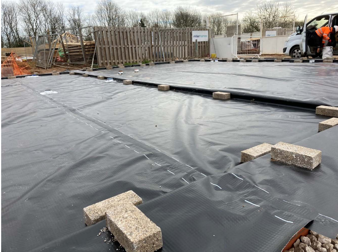
Plate 16 Plots 132 to 133 – Sealed Penetrations (27/03/2023)
