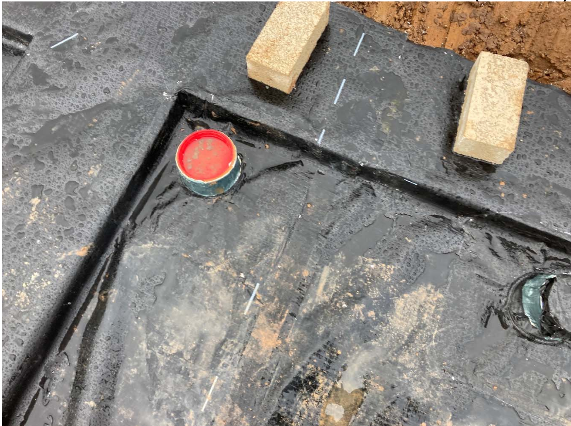
Plate 12 Plots 134 to 137 – Sealed Penetrations and Corner Detail (01/03/2023)
