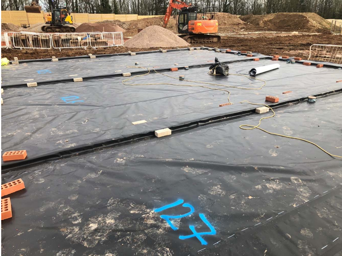
Plate 2 Plots 125 to 127 – Passive Vent Boxes (02/02/2023)
