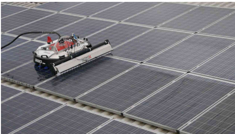
D. 003 – Cleaning of modules by Robot example
