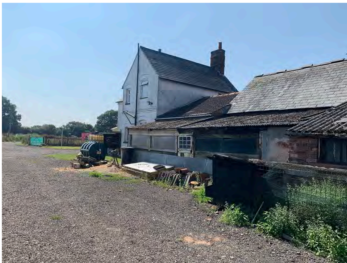
Figure 25: The farmhouse and outbuildings, looking south-east
