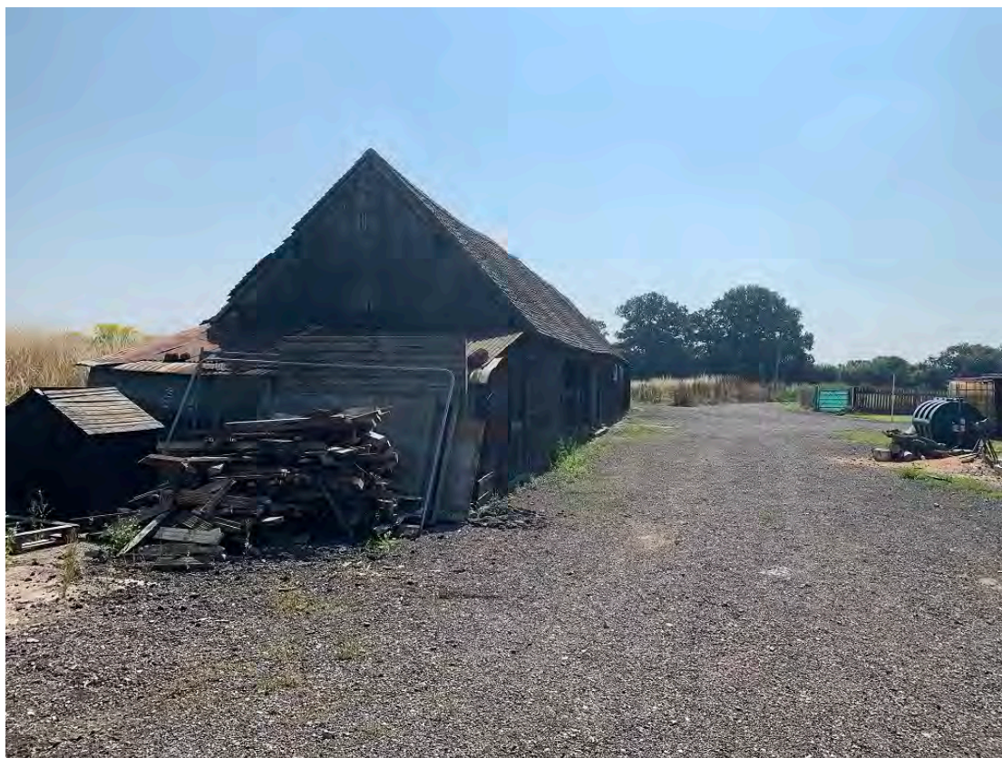
Figure 26: The shed opposite the farmhouse, looking east
