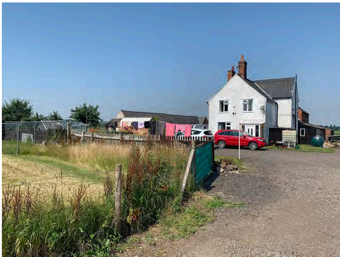
Figure 24: The farmhouse, looking west
