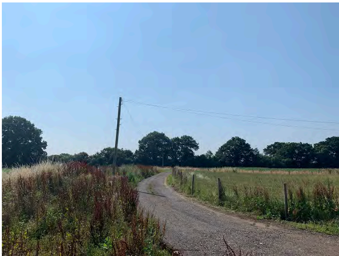
Figure 22: Power line crossing track close to farm, looking south
