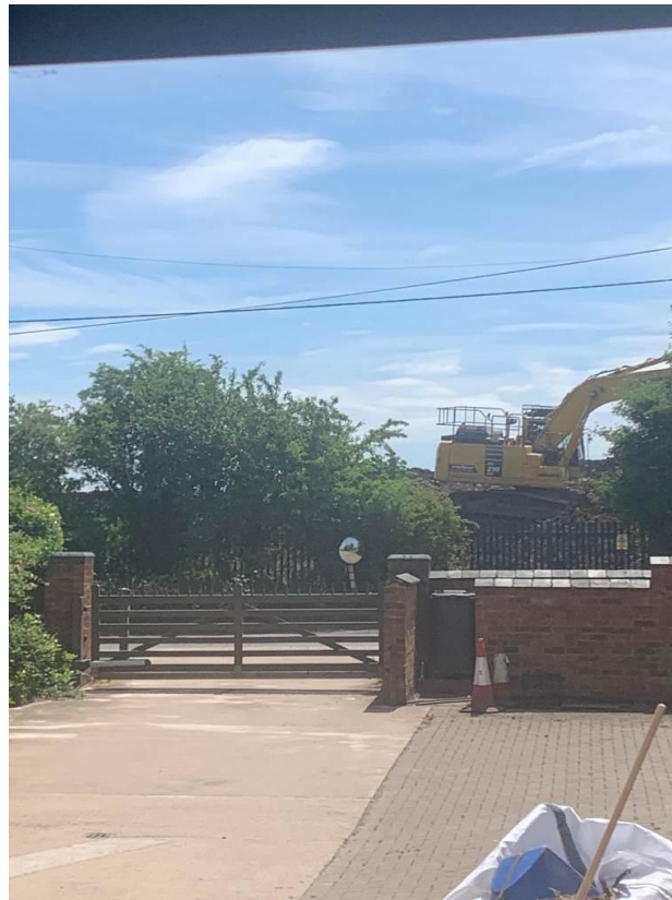
60. Heavy machinery on the Horiba Mira Automotive Proving Ground adjoining Fenn Lanes to the south (photograph taken from Willow Farm existing vehicular access)
