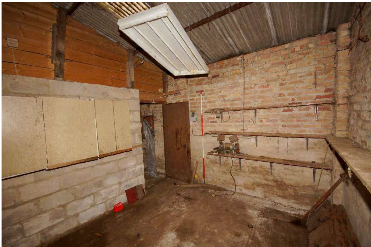
Plate 100: G10 – concrete blockwork partition with doorway to G9
