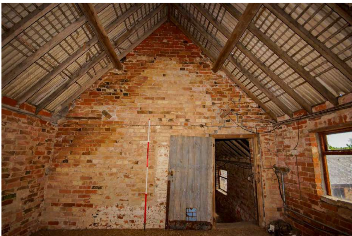
Plate 126: F2 – southeast gable wall with doorway to F3
