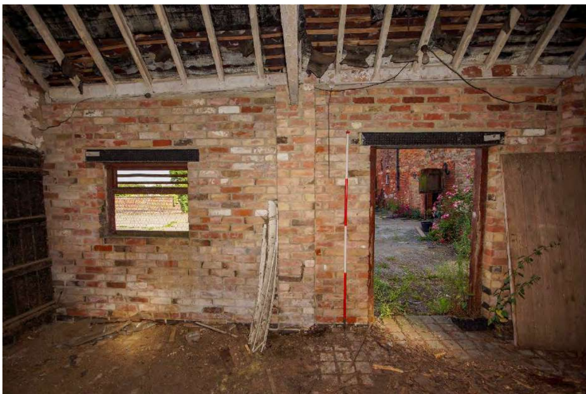
Plate 102: G11 – doorway to the courtyard
