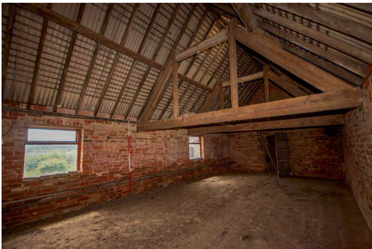
Plate 123: F2 – first-floor room of Building 2 with two queen-post trusses
