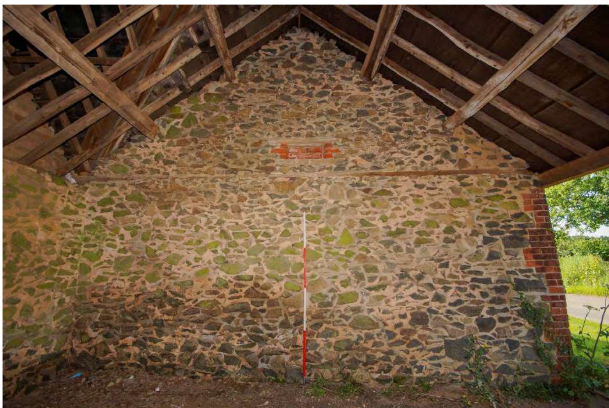
Plate 116: G13 – opposite gable wall with blocked opening
