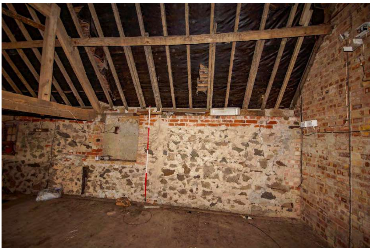
Plate 130: F3 – blocked window opening
