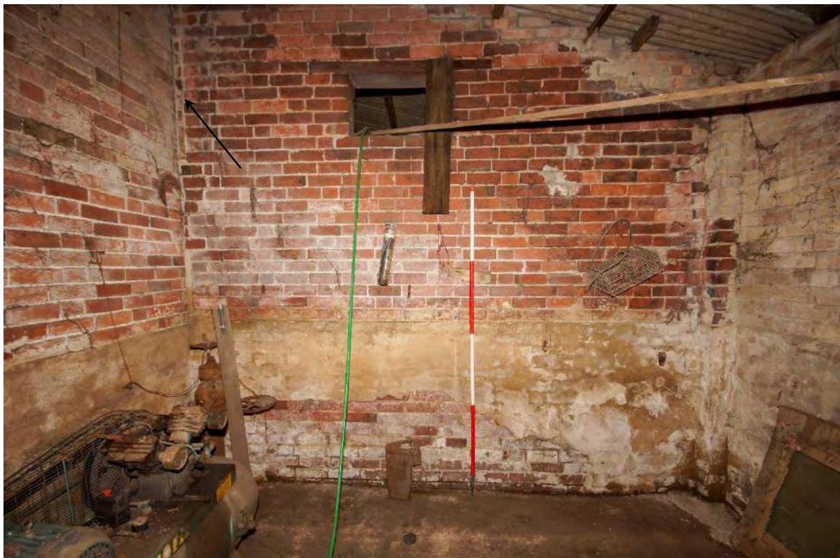
Plate 94: G8 – northwest wall with construction joint to the southwest end (arrow)
