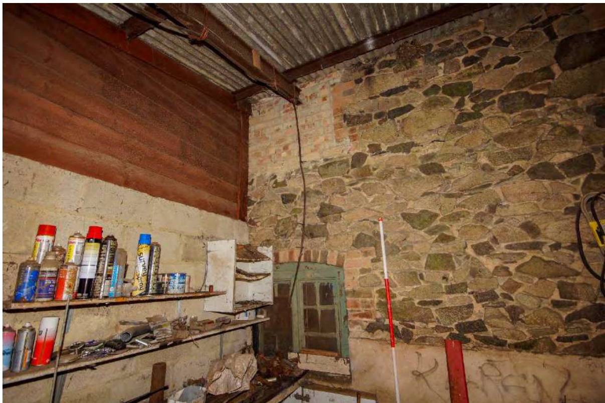
Plate 96: G9 – southwest wall with blocked first-floor window opening
