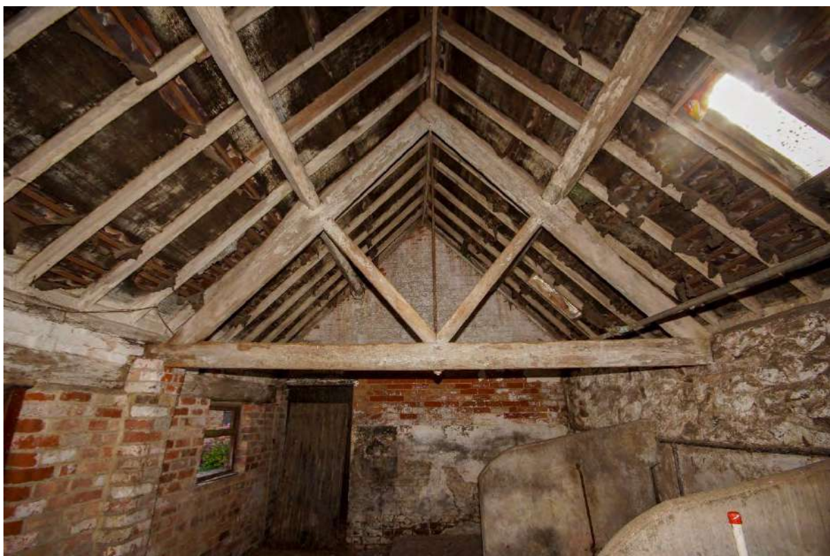
Plate 114: G12 – detail of composite king-bolt truss
