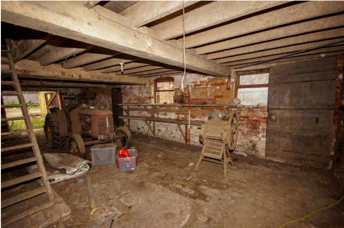
Plate 91: G7 – window openings to the courtyard
