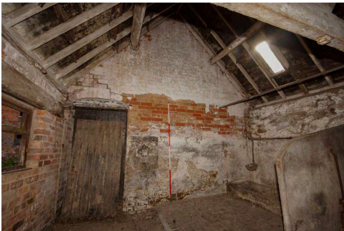
Plate 111: G12 – northeast gable wall with doorway to G11
