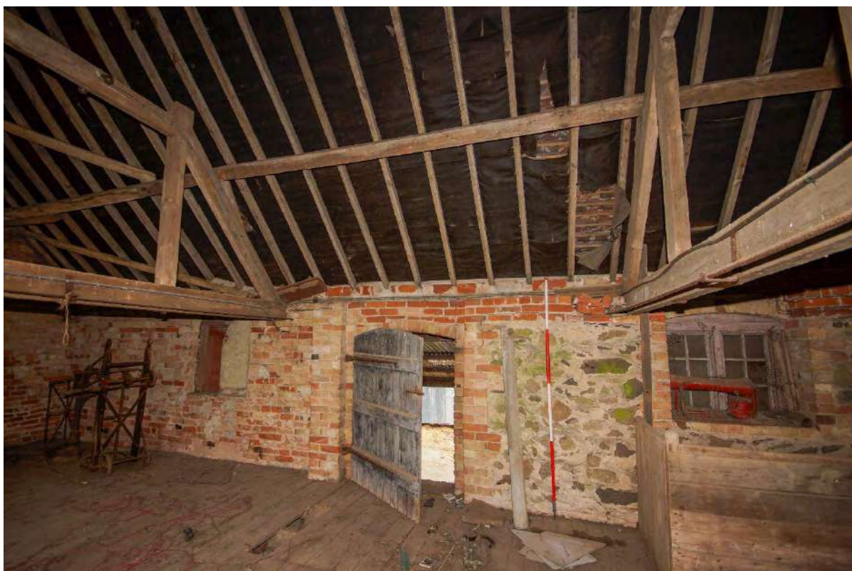
Plate 128: F3 – taking-in door to the rear northeast wall
