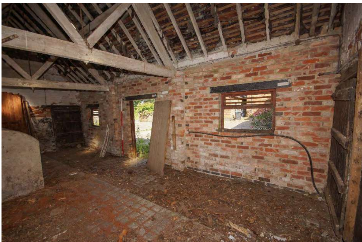
Plate 103: G11 – brick pillars and infilled brick panels with central window openings
