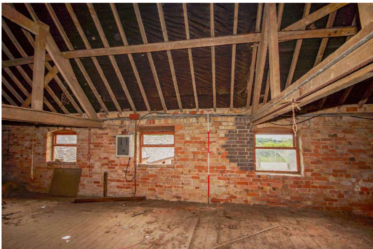
Plate 133: F3 – window openings to the courtyard
