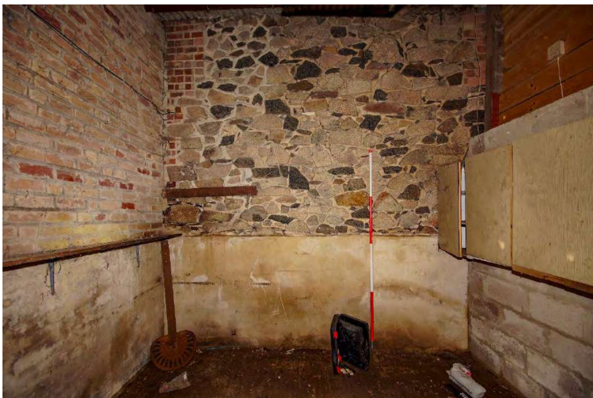
Plate 101: G10 – southwest wall with stone masonry and later cement plinth
