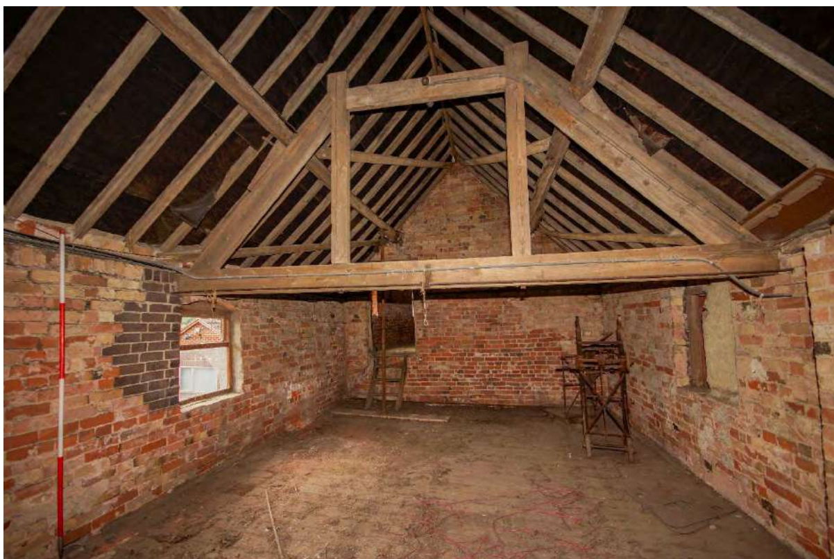
Plate 134: F3 – detail of queen-post truss
