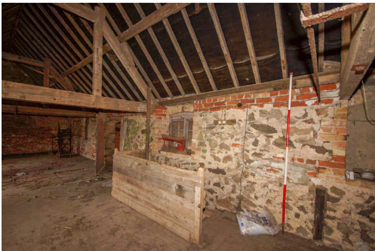
Plate 129: F3 – stone masonry within the northeast wall
