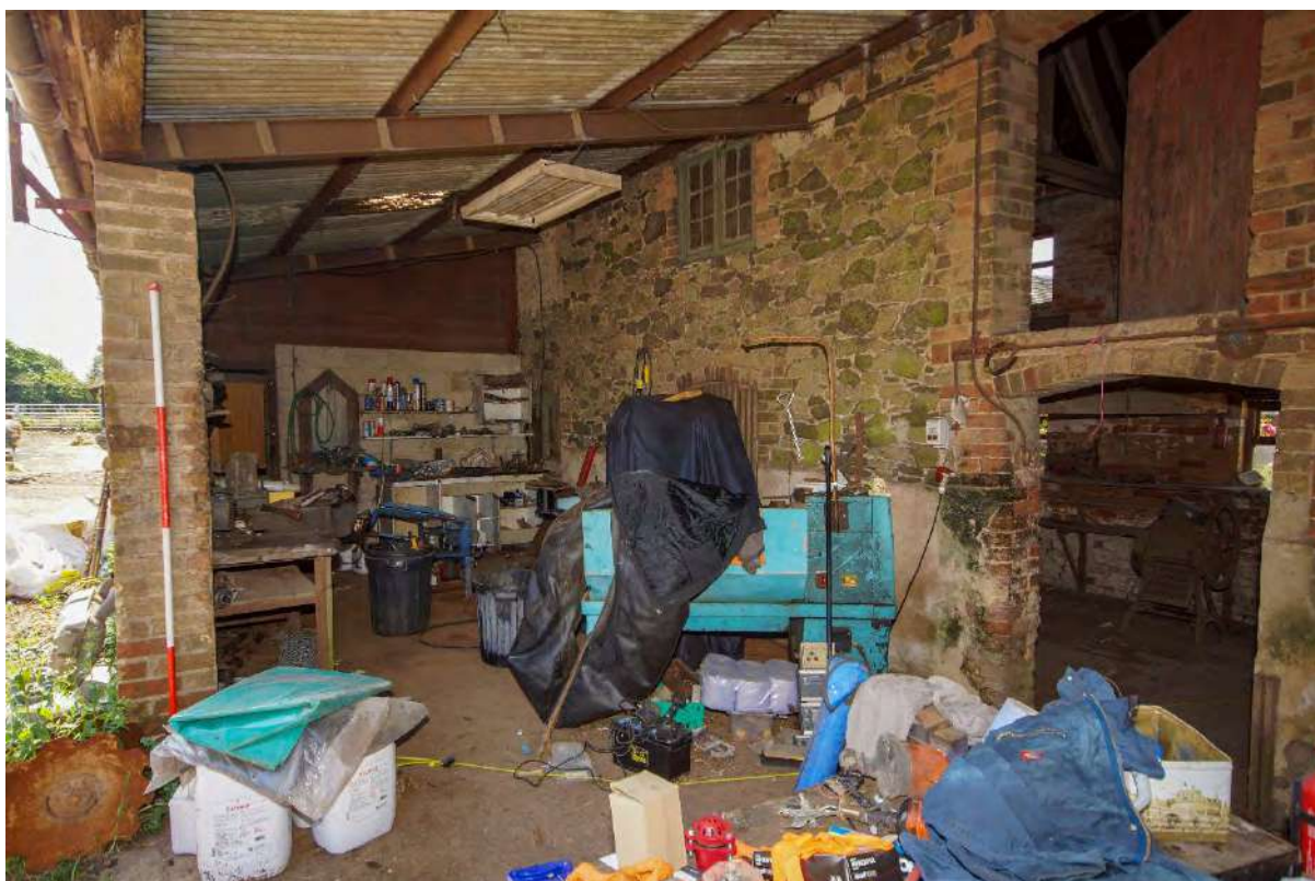
Plate 97: G9 – stone built southwest wall with window openings and doorways on each level
