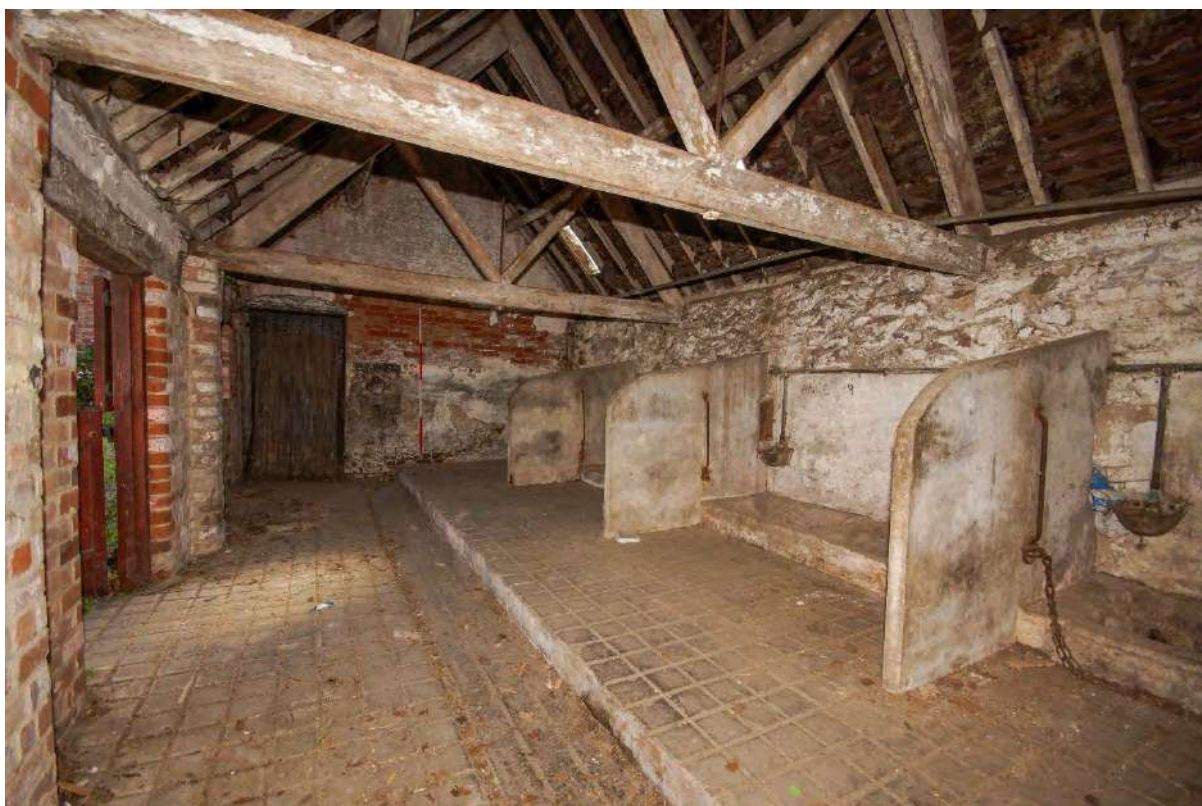
Plate 110: G12 – paved floor with drainage gully and boskin of former cow stalls
