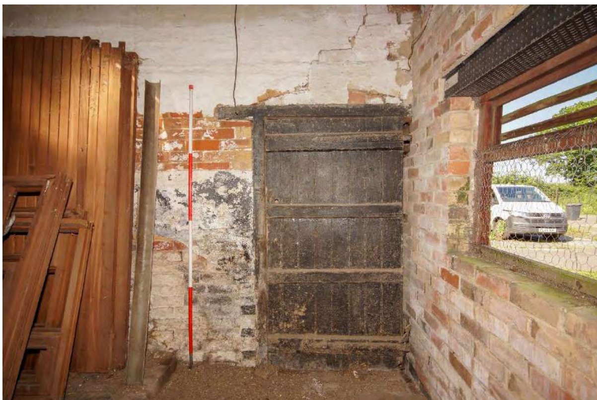
Plate 107: G11 – detail of ledged door
