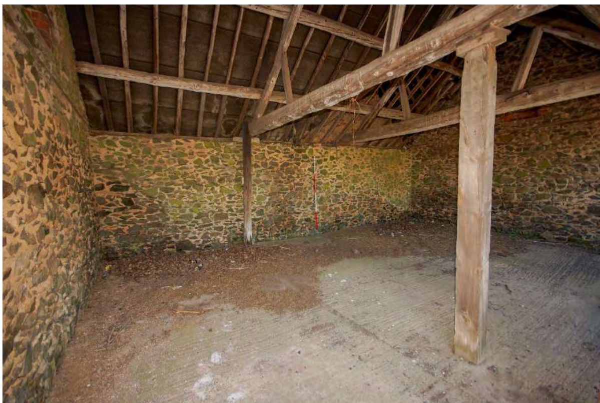
Plate 117: G13 – rear side wall to the northeast
