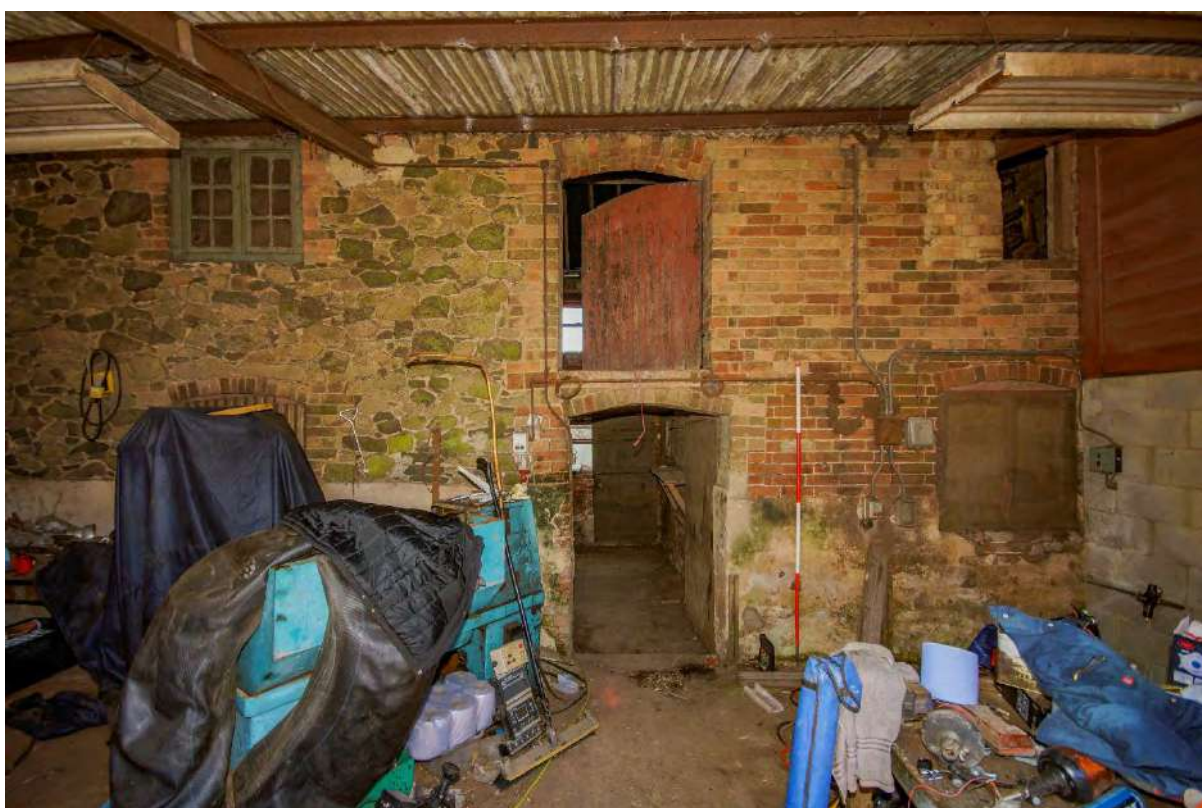
Plate 98: G9 – brick-built section to the northwest end of the southwest wall
