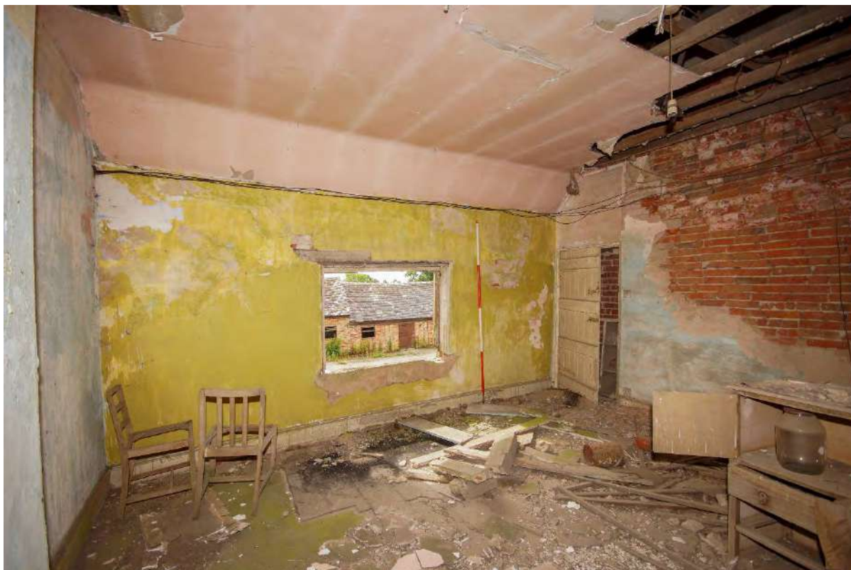
Plate 119: F1 – window opening to the courtyard
