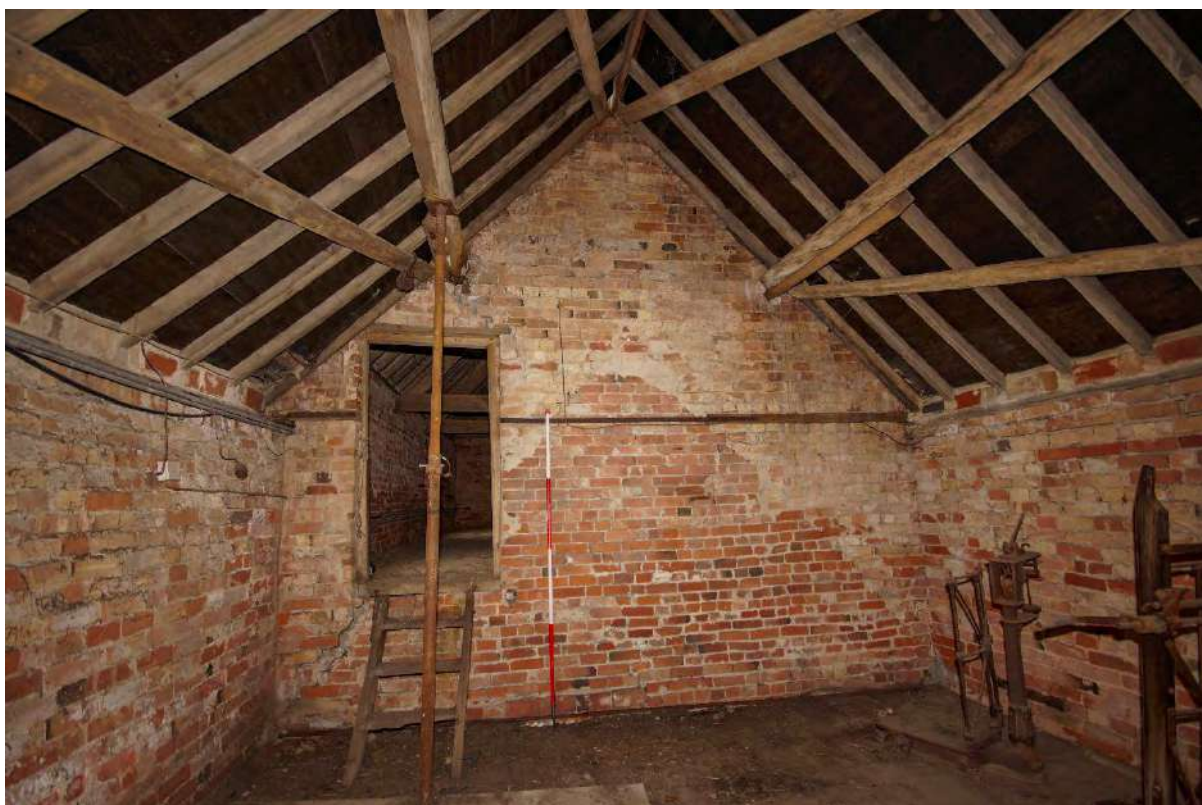
Plate 127: F3 – northwest gable wall with scars of former lower gable
