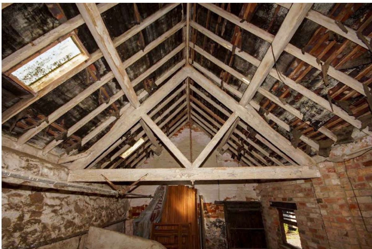
Plate 108: G11 – detail of composite king-bolt truss
