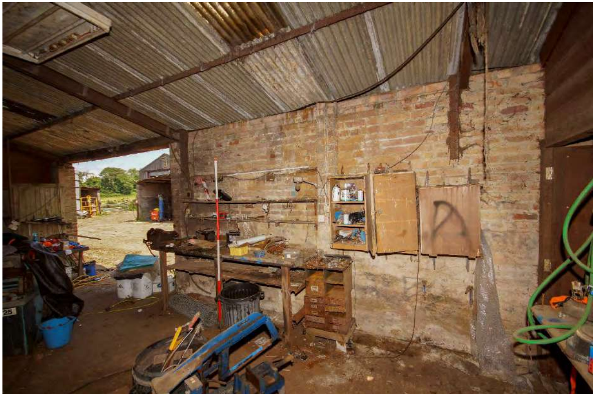
Plate 99: G9 – northeast wall with a large opening to the rear yard
