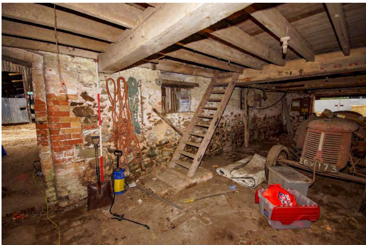
Plate 86: G7 – northeast wall with remains of stone masonry
