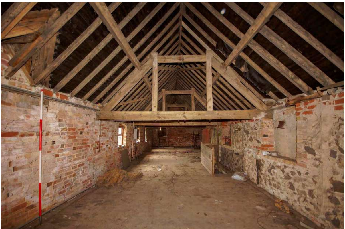
Plate 132: F3 – long first-floor of Building 3 with three queen-post trusses
