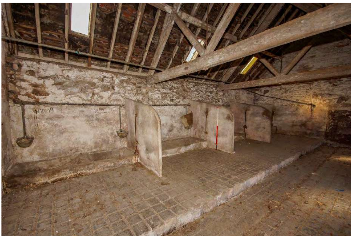
Plate 112: G12 – stone-built southeast wall abutted by concrete stalls
