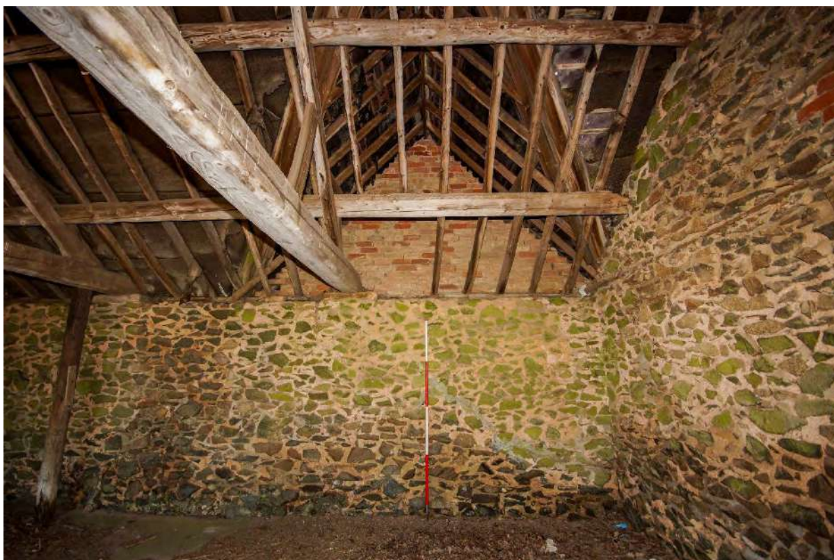
Plate 118: G13 – later brick gable for the roof of the adjacent G12
