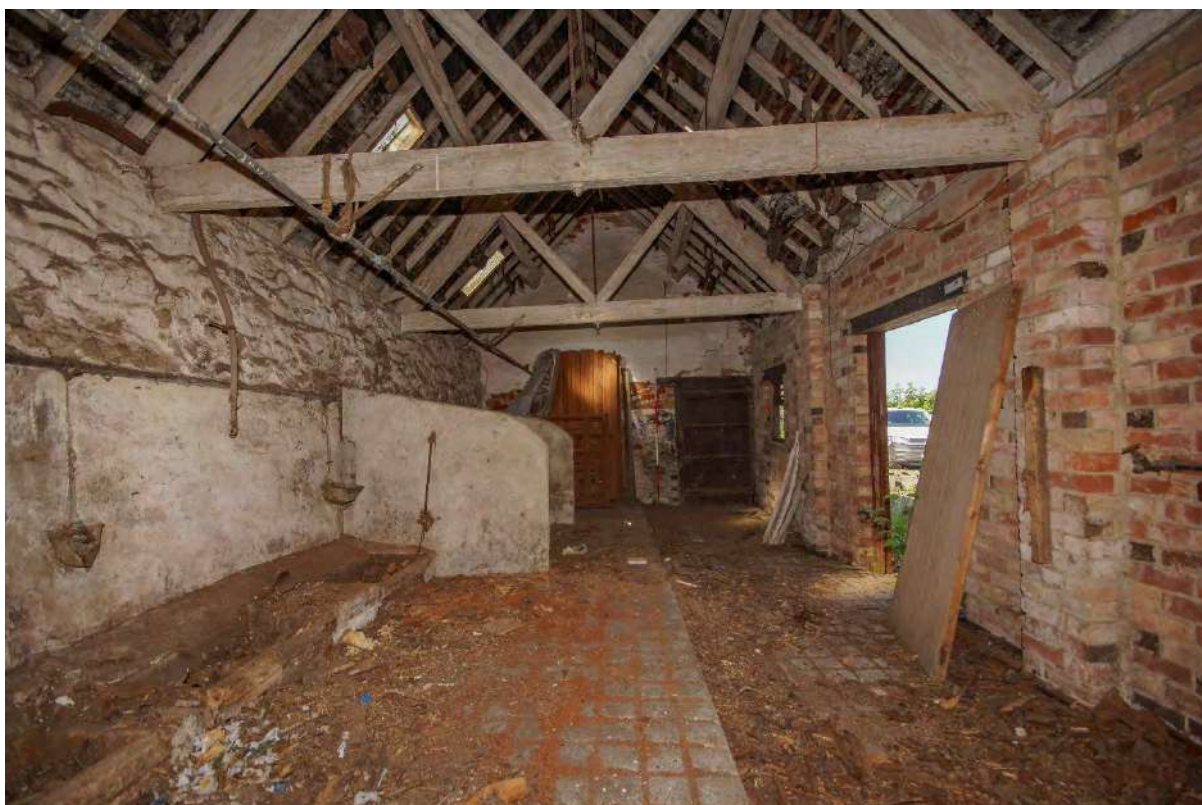
Plate 105: G11 – stone-built southeast wall abutted by concrete boskin and stalls
