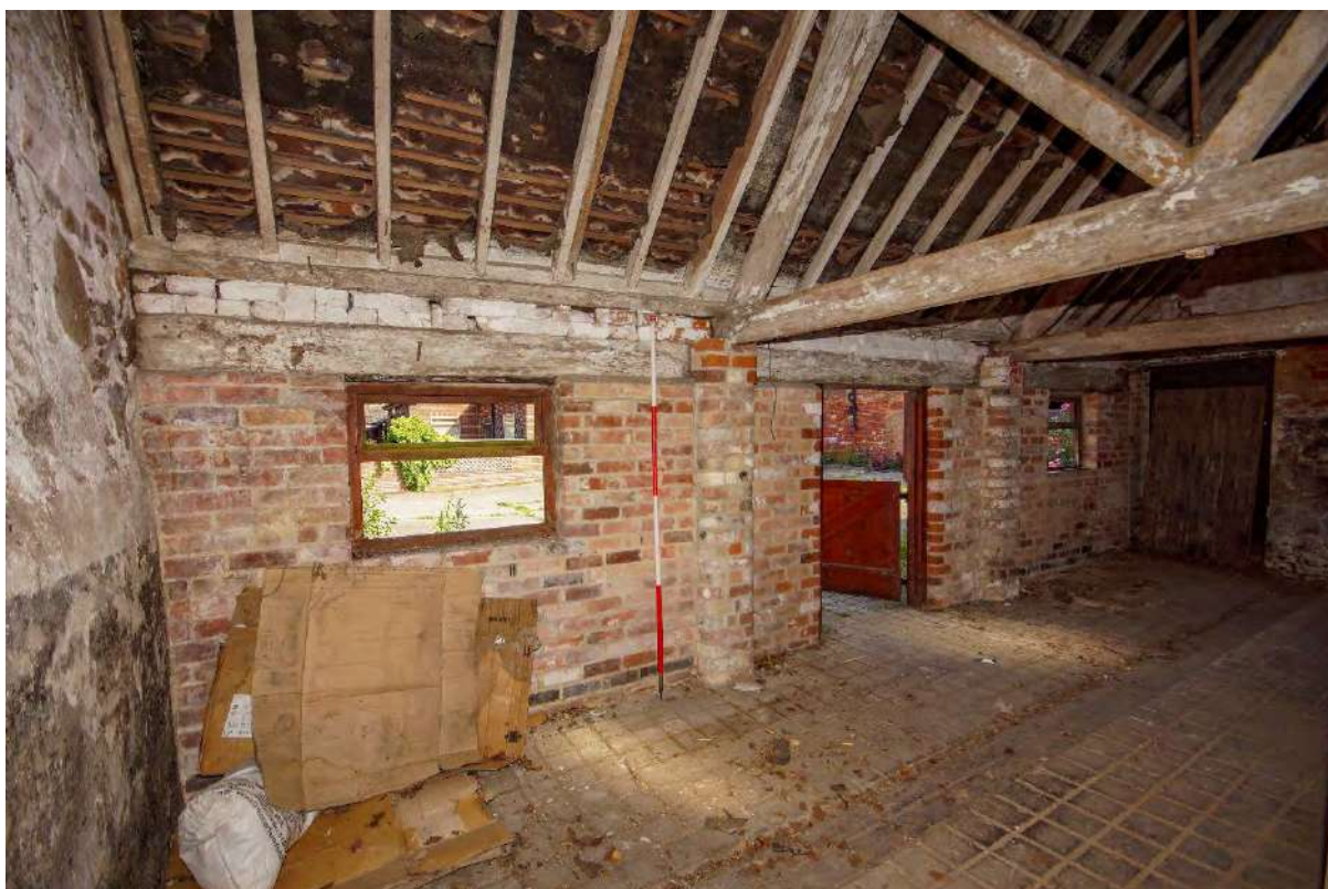
Plate 109: G12 – doorway to the courtyard flanked by infilled brick panels with central window openings
