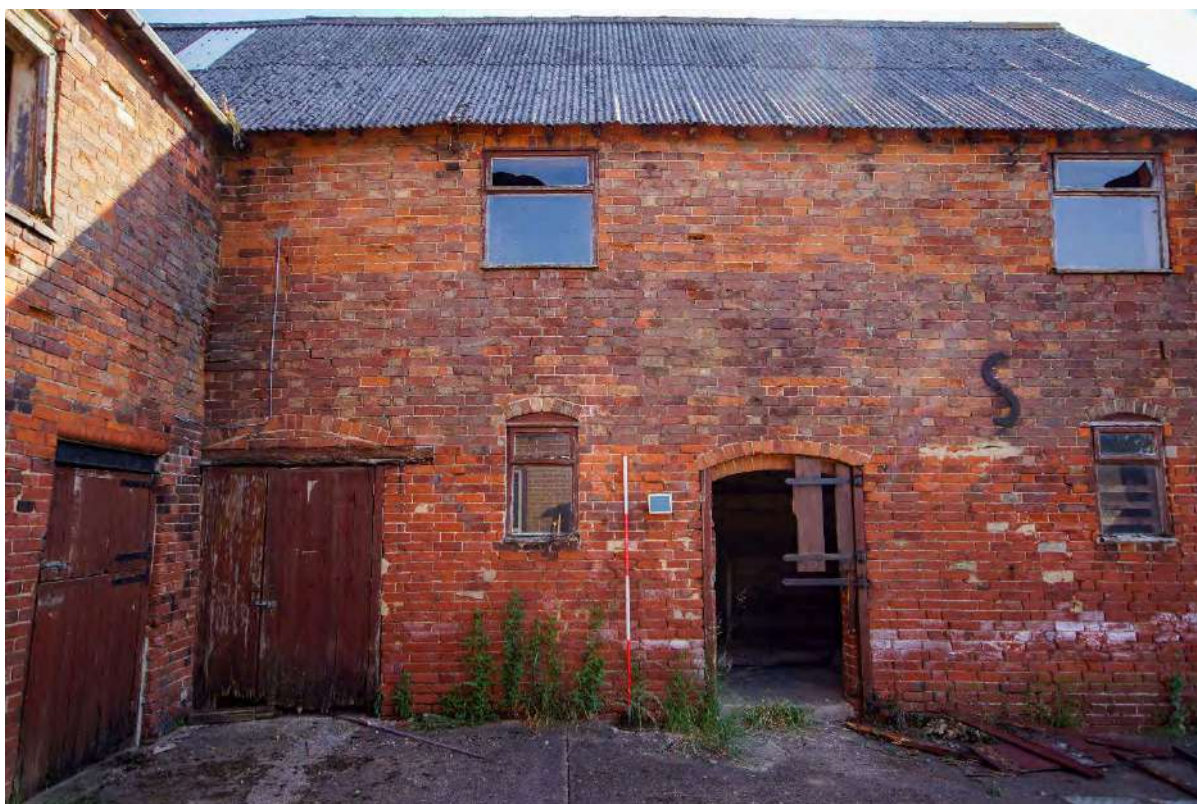
Plate 22: Building 2 – southwest elevation, detail of successive brickwork construction
