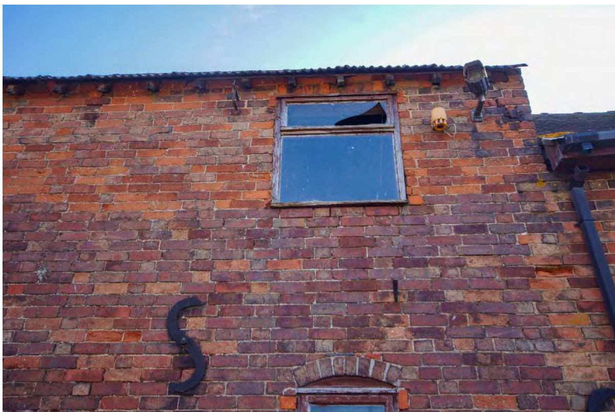
Plate 25: Building 2 – southwest elevation, detail of first-floor window opening
