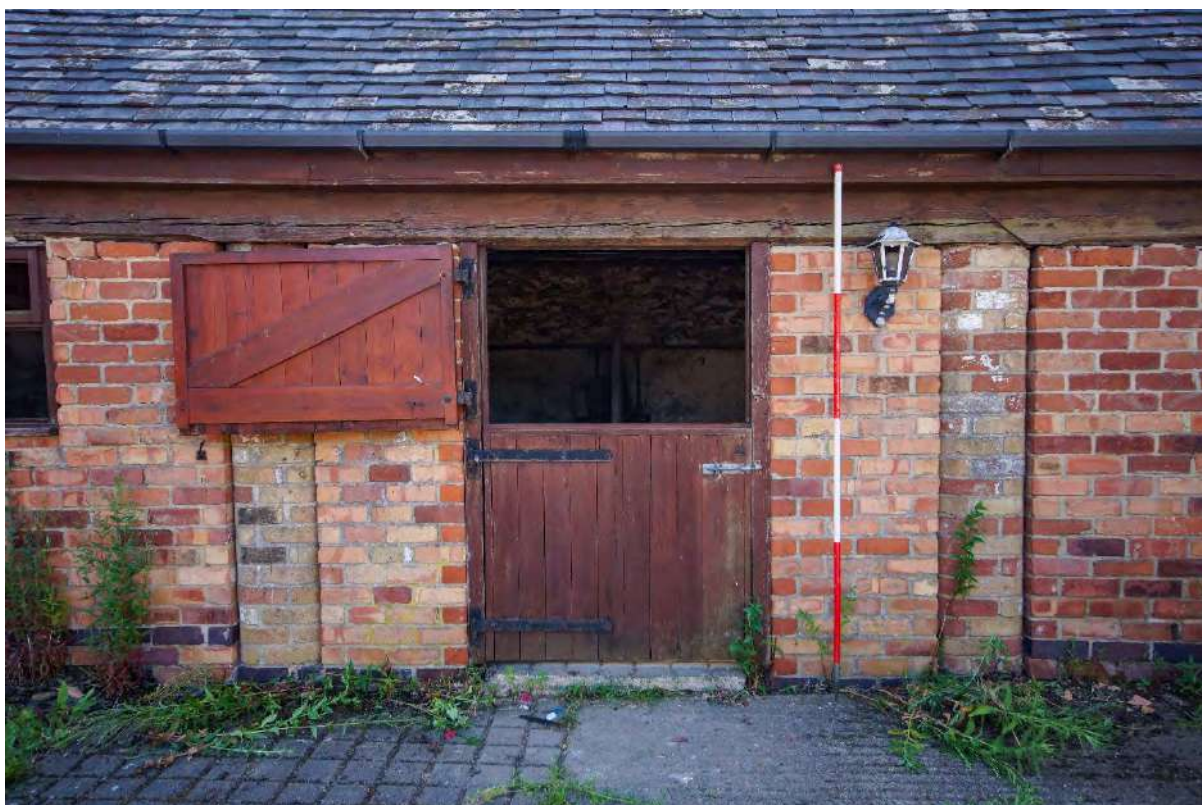
Plate 47: Building 5 – northwest elevation, detail of central doorway
