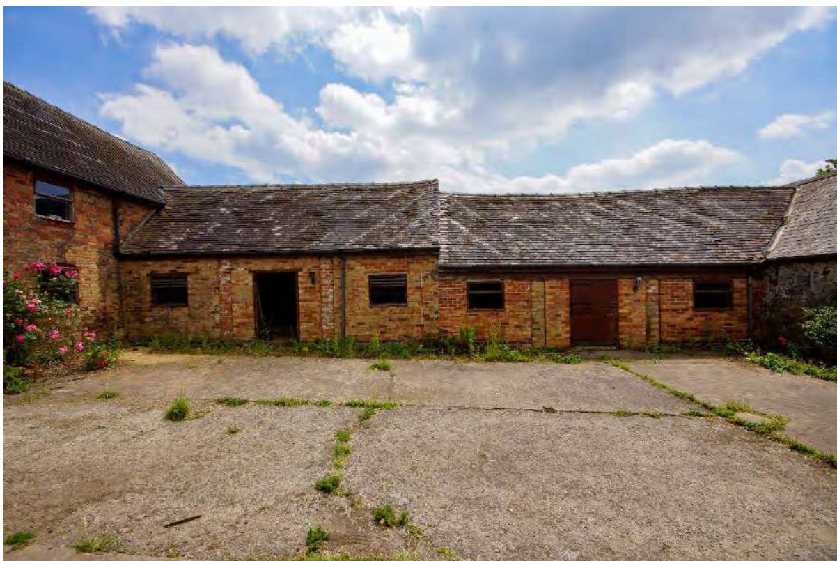
Plate 41: Building 4 – northwest elevation with contiguous Building 5 to the right
