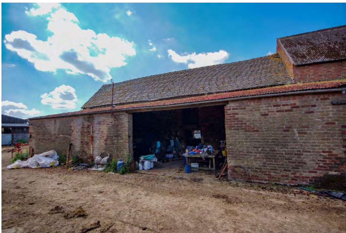
Plate 38: Building 3 – northeast elevation with lean-to extension
