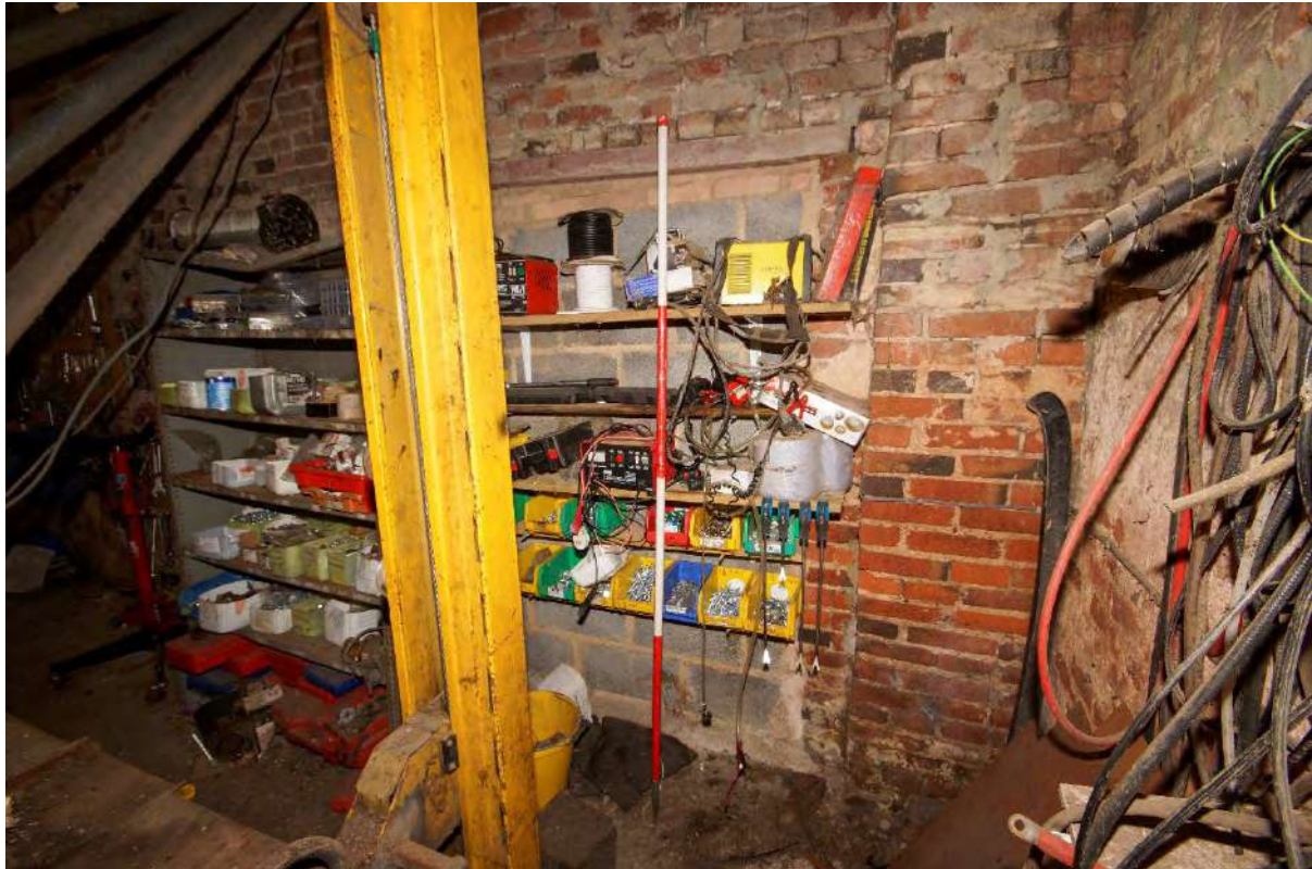
Plate 63: G2 – later doorway blocked with concrete blockwork
