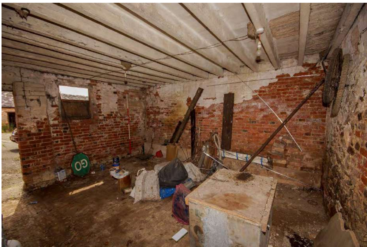
Plate 57: G1 – southeast wall with doorway and window opening
