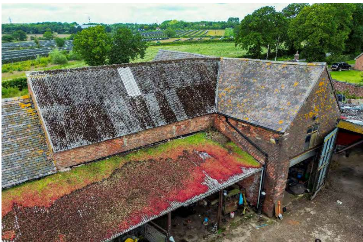
Plate 19: Building 2 – aerial view of the northeast elevation with a later open-fronted lean-to extension
