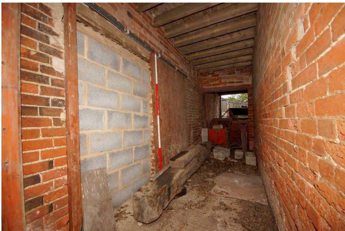
Plate 70: G3 – blocked doorway to G2
