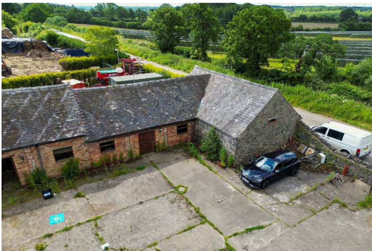
Plate 52: Building 6 – aerial view with cross wing Building 5 to the left
