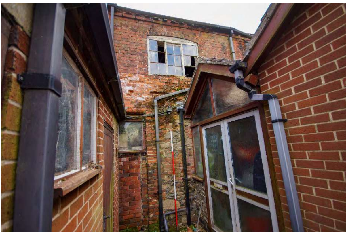
Plate 14: Building 1 – northwest elevation, remains of stone masonry and blocked doorway
