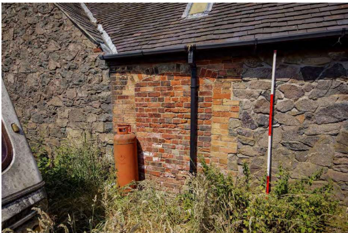
Plate 51: Building 5 – southeast elevation, blocked doorway to the southwest end
