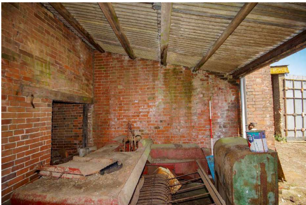
Plate 77: G5 – arched doorway to passage G3
