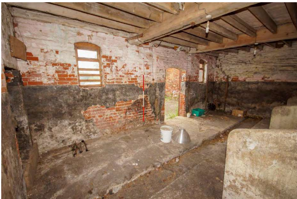
Plate 73: G4 – doorway to the courtyard
