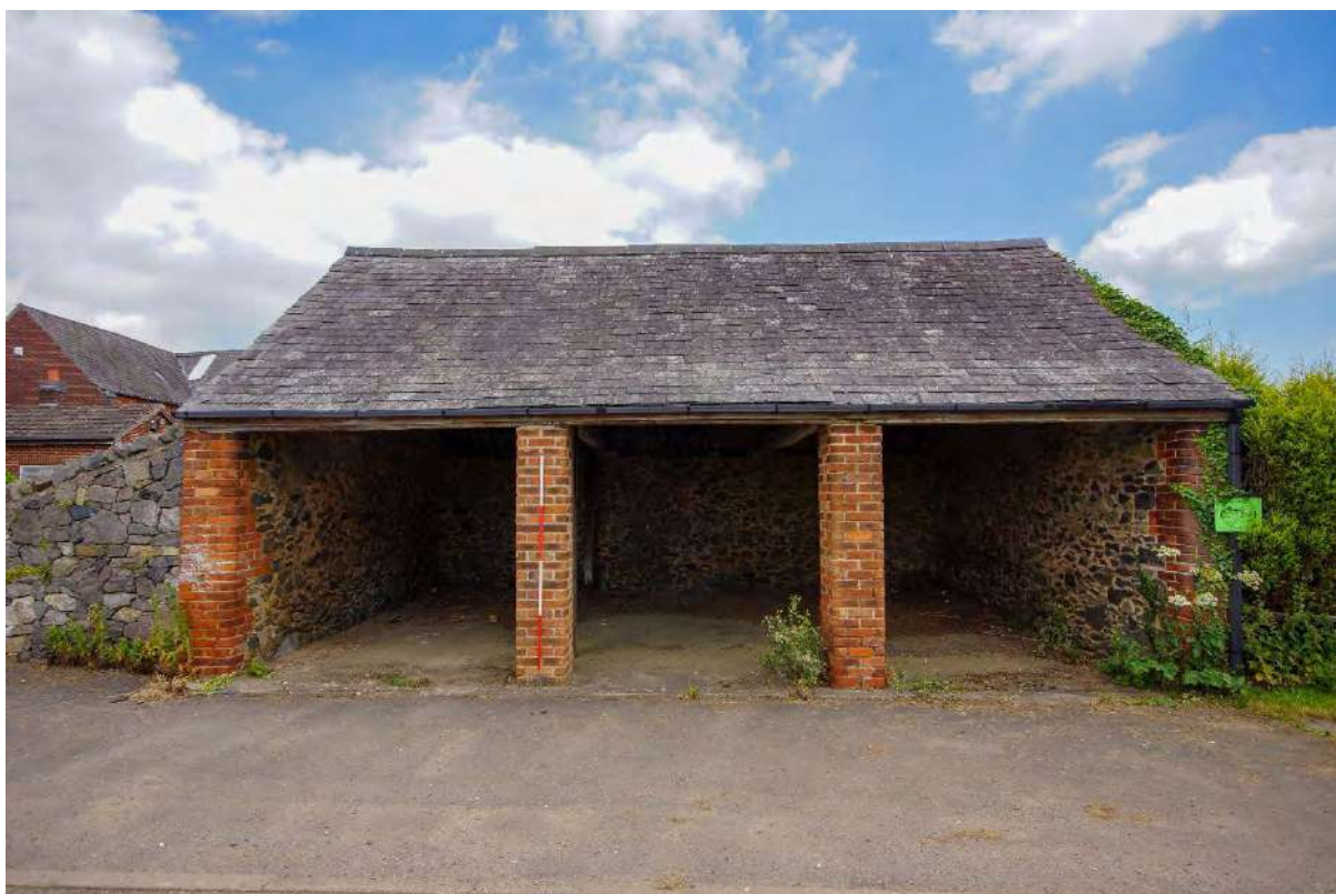
Plate 53: Building 6 – southwest open-fronted elevation
