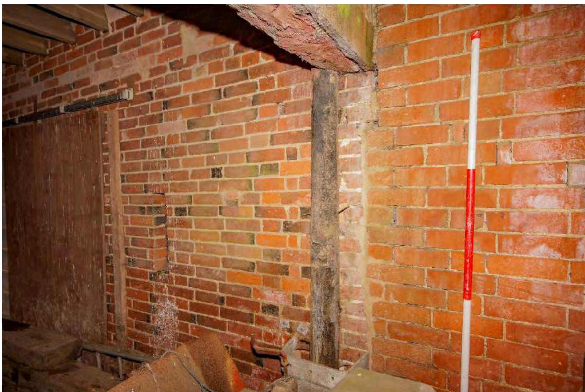
Plate 72: G3 – northwest doorway and construction joint
