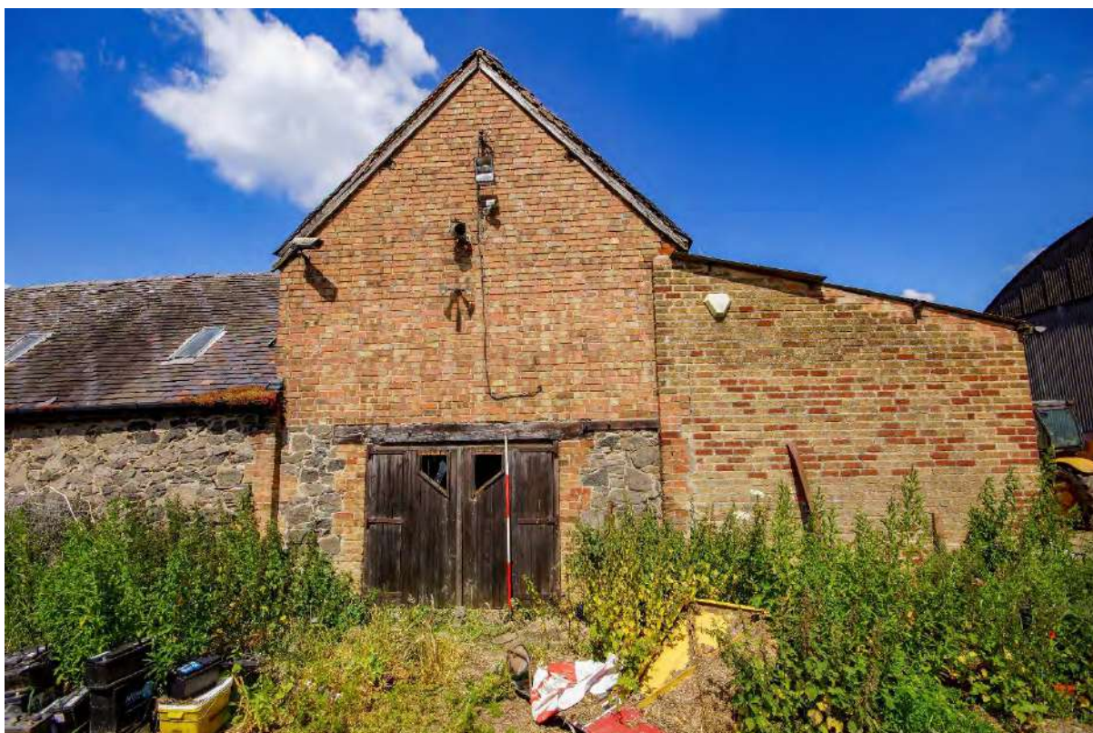
Plate 36: Building 3 – southeast elevation
