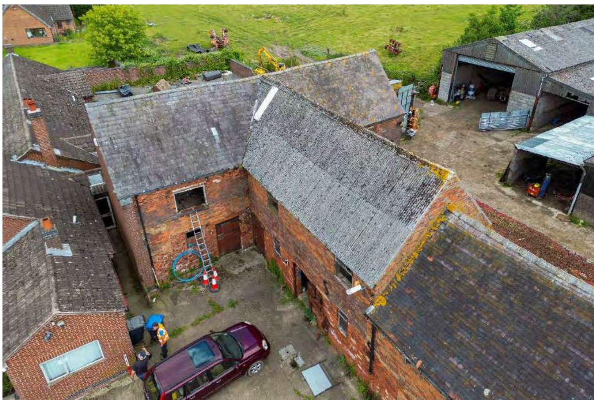
Plate 7: Building 1 – aerial view of the southeast elevation with cross-wing Building 2
