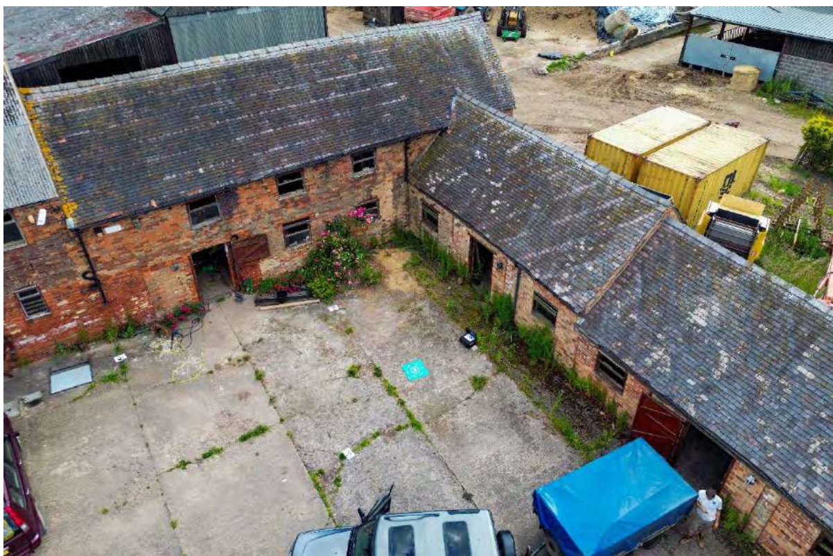
Plate 28: Building 3 – aerial view of the southwest elevation abutted by Building 4 to the right
