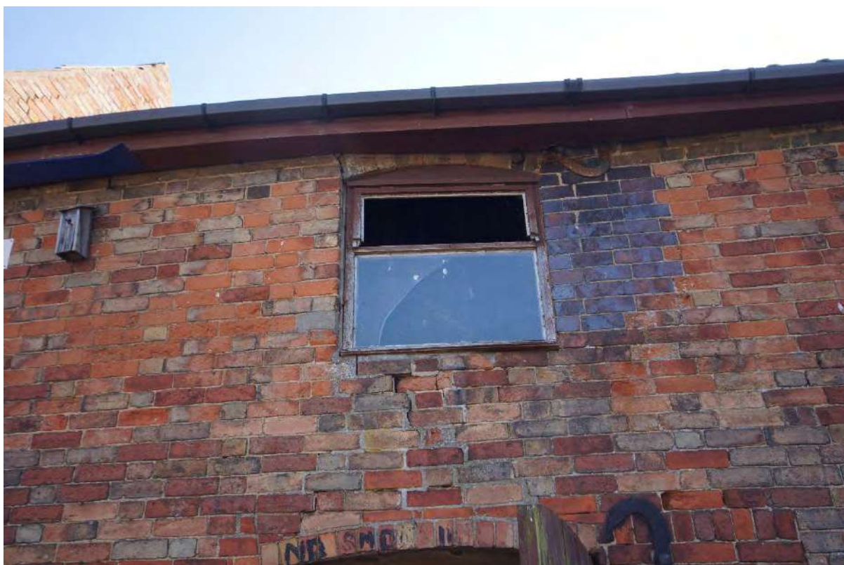
Plate 35: Building 3 – southwest elevation, detail of first-floor window opening
