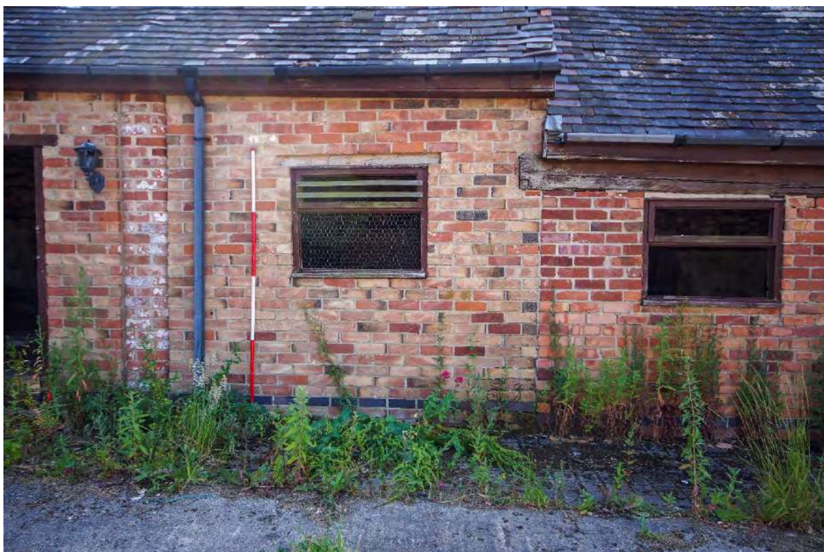
Plate 43: Building 4 – northwest elevation, detail of construction joint to Building 5
