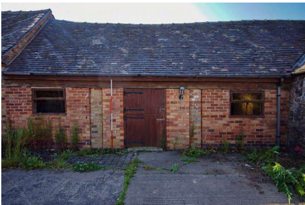
Plate 46: Building 5 – northwest elevation
