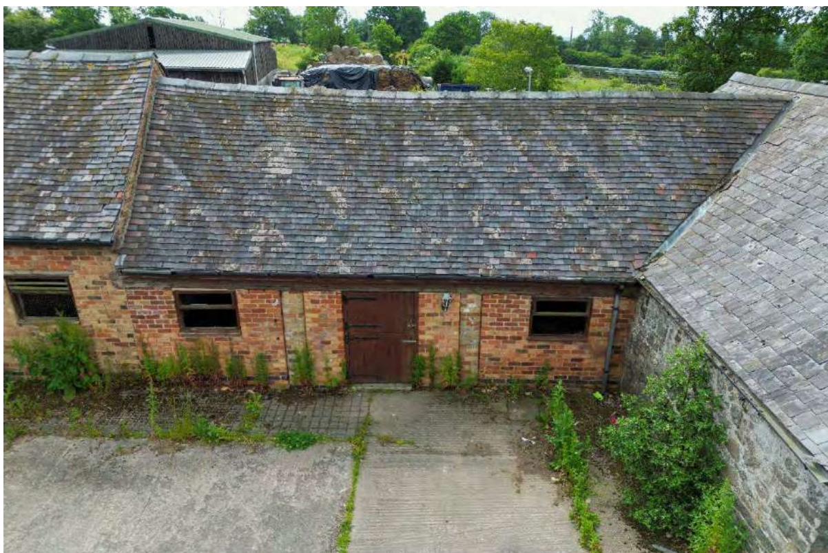
Plate 45: Building 5 – aerial view of the northwest elevation
