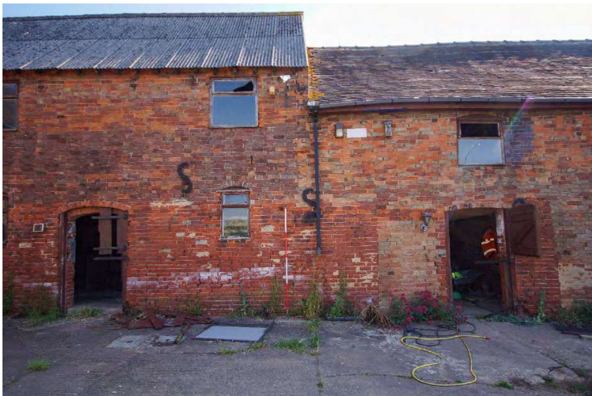
Plate 21: Building 2 – southwest elevation, detail of staggered construction joints
