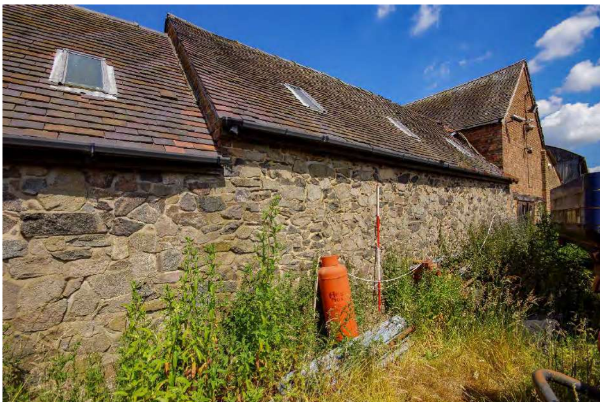
Plate 44: Building 4 – southeast elevation
