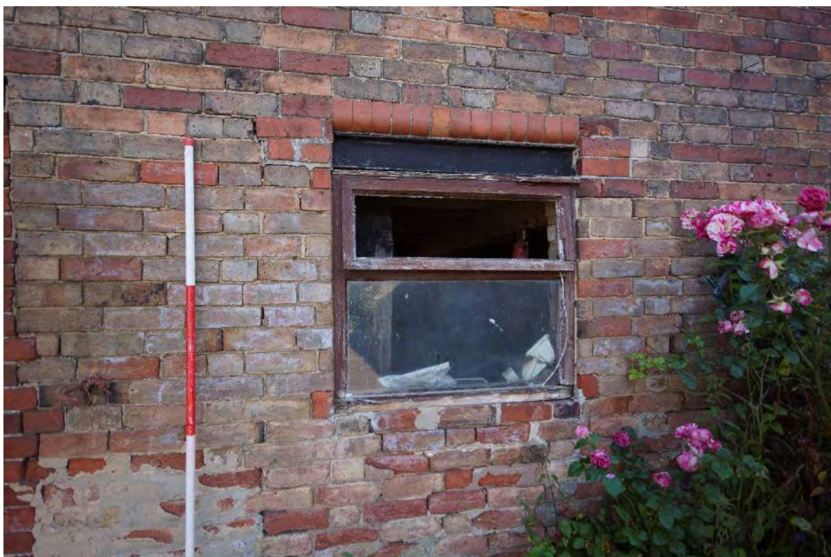
Plate 33: Building 3 – southwest elevation, inserted ground-floor window opening
