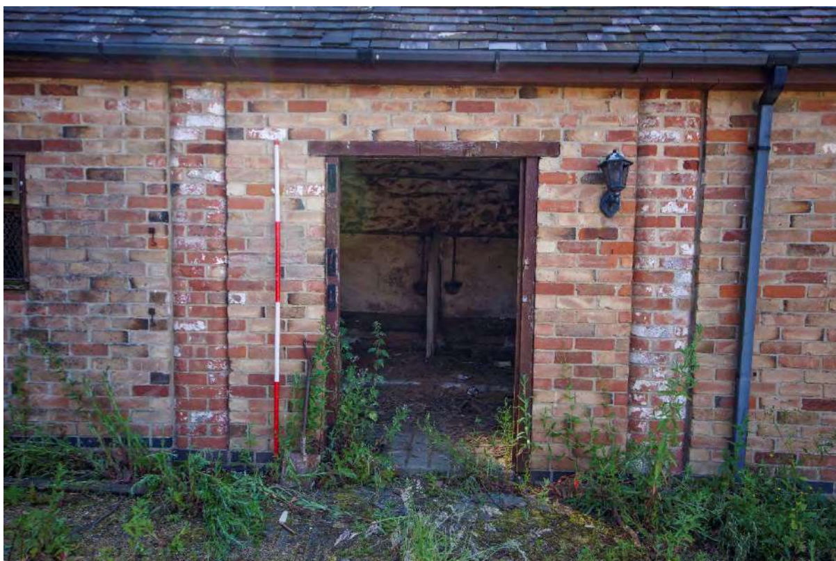
Plate 42: Building 4 – northwest elevation, detail of central doorway
