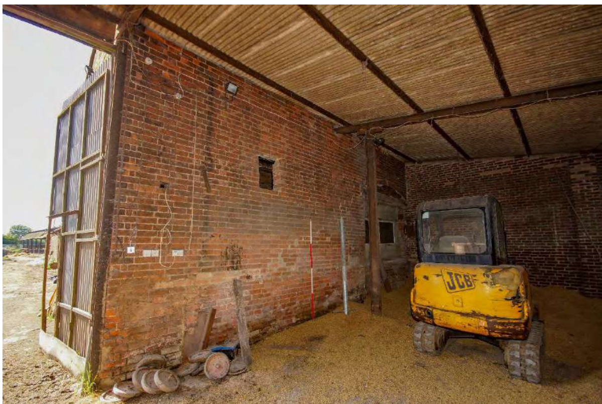
Plate 15: Building 1 – northwest elevation viewed from inside a later store
