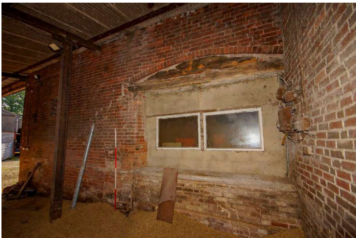
Plate 17: Building 1 – northwest elevation with blocked arched doorway
