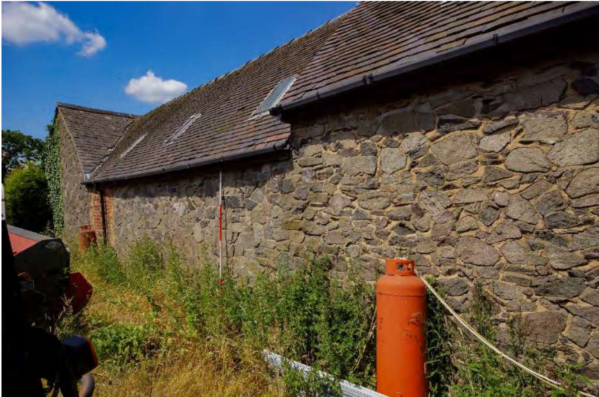
Plate 49: Building 5 – southeast elevation with contiguous Building 4 to the right
