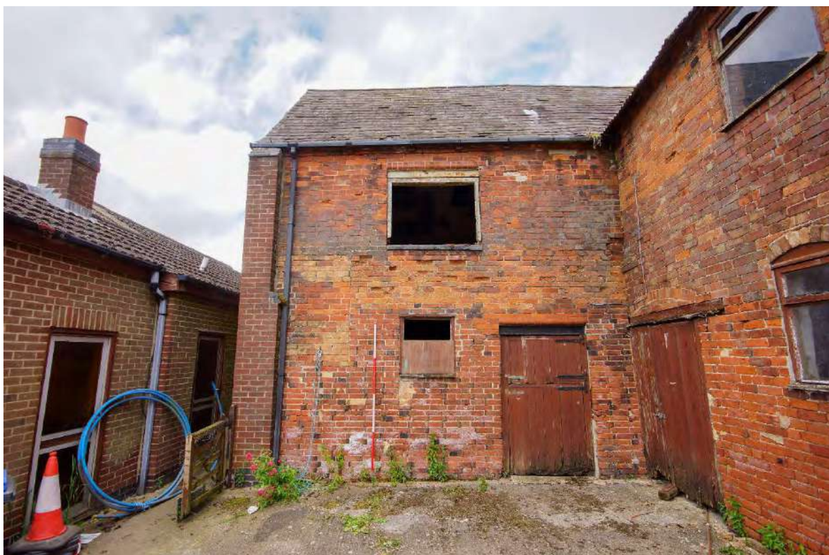
Plate 9: Building 1 – southeast elevation
