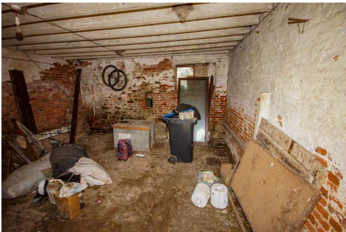
Plate 59: G1 – northwest wall with remains of stone masonry
