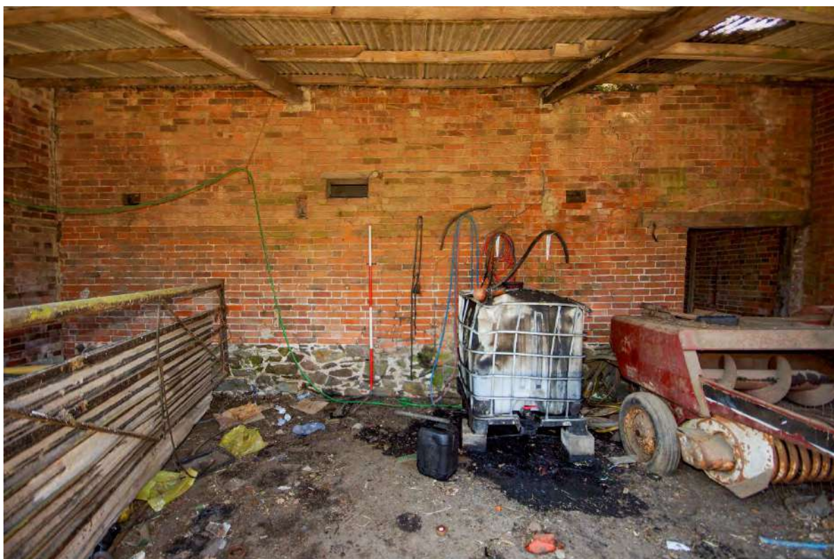
Plate 78: G5 – northeast wall with lower stone masonry
