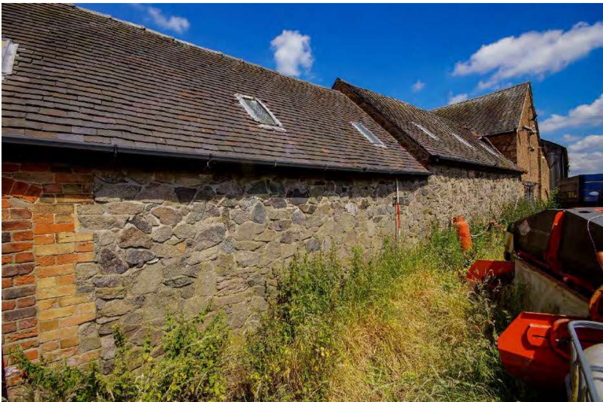
Plate 50: Building 5 – southeast elevation
