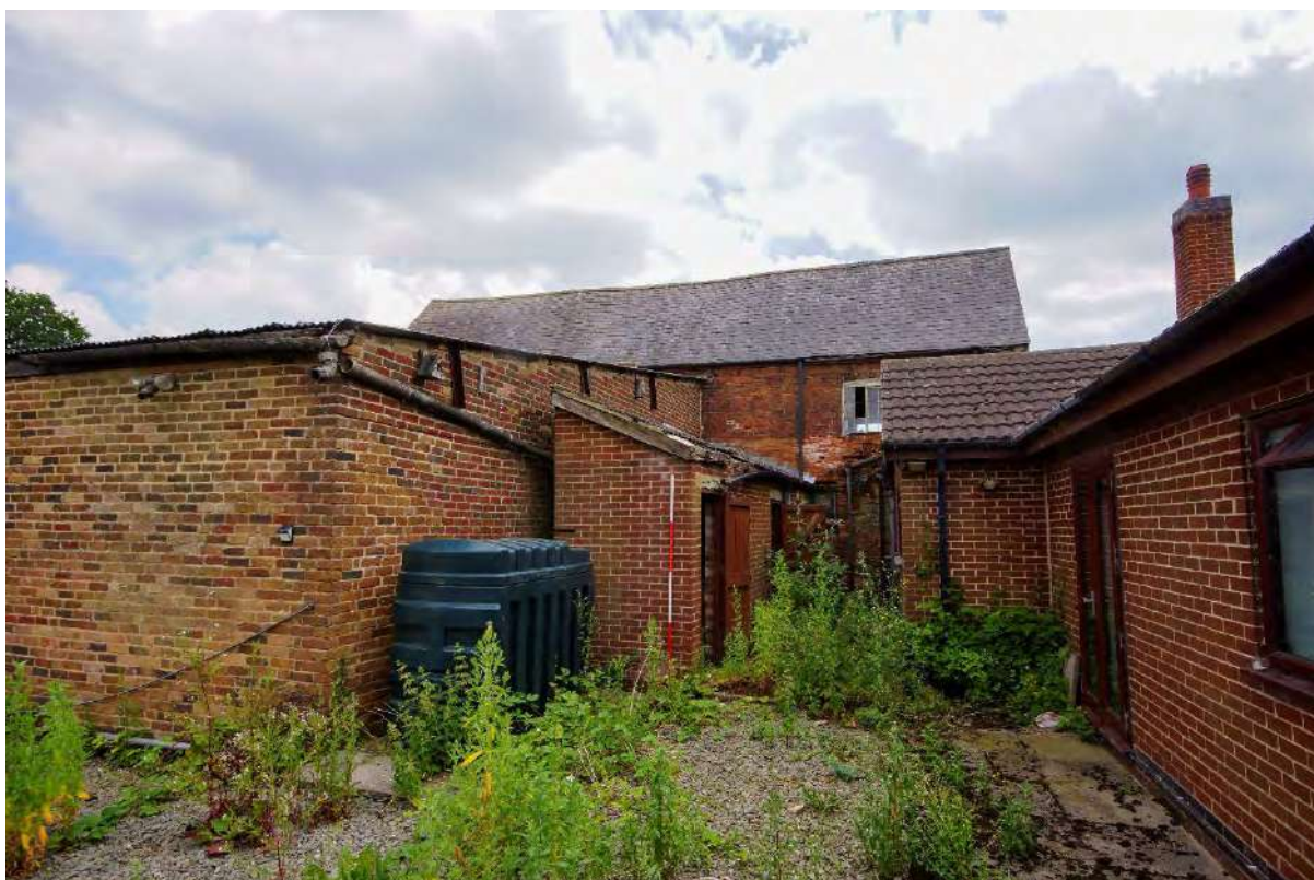
Plate 13: Building 1 – northwest elevation
