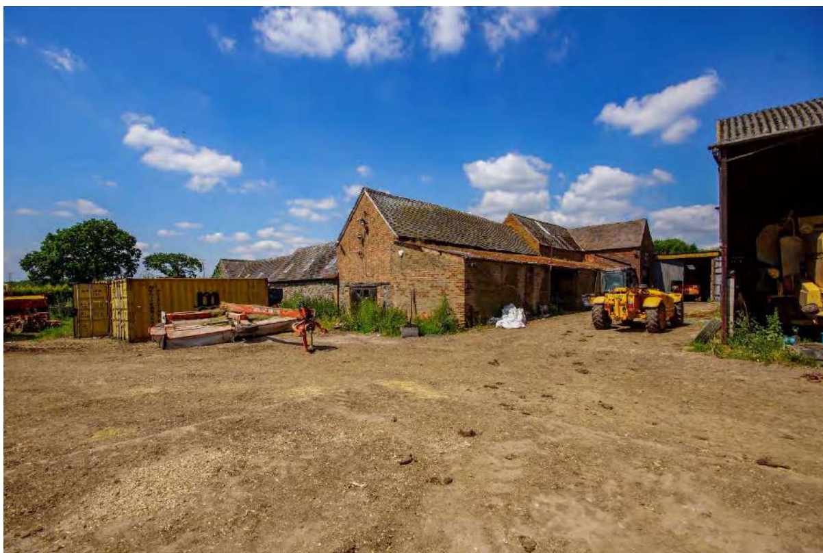
Plate 30: Building 3 – general view to the rear side with later lean-to extension
