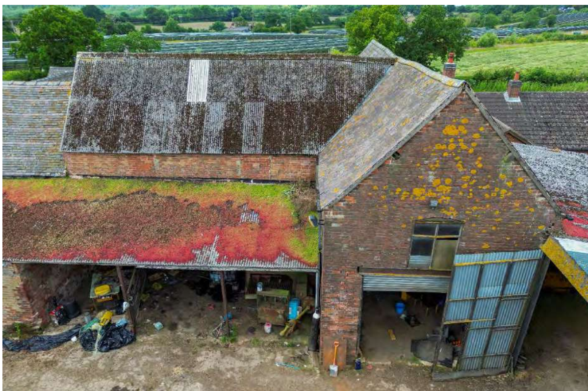
Plate 8: Building 1 – aerial view of the northeast gable and adjacent Building 2
