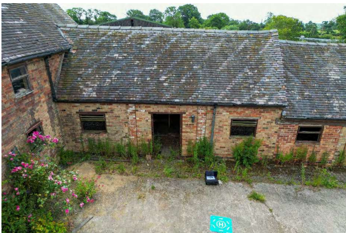
Plate 40: Building 4 – aerial view of the northwest elevation
