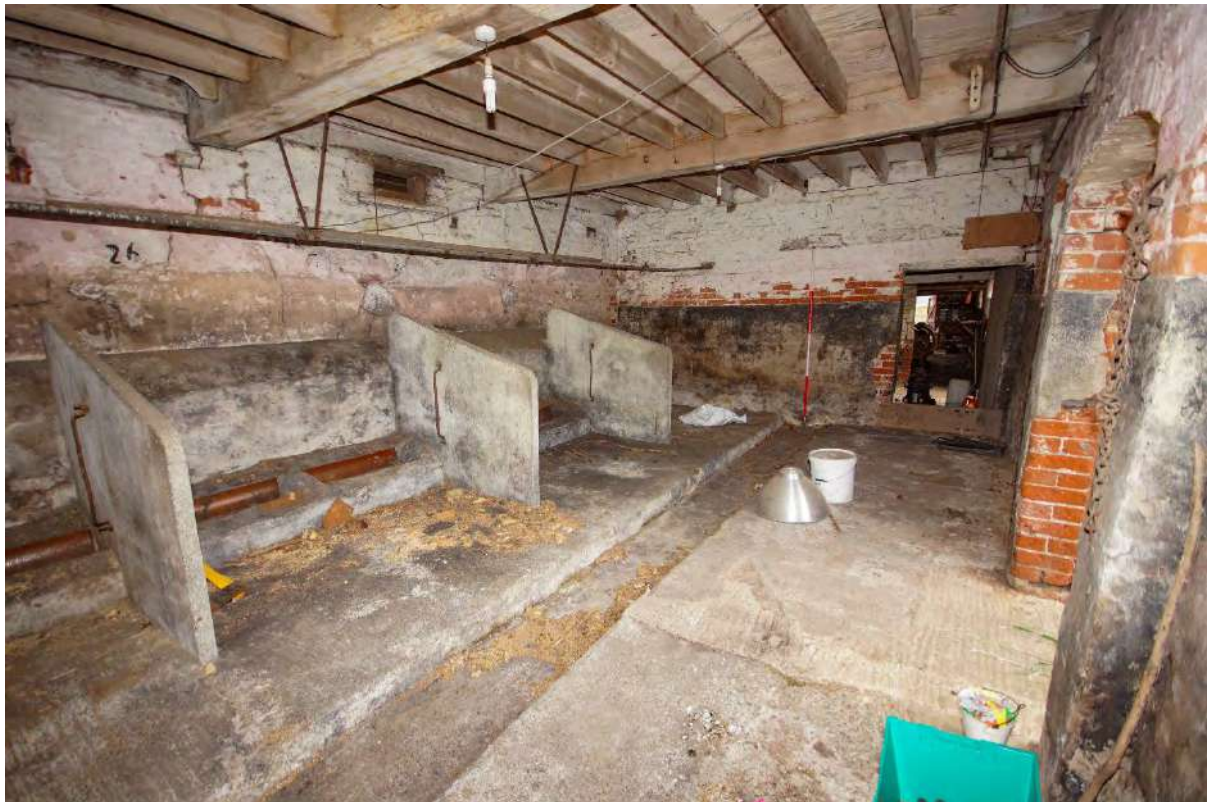
Plate 75: G4 – concrete boskin with drainage gully
