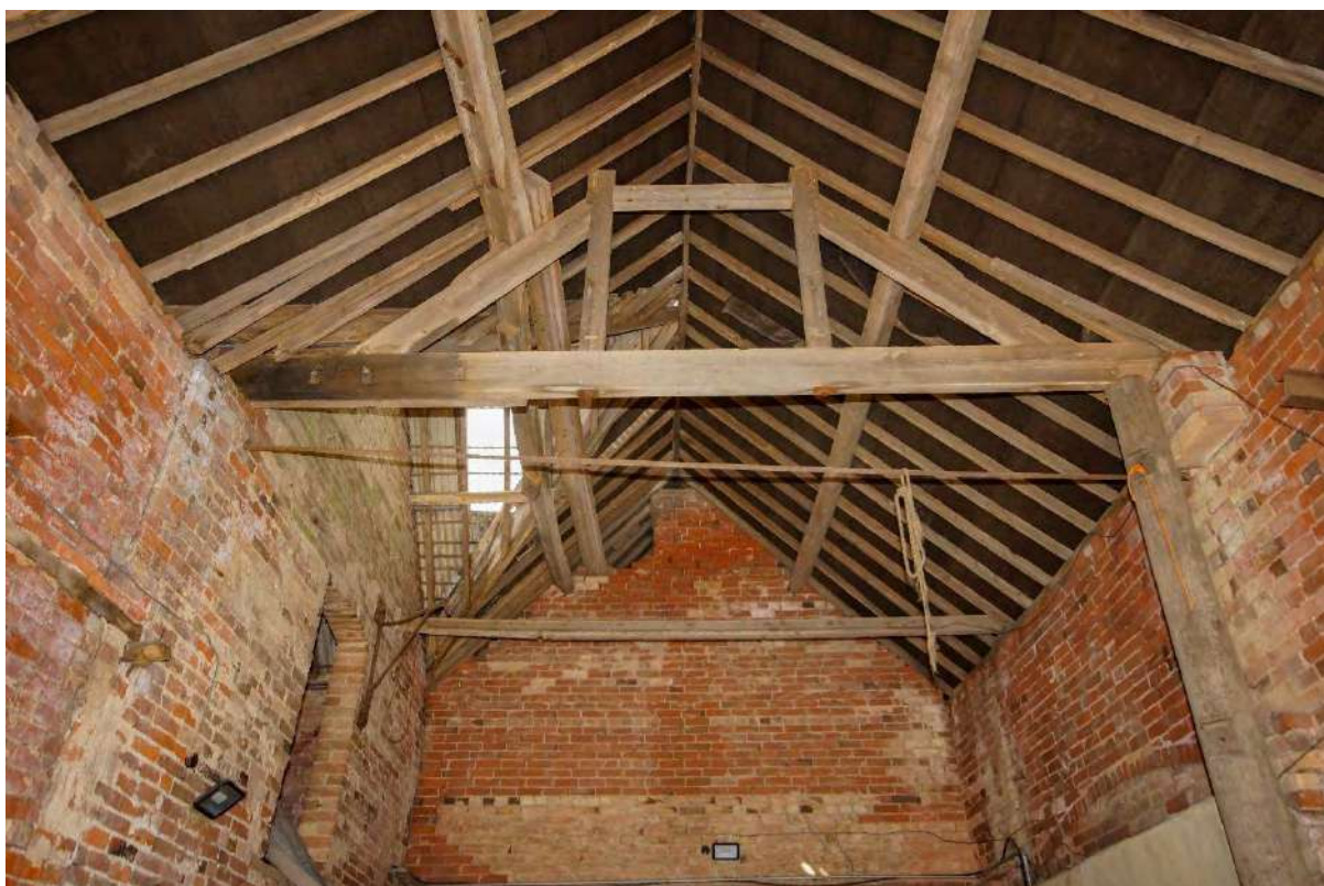
Plate 65: G2 – detail of queen-post truss
