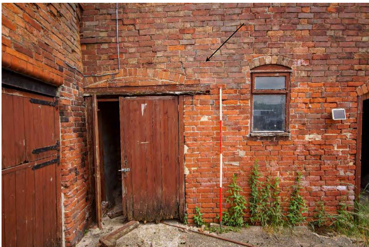
Plate 24: Building 2 – southwest elevation, doorway to the northwest and incised graffiti '1861' (arrow)
