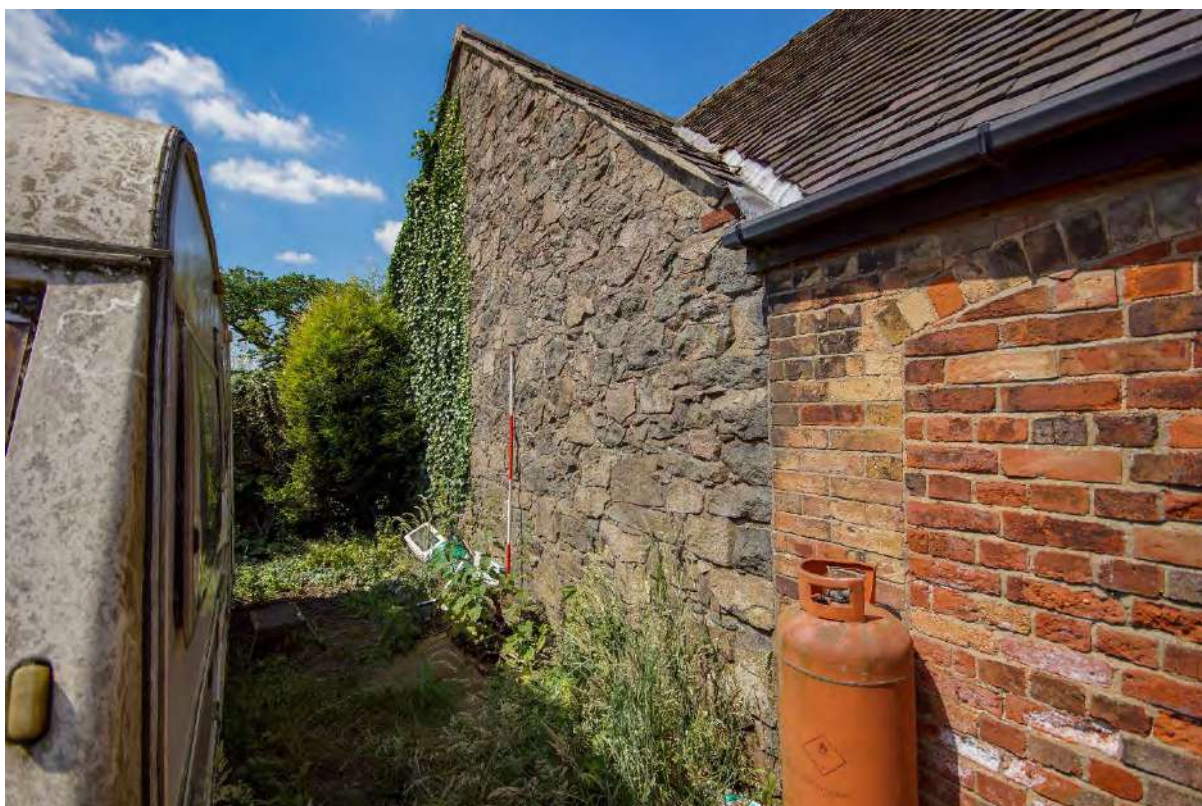
Plate 56: Building 6 – southeast gable elevation
