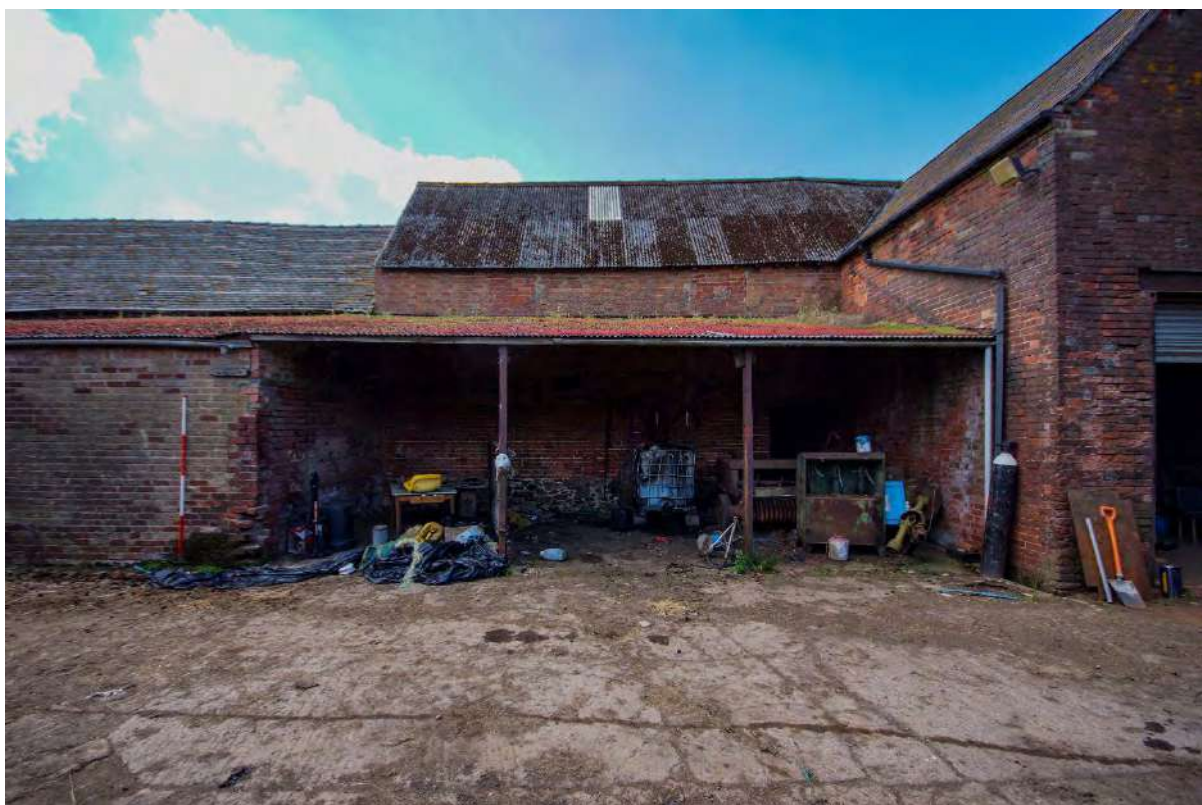
Plate 27: Building 2 – northeast elevation, leant-to extension and blocked first-floor window openings
