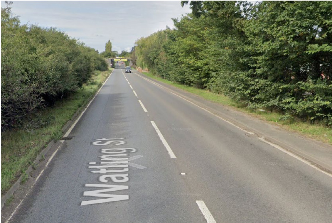
Photograph 3.2: View North West on The A5 from the Site Frontage
