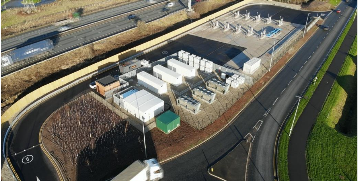
Figure 2. Existing CNG Fuels Station (Warrington)
