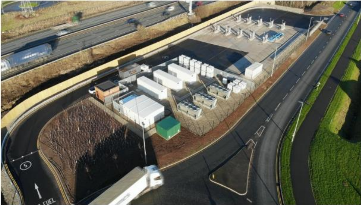
Figure 1. Example aerial photograph of existing CNG Fuelling Station at Warrington
