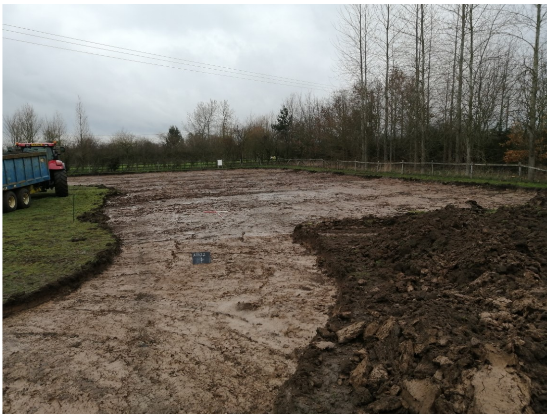
Plate 5; new access road, View northeast.
