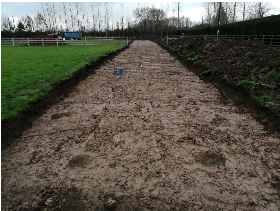
Plate 6; new access road, view east
