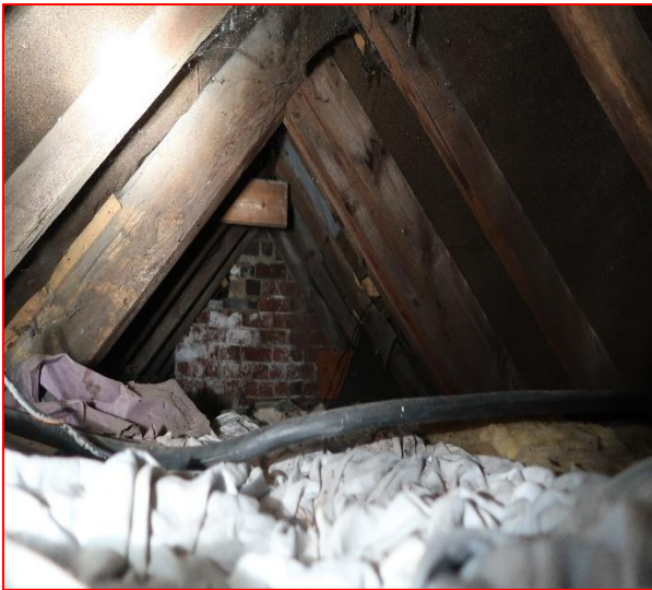
Internal view of roof space
