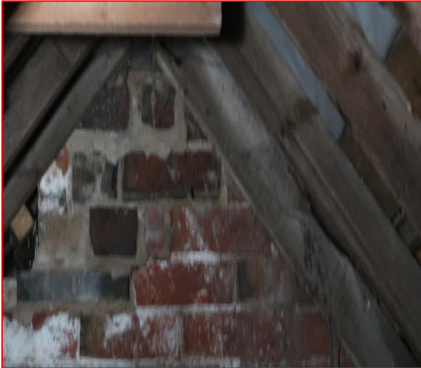
Internal view of roof space
