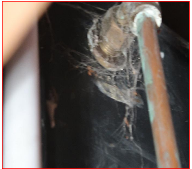
View of roof space
