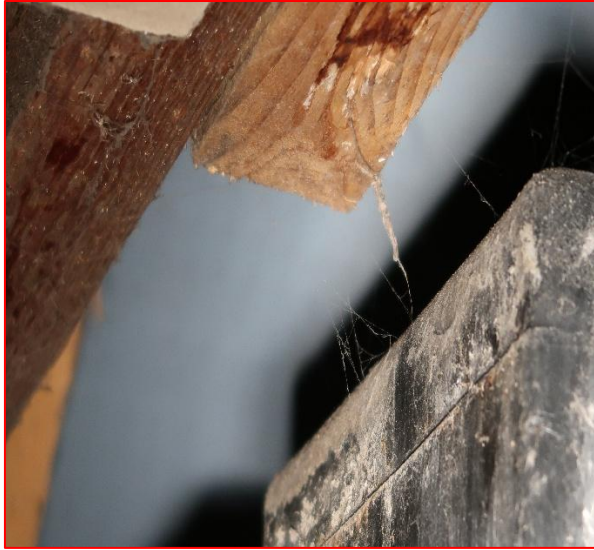
Internal view of roof space
