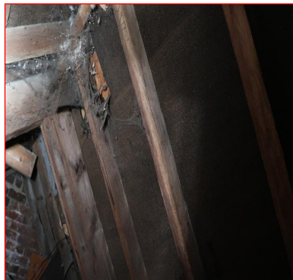
Internal view of roof space
