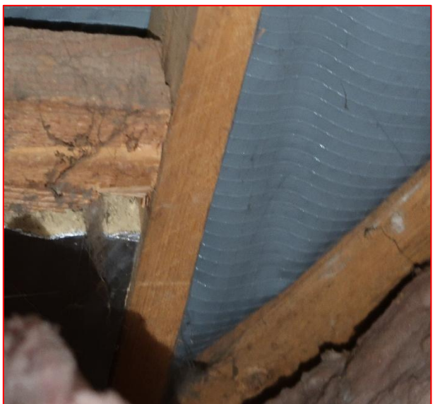
Internal view of roof space
