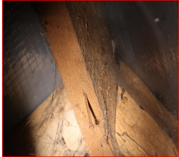
Internal view of roof space
