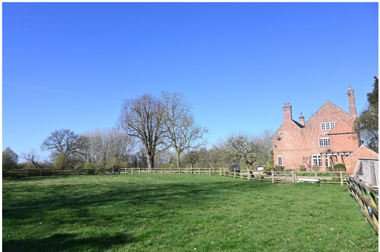
Fig. 9 View of the Old House from the Brick Stable
