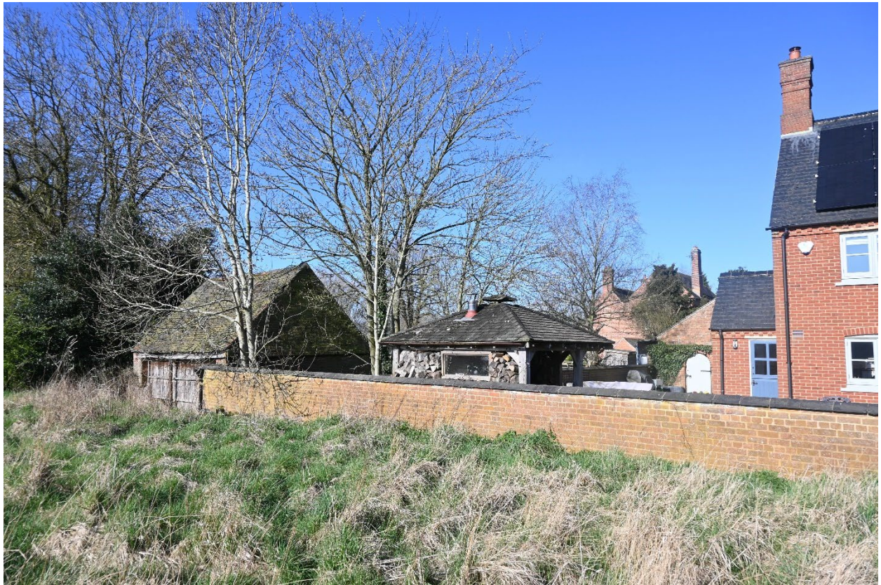
Fig. 8 Brick Stable, Boundary wall and Neighbouring dwelling - Field View
