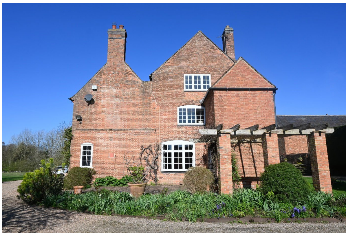
Fig. 3 The Old House side Elevation
