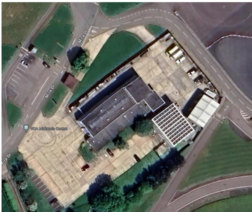
Existing site aerial.
