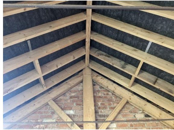
Figure 6- Rafters and membrane
