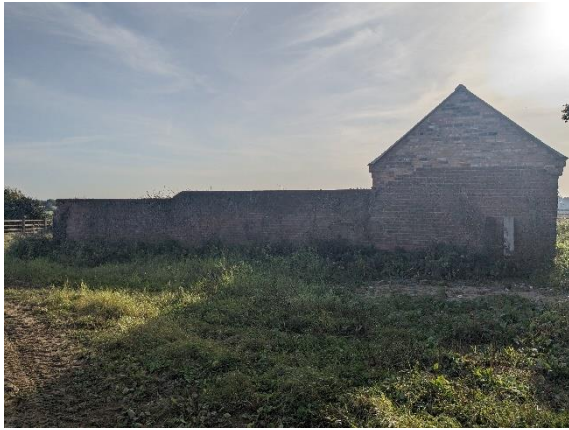
Figure 9- Courtyard wall in good condition
