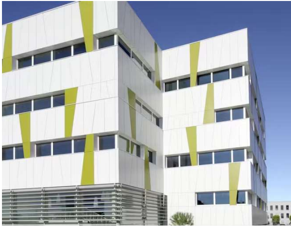
Figure 4 - Rockpanel Cladding shown in situ.
