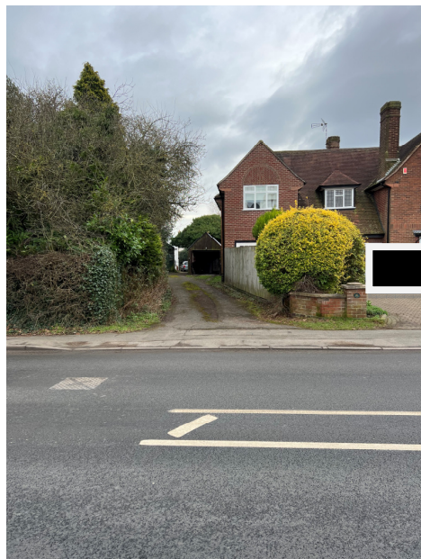
Entrance to 'shared driveway' from main rd.
