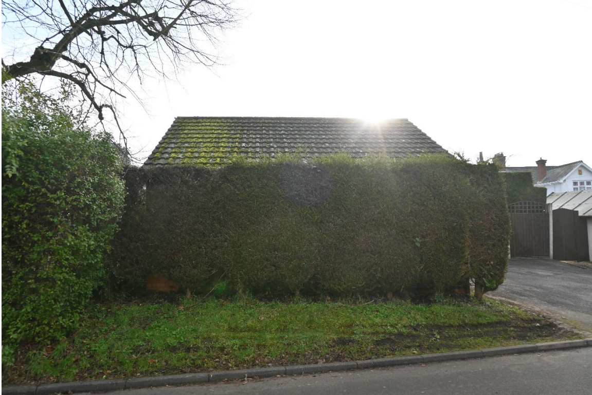
Fig 2. Street view of Garage from Victoria Road
