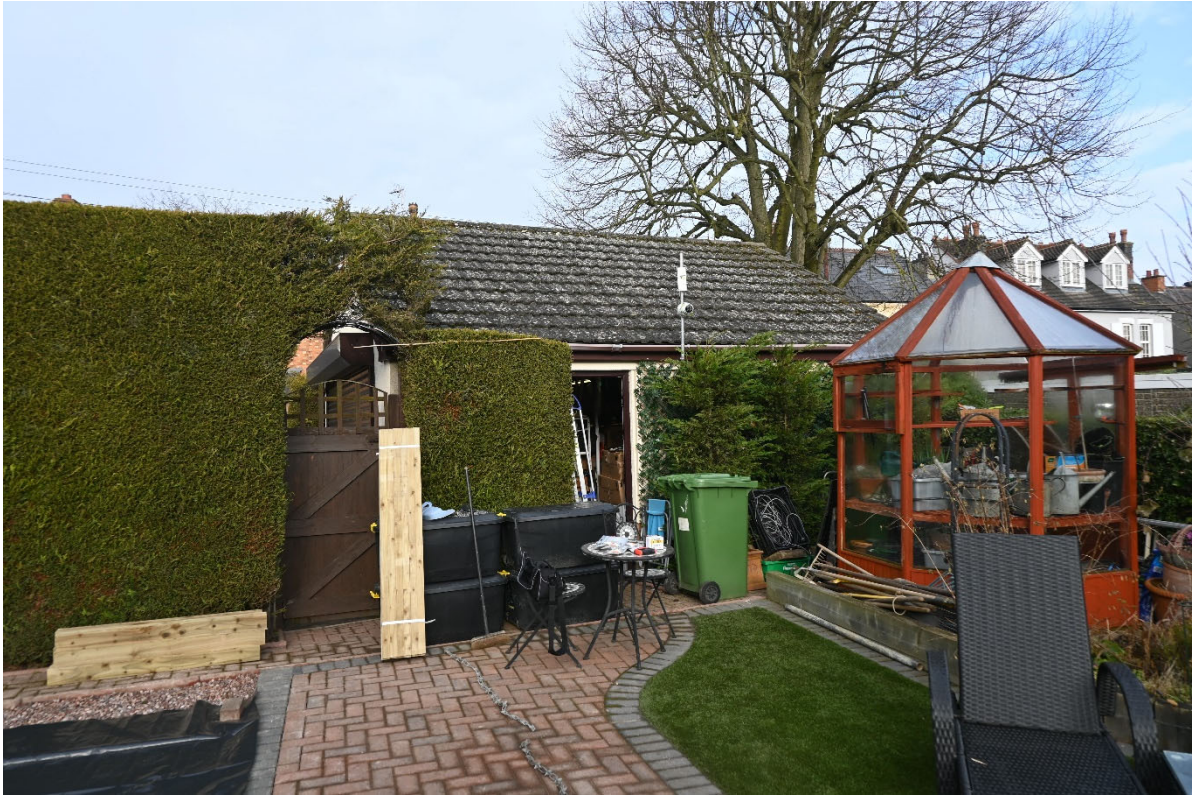
Fig 4. Rear view of Garage from Garden
