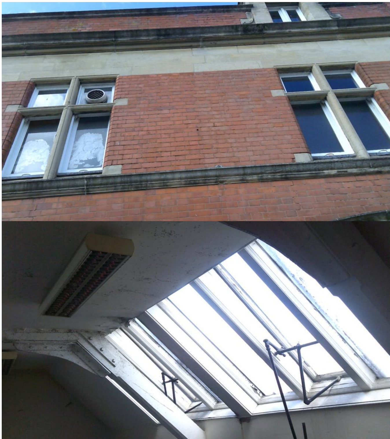
Internal 3 rd storey showing small loft (inaccessible)
