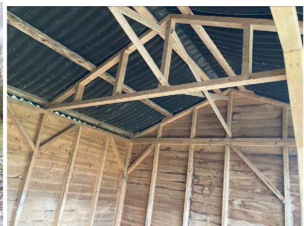
Interior of Horse Shelter
