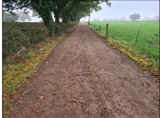
Photograph 2: hardstanding roadway in the east of the Site.
