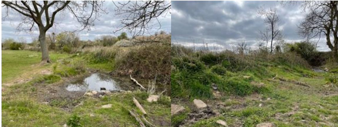
Existing pond looking north
