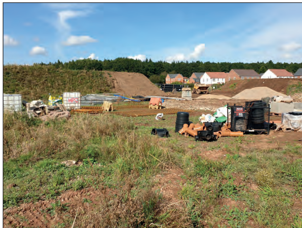
Site (southern field), looking north
