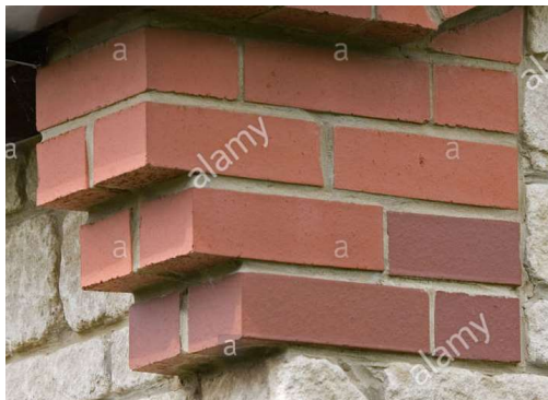
(Left) Corbel brickwork detail material key '13', (Middle) Render and brick, (Right) Soldier bond head detail.
