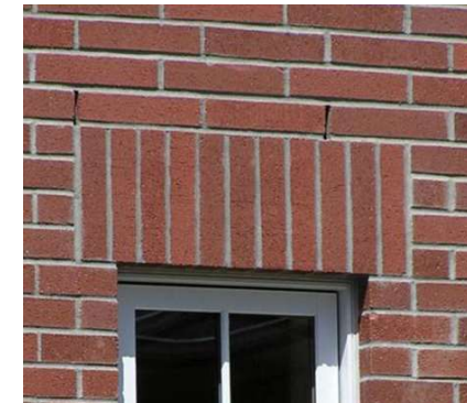
(Left) Corbel brickwork detail material key '13', (Middle) Render and brick, (Right) Soldier bond head detail.
