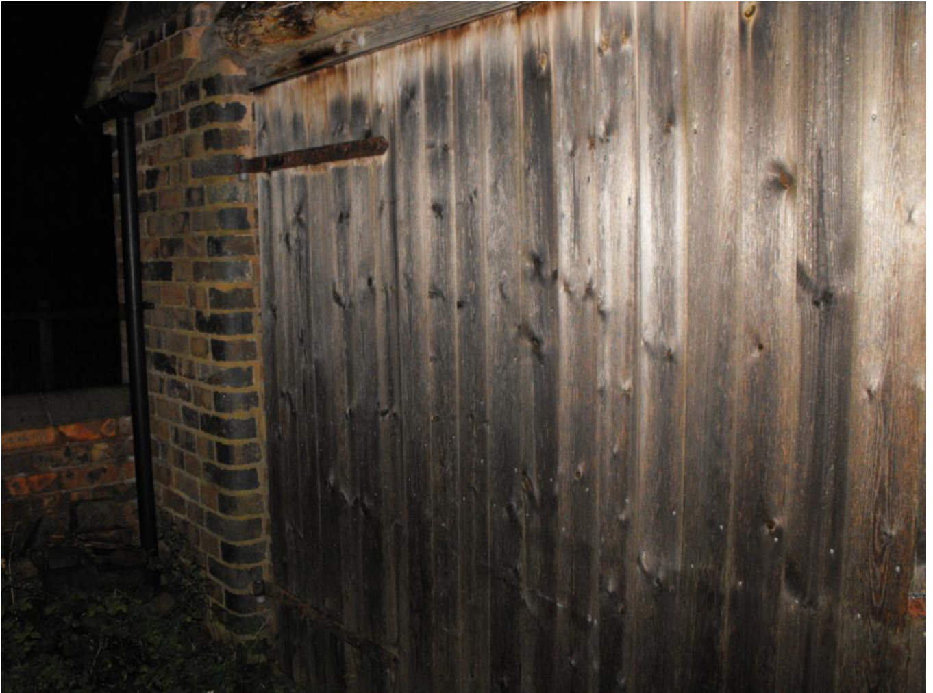
External doorway (tight fitting)
