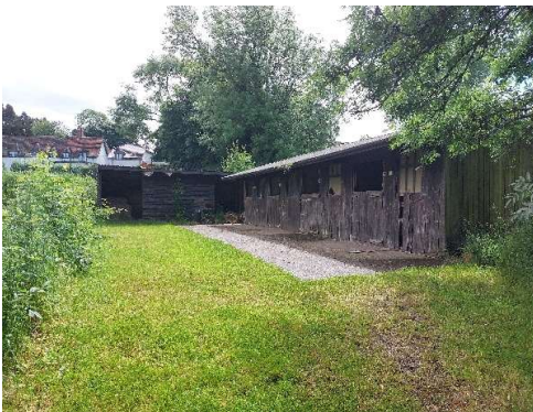
Existing timber 'L' shaped outbuildings to be demolished
