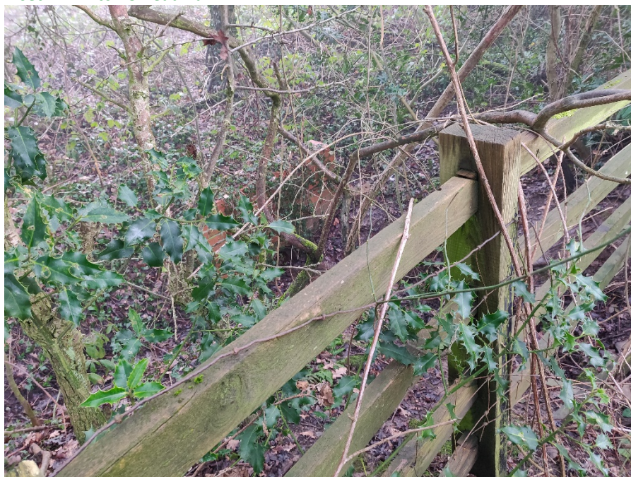
Inset 2.1: Ditch C Headwall
